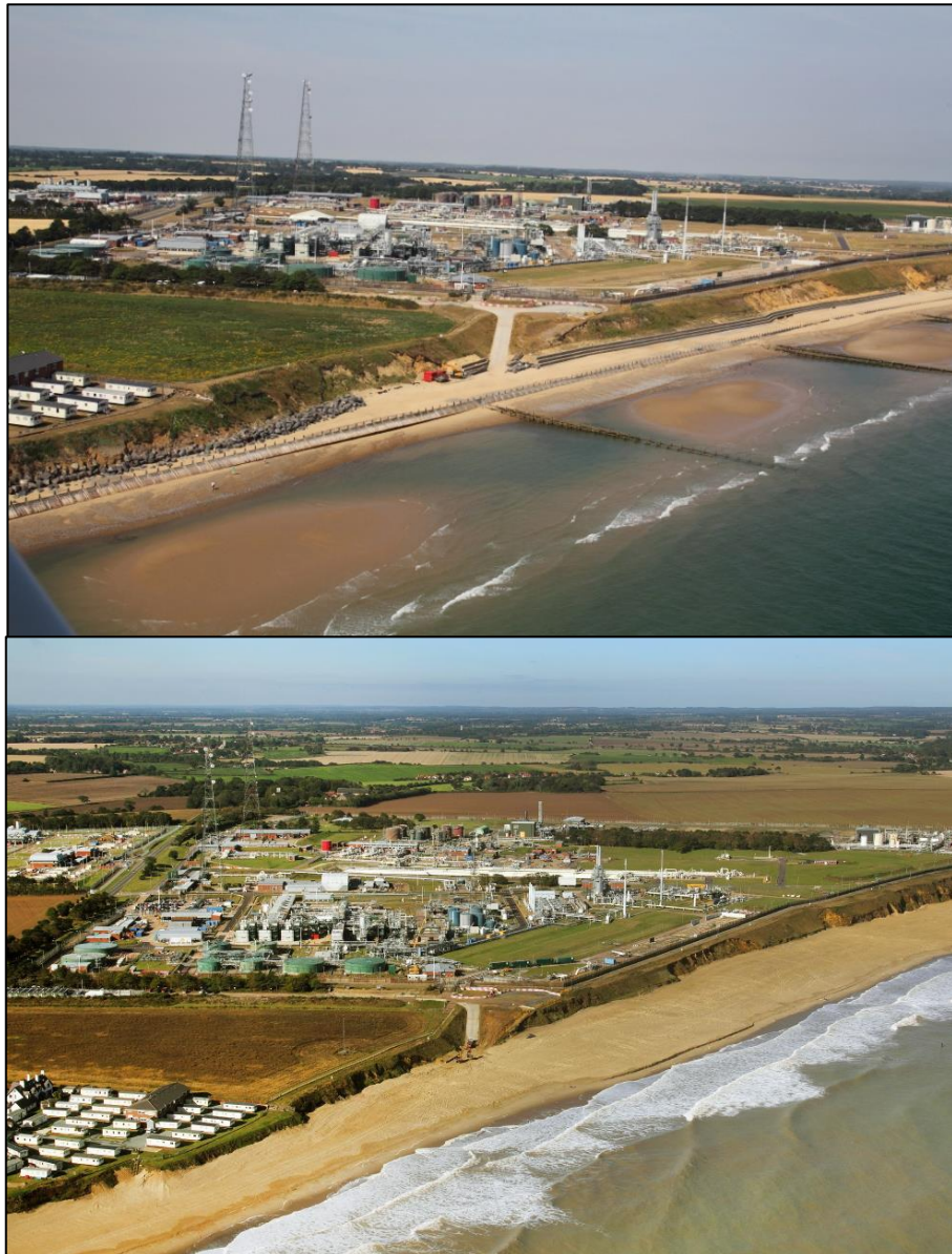
Figure 2.13. Before (top, July 2018) and after (bottom, Sept 2019) photos of Bacton Gas Terminal © Mike Page.
