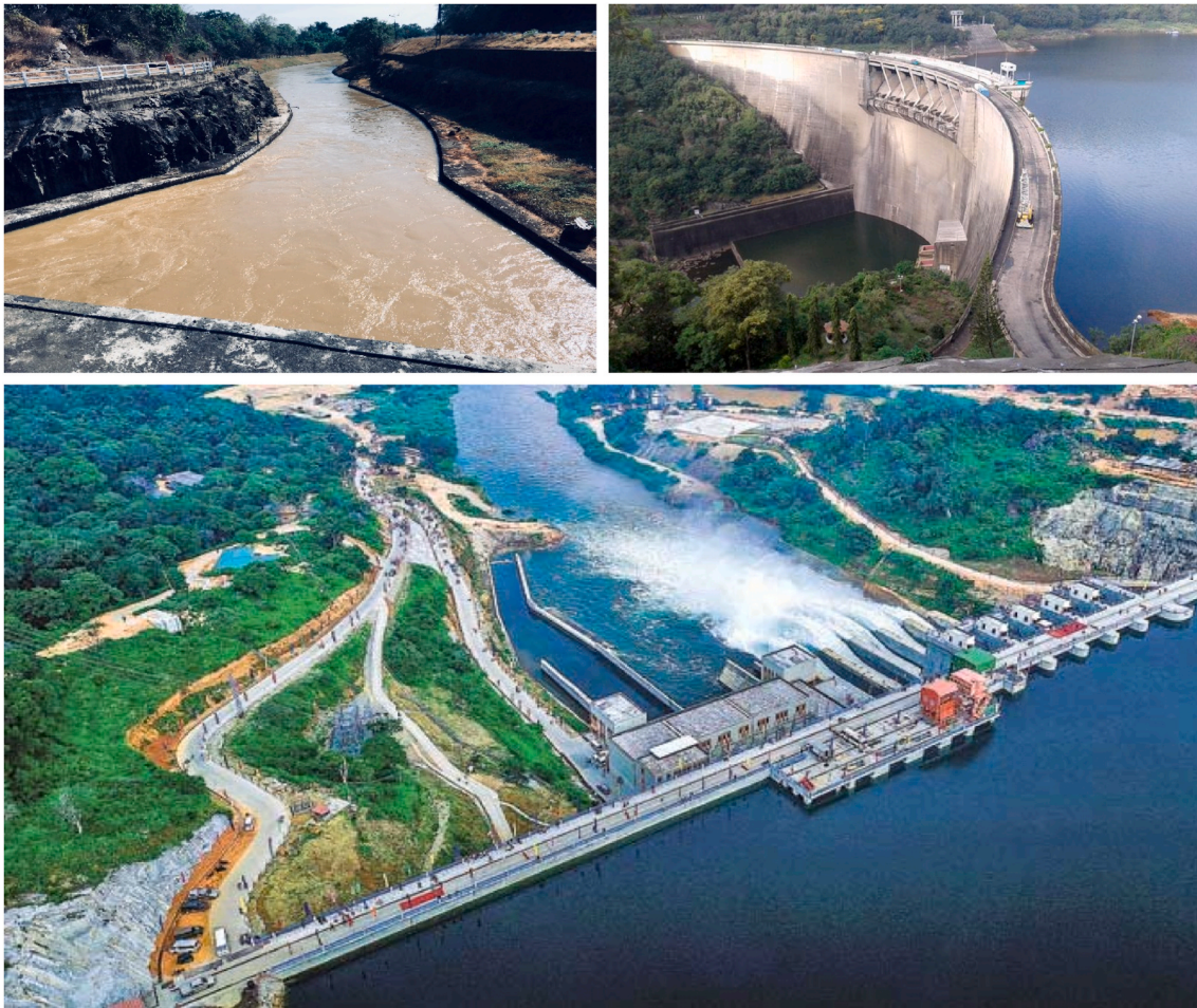
Fig. 2. Examples of the material infrastructure created by the MDP. Top left: A water distribution canal (photographed by the Authors); Top right: The Victoria reservoir. Bottom: The Moragahakanda reservoir – the last major reservoir of the MDP to be completed (Lanka Business Online, 2018).
