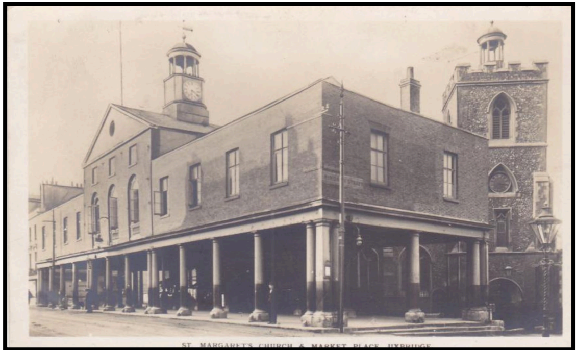
Figure 32: Uxbridge's Market Hall
