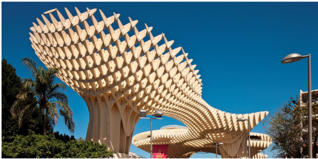
Fig. 3. The Metropol Parasol in Seville, Spain, designed by Jürgen Mayer and completed 2011 features planar mesh parameter lines. The planes carrying parameter are structural elements.
