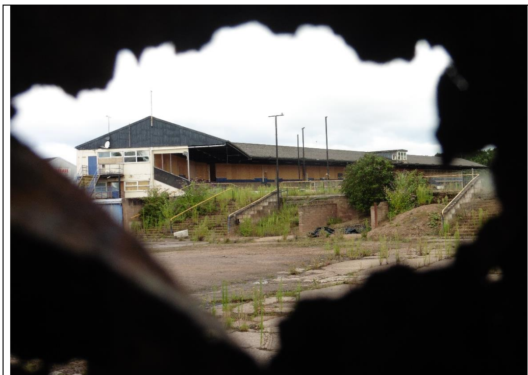
Figure 1: Dereliction at Coventry Stadium, Brandon, Warwickshire. Author, 2019.
