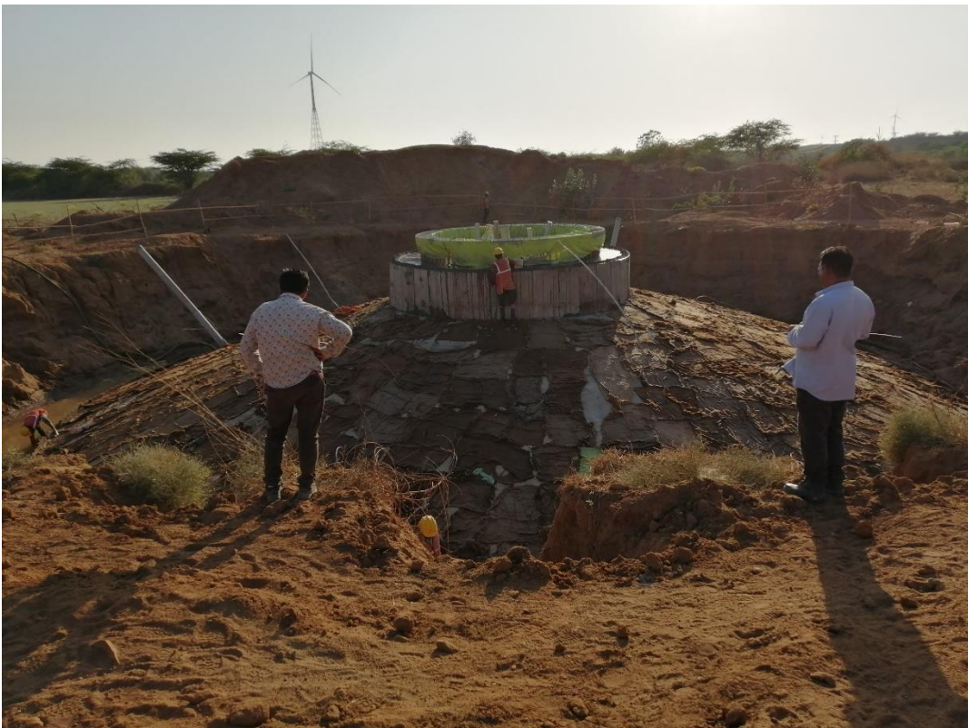
Figure 9 Picture of a 'water location'. The wind turbine point is situated on a groundwater source. The water is drained with the use of a motor pump and released a few meters away from the future wind turbine. (Photo by author)
