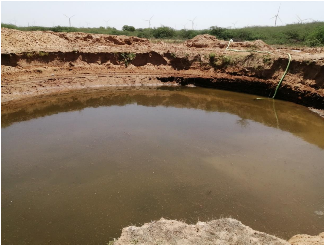
Figure 9 Picture of a 'water location'. The wind turbine point is situated on a groundwater source. The water is drained with the use of a motor pump and released a few meters away from the future wind turbine. (Photo by author)
