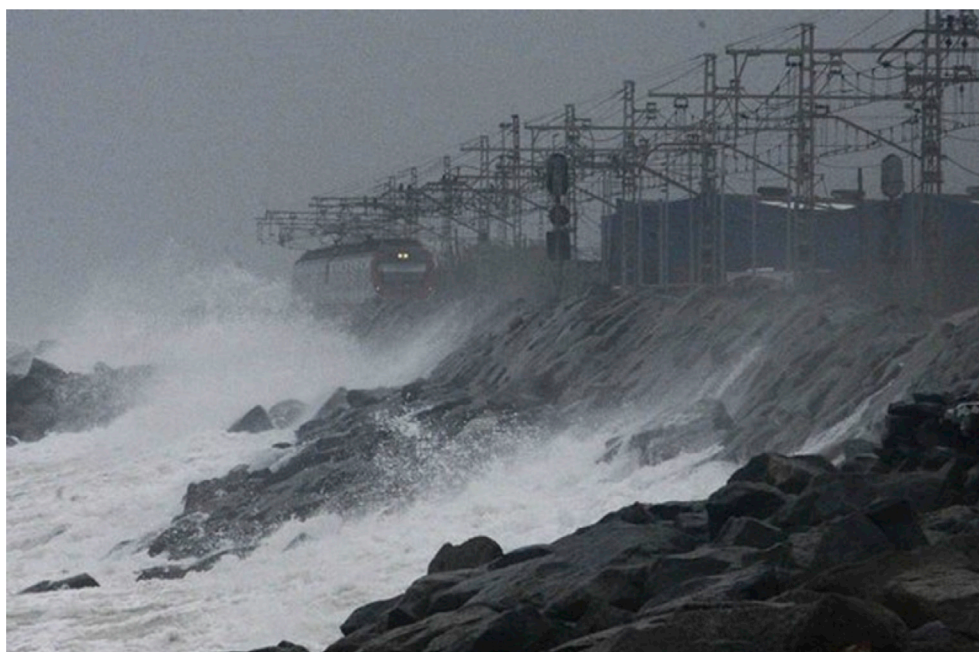
Fig. 5. Affectation of the coastal railway along the Maresme coast during the impact of a storm on March 2003.
