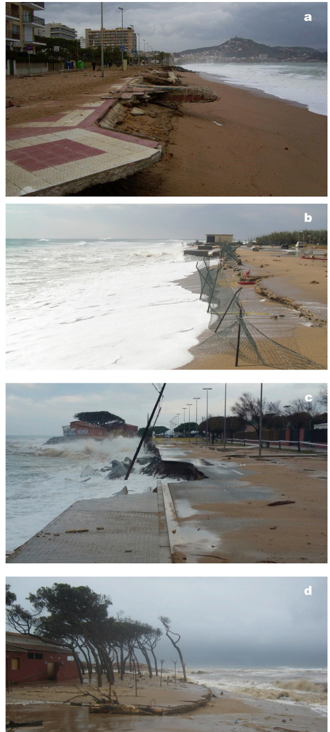
Fig. 10. Example of damages induced in Tordera delta beaches during the impact of different storm events in the last decade (see locations in Fig. 6).
