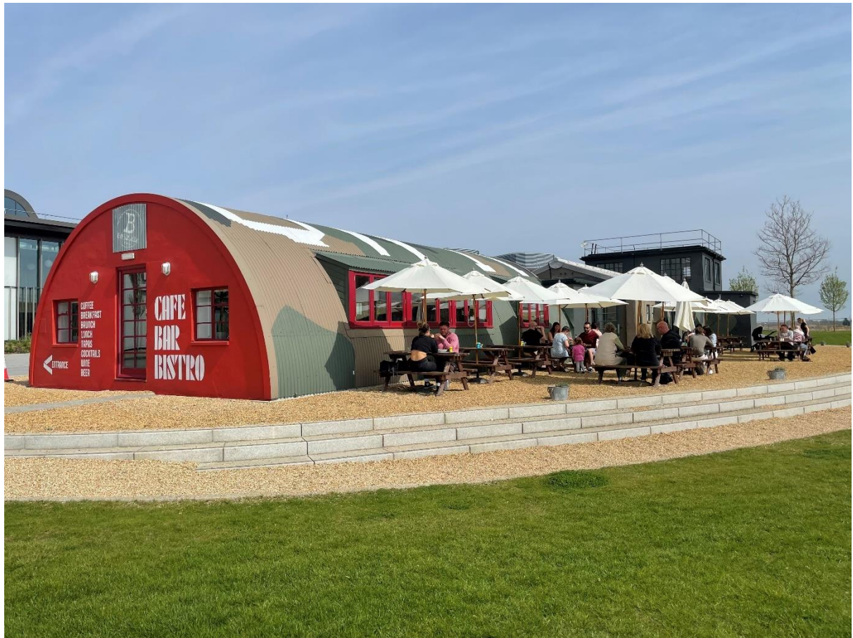
Figure 27 The restored Second World War Watch Tower at Alconbury, April 2022 (Source: Author)
