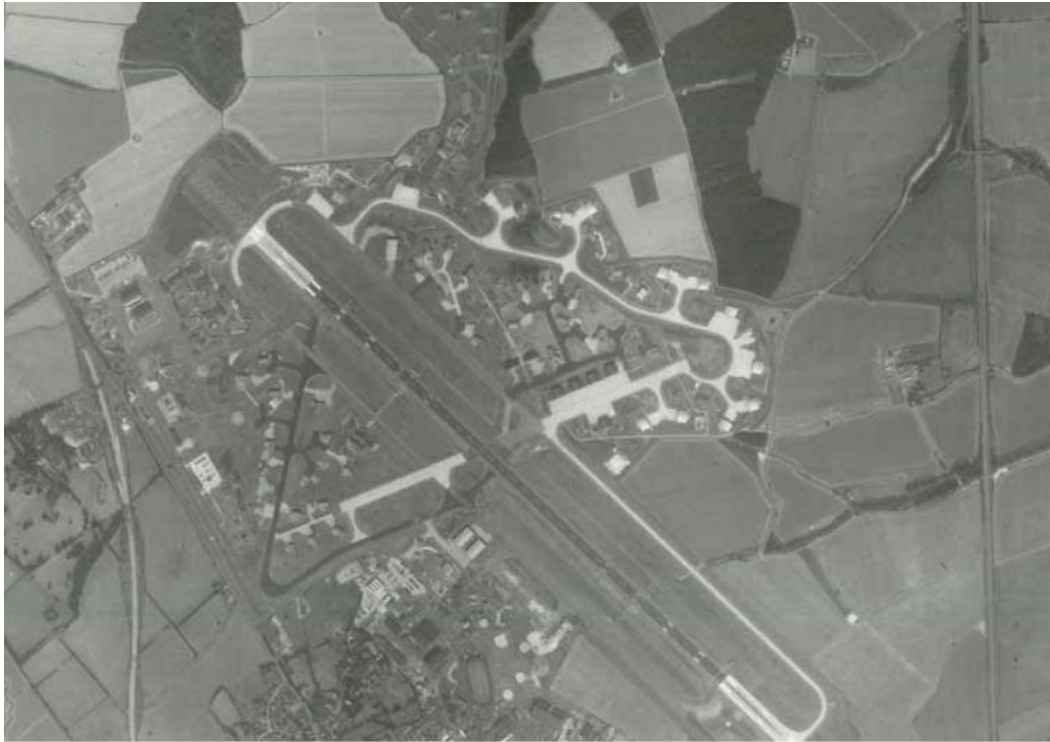
Figure 32 RAF Alconbury in 1991, at the end of an expansive building program which took place between 1977 and 1990 (Source: Urban & Civic)
