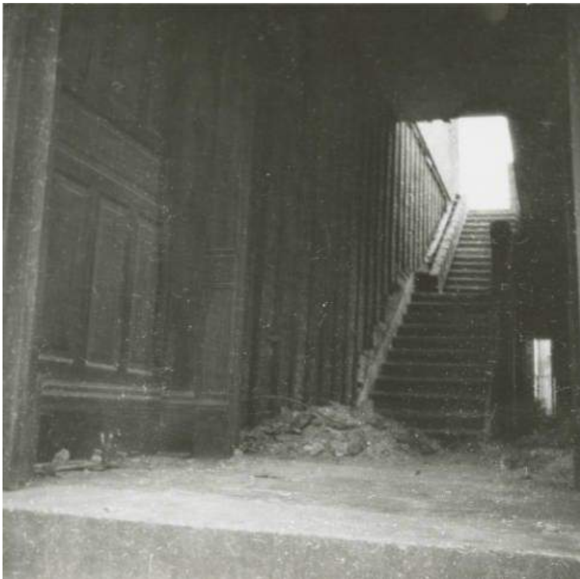
Figure 17 Dan Leyrer, Mahogany Hall before its demolition in 1949
