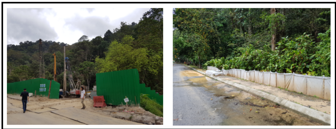
Figure 5.10: Picture taken 500 meter from the entrance of the Ampang Forest Park. This shows the extent of damage caused by the construction, making access to the park difficult.
