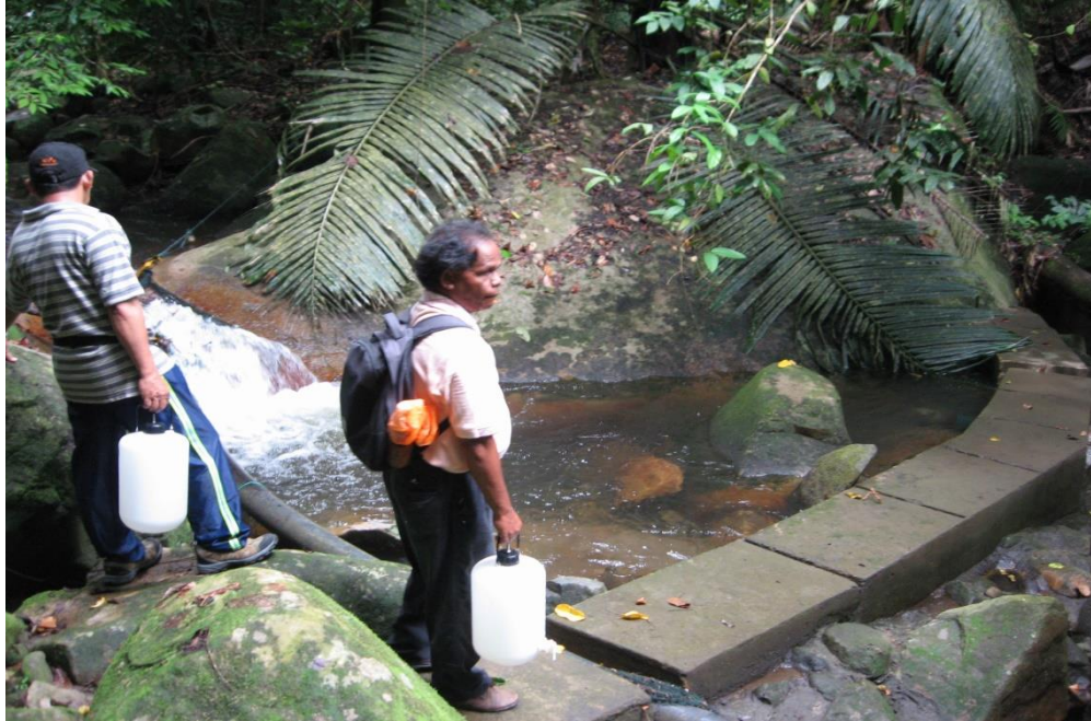
Figure 3-5 Kampung Juara gravity feed dam (drinking water source)
