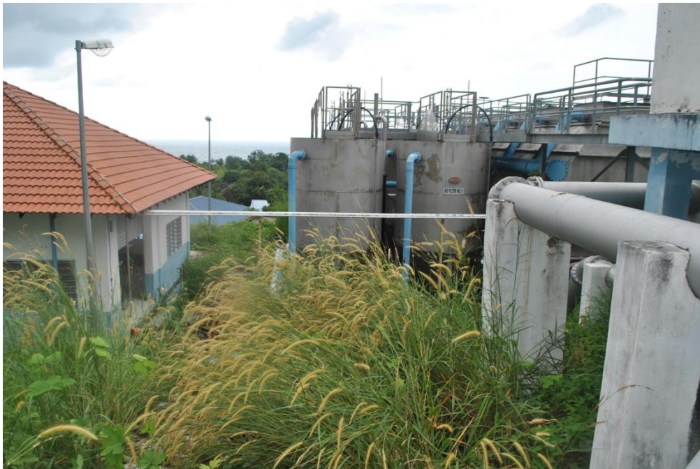
Figure 3-9 Mostly abandoned water treatment plant in Tekek
