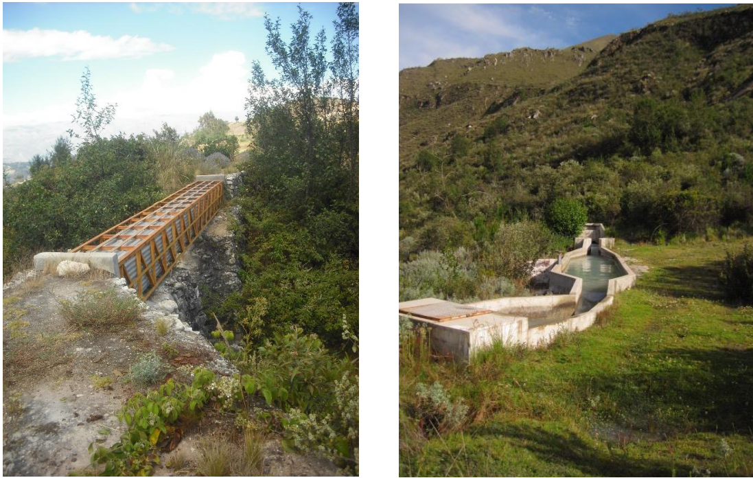
Figure 8.1 Photographs of Yurac Uran Atma lined irrigation canal. Source: own.
