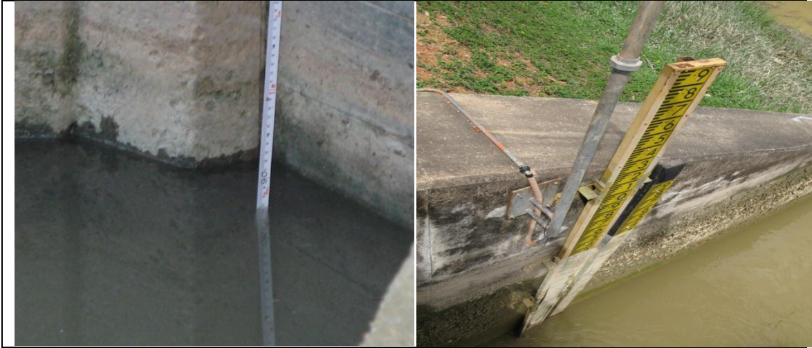
Figure 4-15: Measurement tape used to determine the water level upstream of the gate (left panel) and existing gauge board at the downstream of the gate (right panel).
