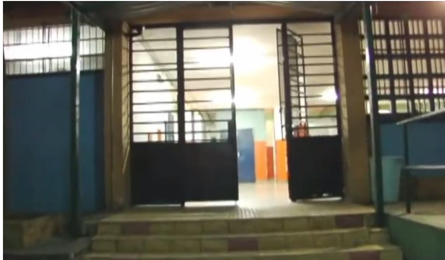
29. Second padlocked entrance gate.
