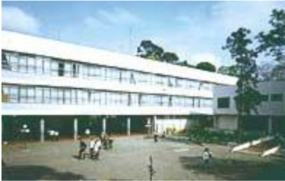
22. School building in São Paulo, 1961. 53
