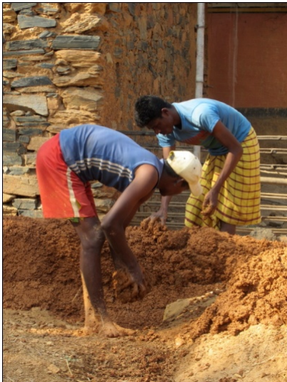
Figure 4-8: Smoothing of murrum mati to create flat surfaces
