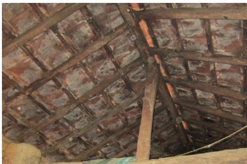
Figure 4-31: Battens spaces further apart for tali (rectangular clay tiles)
