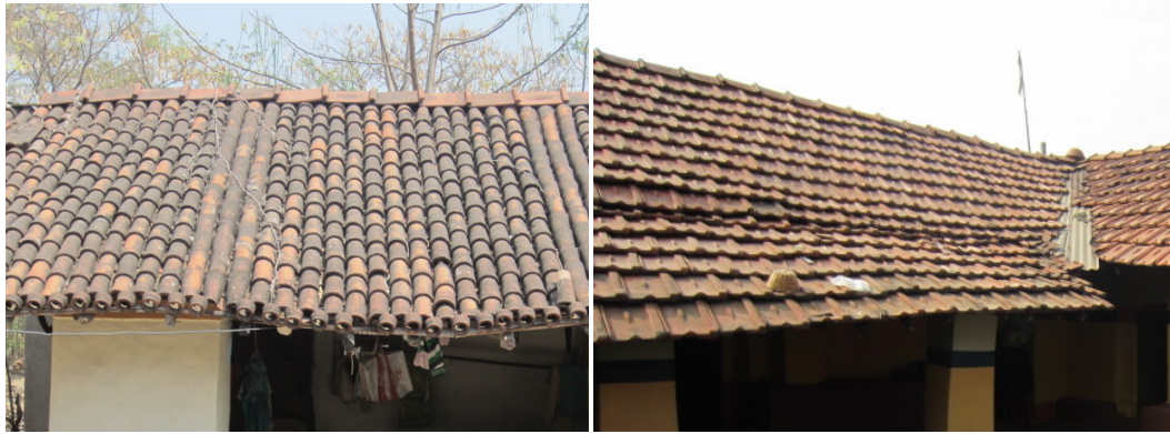
Figure 4-35: Types of clay tiles used for roofing: khapra on the left and tali on the right
