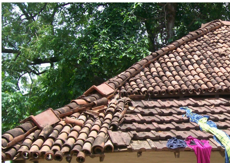
Figure 4-44: Two layers of tiles used to cover the hip junction in an L-shaped roof
