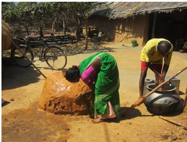
Figure 4-39: After kneading, the pile is smoothened out and left to rest. This processes of kneading and resting is repeated three times before the murrum mati is ready for use.
