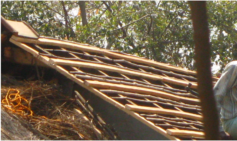
Figure 4-17: Rafter with rectangular cross section
