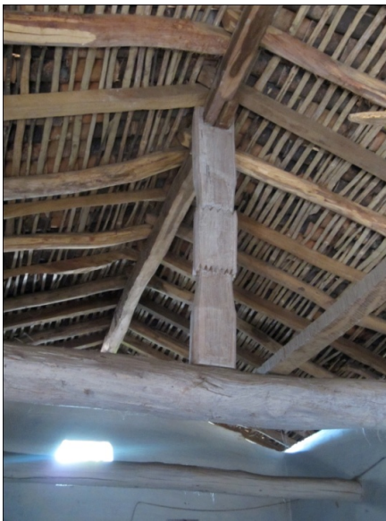
Figure 4-11: Post notched into central beam
