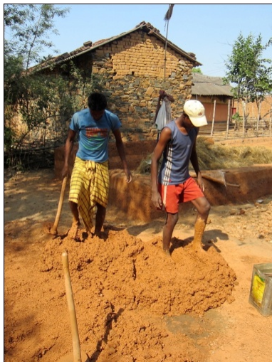
Figure 4-5: Kneading of murrum mati to soften and prepare it for use
