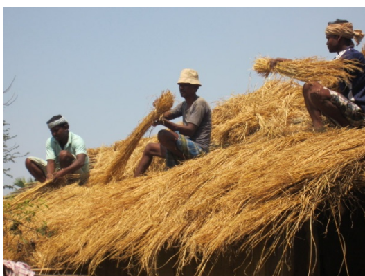
Figure 4-33: Men laying thatch on a roof
