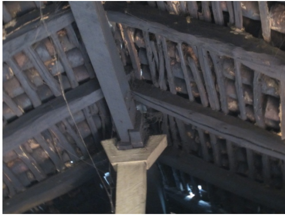
Figure 4-14: Joint between post and ridge beam made using additional wooden member
