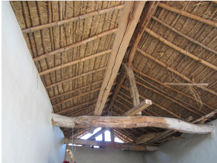
Figure 4-48: Bamboo used in roofing. Note both rafters and battens are made of bamboo.
