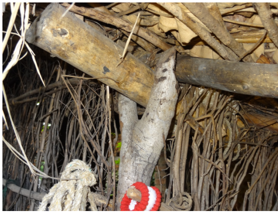
Figure 4-46: Forked end of post used to support beam in Birhor house
