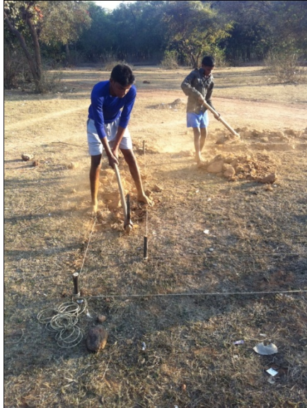
Figure 4-1: Digging the area marked within ropes on ground
