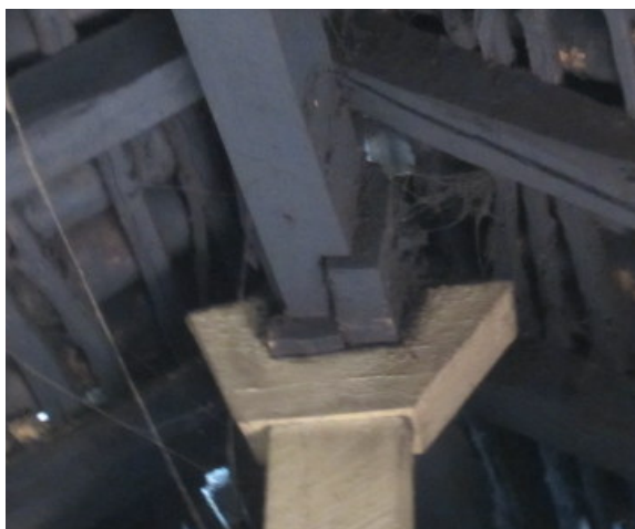
Figure 4-15: Lap joint in ridge beam held between and propped by the post
