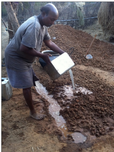
Figure 4-37: Pit filled with murrum mati and filled with water. The murrum mati absorbs the water and softens before being used.
