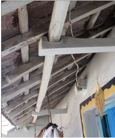
Figure 4-21: Eaves beam supported on additional wooden supports projecting from wall
