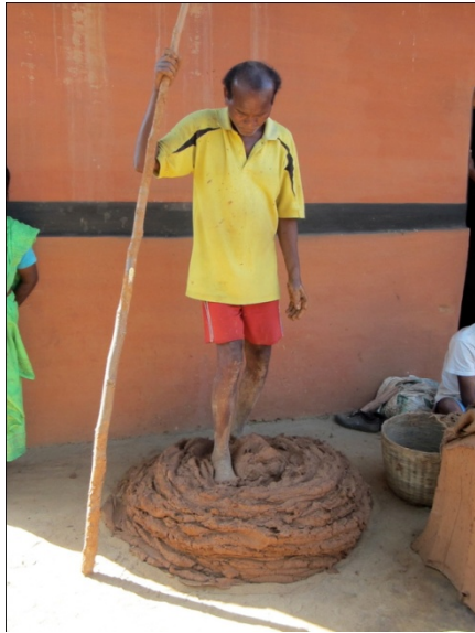
Figure 4-38: The soaked murrum mati is piled outside the pit and kneaded by repeatedly stepping on it.
