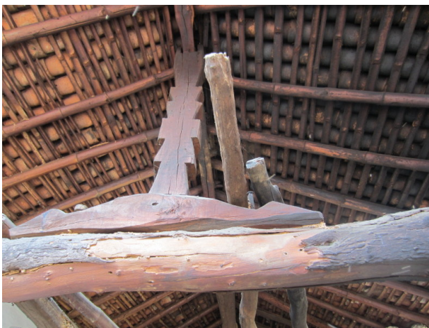
Figure 4-12: Additional wooden member used for creating joint between post and beam
