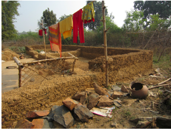
Figure 4-9: Wall left to dry before addition of further courses
