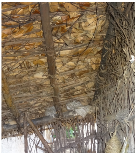
Figure 4-47: Rafters, battens (made of thin branches) and thatch visible in the ceiling of Birhor house
