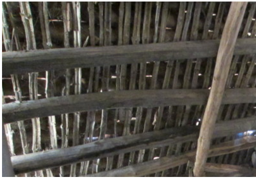
Figure 4-30: Closely spaced battens for khapra (burnt clay tile) roofing
