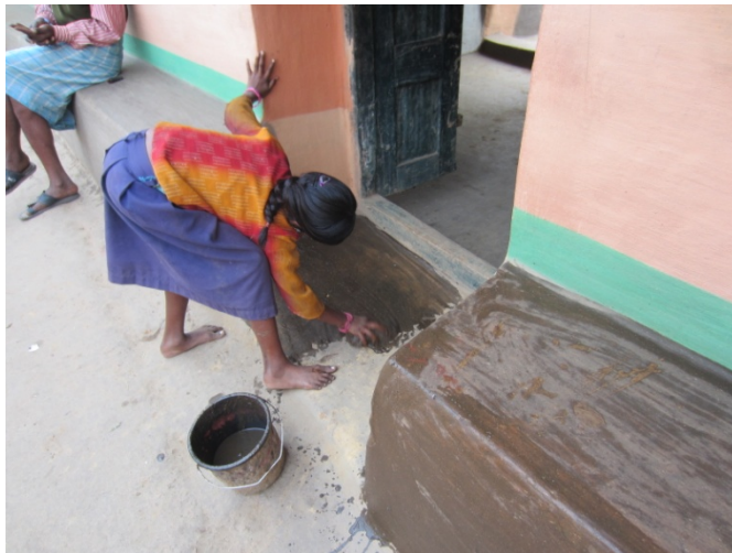
Figure 5-6: Plastering the entrance to the house with a piece of cloth dipped in a cow dung mixture
