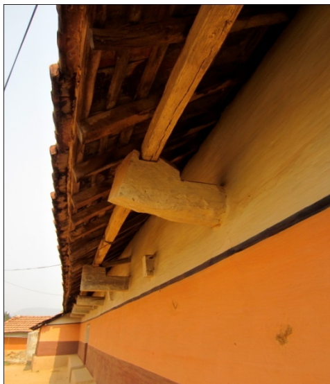
Figure 4-20: Eaves beam supported on extension of central beam
