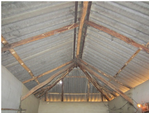
Figure 4-32: Very few battens required for roofing done using sheets
