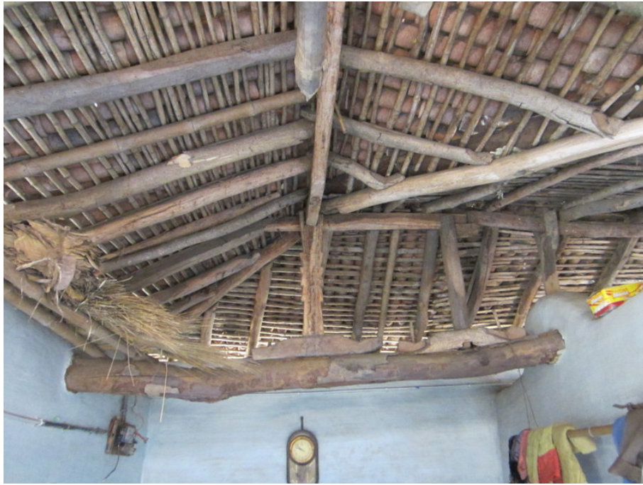
Figure 4-27: View of L-shaped junction in the roof of courtyard houses
