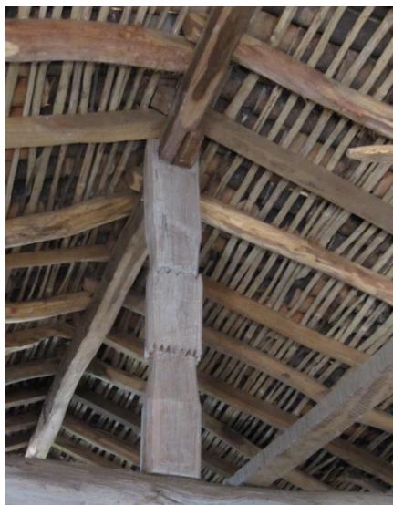
Figure 4-13: Post carved to accommodate ridge beam
