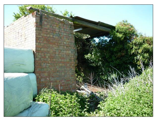
Figure 14: Photograph taken looking north-west towards the entrance to Room 7 of the Generator Building. The 'English' bond brickwork is clearly visible. At a later date, the southern section of the eastern elevation was partially demolished. There is no evidence that the room was originally roofed (Gregory 2013).
