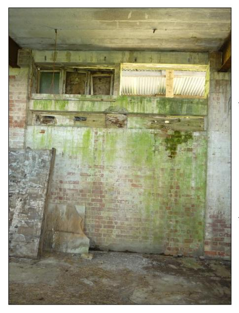
Figure 22: Photograph of one of the panels which form the elevations of Room 4 and 5. Numerous wooden window frames survive in situ. At the base of a number of the window frames are pulleys which are associated with pulleys on the ceiling. The pulleys enabled the windows to be opened from the floor level with the rope being tied off on one of the brackets attached to the buttresses (*Gregory 2013*).
