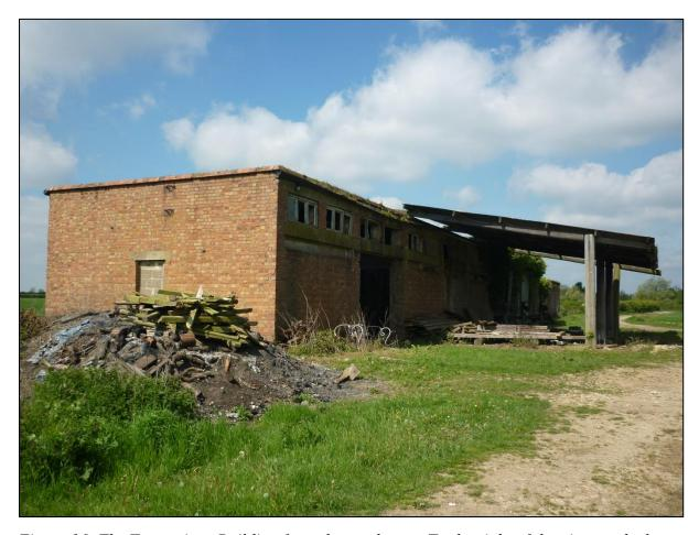
Figure 16: The Transmitter Building from the north-east. To the right of the picture, the later addition of a lean-to is clearly visible. It is believed that the wooden posts once formed the antennae of SOE's Station 53B transmitter complex. The blocked up doorway into Room5 is visible on the eastern elevation of the building (Gregory 2013).
