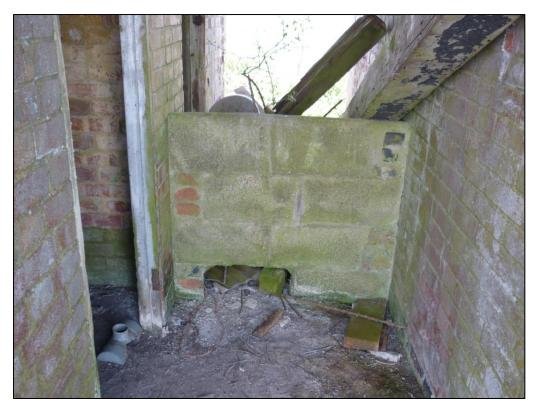
Figure 28: Photograph of the breeze block half-wall in Room 1 of the Generator Building (Gregory 2013).
