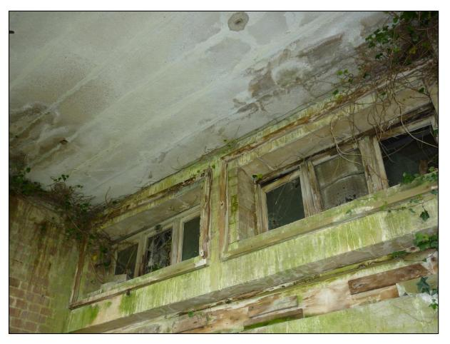
Figure 23: Photograph of in situ window frames in Room 4 of the Transmitter Building. Wire-meshed glass panes are visible within the windows. The method of opening the windows via a series of pulleys can be observed in this photograph (Gregory 2013).
