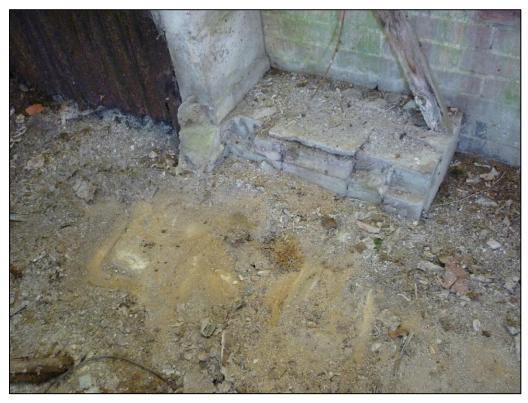
Figure 31: Brick footing attached to the western section of the northern elevation in Room 4 of the Generator Building (Gregory 2013).
