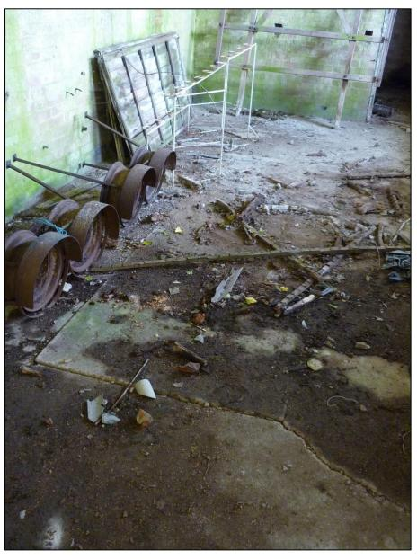
Figure 9: Photograph taken looking south-west within Room 5 of the Generator Building. The scar associated with the generator is clearly visible on the concrete floor (Gregory 2013).
