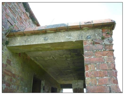
Figure 27: Supporting beam across the northern entrance to Room 1 of the Generator Building (Gregory 2013).
