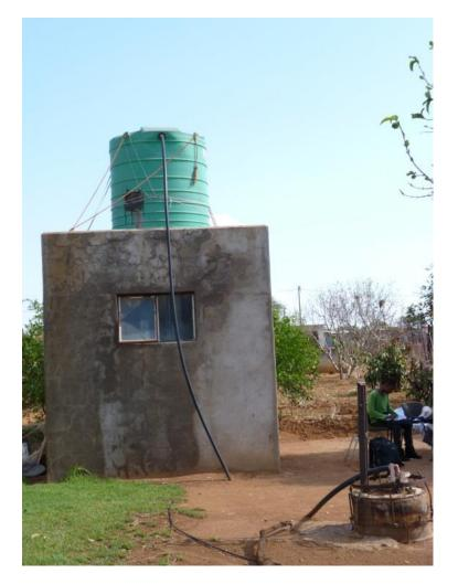
Figure 2.3: Drilled well and storage tank in Community 2 *Source:* Author
