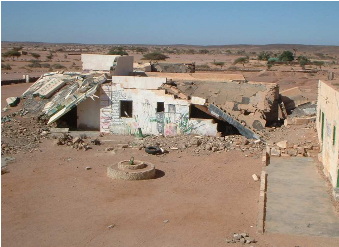
Fig. 6.21: East facing elevation along the west side of the central courtyard of the fort at Tifariti, photographed in 2011. This view almost matches that in Fig. 6.22. The graffiti-like painting on the building remains was applied during one of the ARTifariti festivals held in Tifariti (2007-2010). See Chapter 7.
