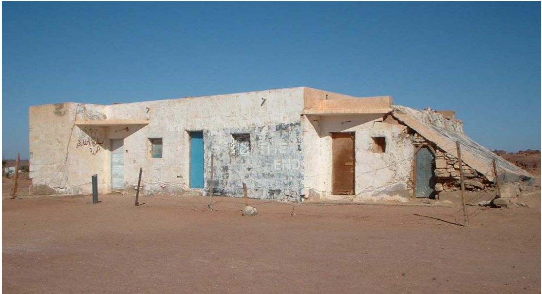
Fig. 6.29: View of the Spanish period infirmary in Tifariti (2011), looking northwest. The graffiti-like painting on the building was applied during one of the ARTifariti festivals held in Tifariti (2007-2010). See Chapter 7.
