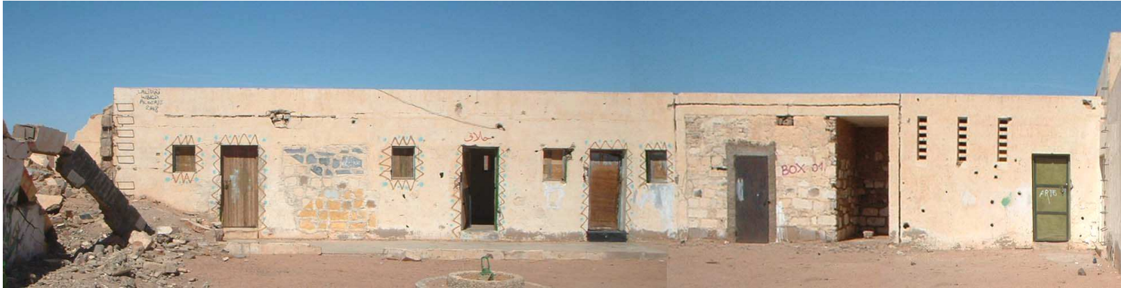
Fig. 6.19: South facing elevation along the north side of the central courtyard of the fort at Tifariti. Composite photograph taken in 2011.
