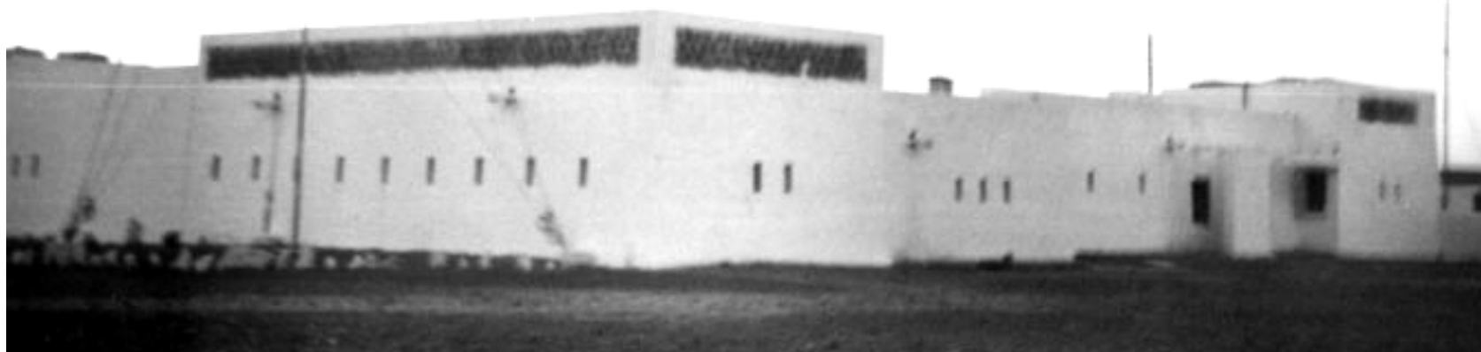
Fig. 6.18: November 1974 view of the rear wall of the fort at Echdeiria, showing what the rear, northern wall of the fort at Tifariti would have looked like before it was damaged in 1991. Image source: photograph taken by Adolfo Peña Herrero, available at: http://www.sahara-mili.net/person/albumPersonalMarcos.htm accessed 9 March 2013.
