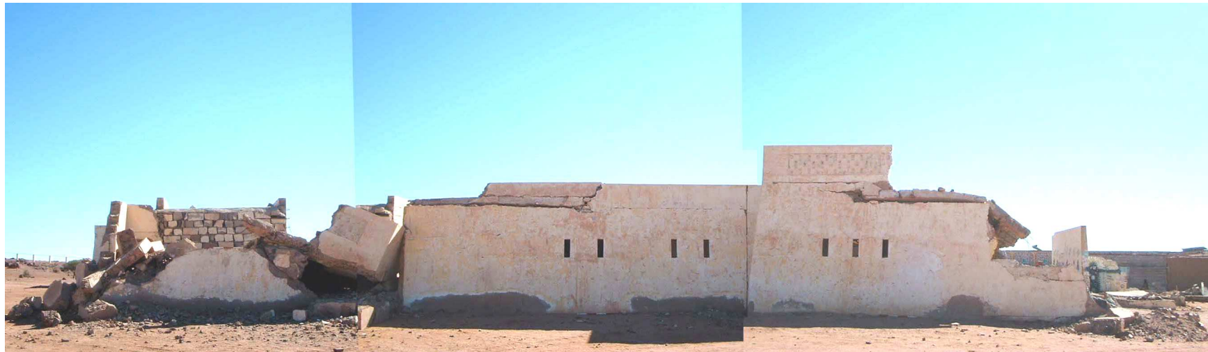
Fig. 6.15: Composite image of the west facing elevation of the fort at Tifariti (recorded in 2011), showing the damage sustained in the Moroccan air strikes of 1991. To see what this elevation must have looked like in an undamaged state, see Fig. 6.16, an image of the contemporary fort at Echdeiria.
