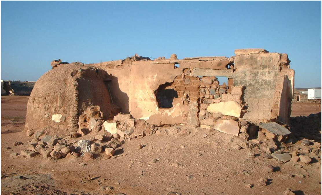
Fig. 6.31: View (looking west) of the bake house behind the fort at Tifariti. The oven is to the left. A doorway has been blocked, and the impressions of wall tiles can be seen on the internal wall, visible to the right.
