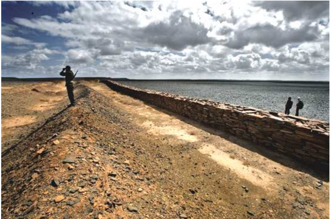
Figure 4.41: A view of the Moroccan barrier at ground level, photographed near Tifariti. The barrier has three elements: the stone wall at the rear, an earthen bank in the centre, followed by a frontal embankment with two ridges, just visible at the left of the photograph. The Saharawi soldier on the barrier gives a sense of scale. Image source: © Bruno Zanzottera, from http://stock.parallelozero.com and http://www.parallelozero.com/images/stock/mid/c72e465d7af3494aa14600a8956d98bb5fa097fc.jpg accessed 12 April 2014.
