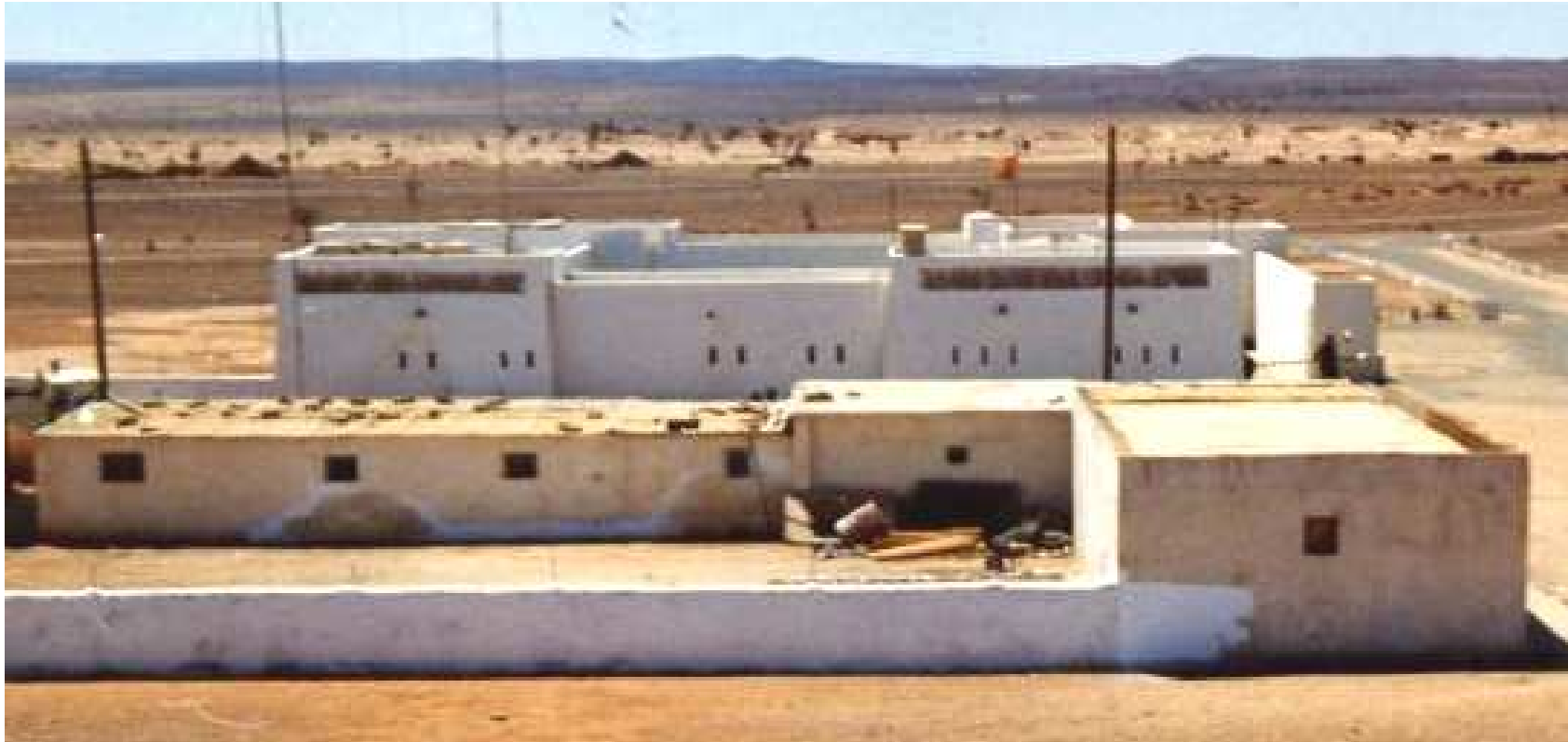
Fig. 6.16: The fort at Echdeiria. As at Hausa, this fort was identical to the one at Tifariti, and this view shows the matching elevation to that shown in Fig. 6.15, before it was substantially damaged in the air attacks of 1991. The blockhouses at either end are clearly shown, as is the entrance to the right, where there is also a bar across it, as is similarly visible in Fig. 6.10. Image source: photograph taken in July 1974 by Adolfo Peña Herrero, available at: http://www.sahara-mili.net/person/albumPersonalMarcos.htm accessed 9 March 2013.
