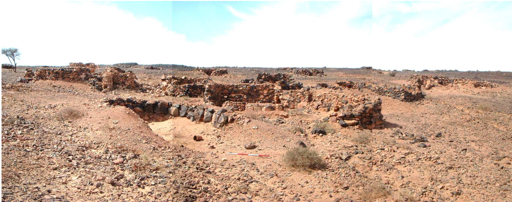
Fig. 6.78: Composite panorama of buidings in the Tifariti 'redoubt'. Just left of the metre scale is a vehicular slot; behind it, to the right and left, are the remains of shelters/accommodation for Moroccan soldiers. These features are protected behind the ridge (to the northwest) in the rear of the image.
