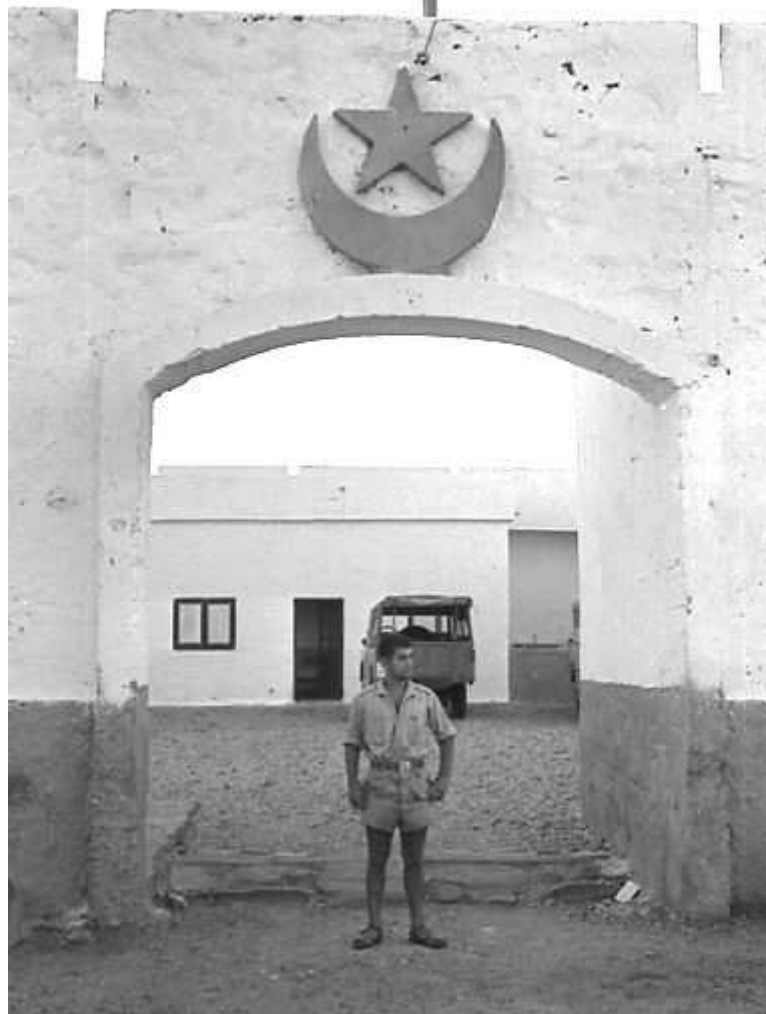
Fig. 6.23: View of the gateway into the 1940s fort at Tichla. Its construction is apparently of stone with a rough render. This is in contrast to the smooth, cast concrete construction of the fort at Tifariti. Image source: photograph taken in 1971 by Juan Piqueras, available at: http://www.sahara-mili.net/lugar/albumLugarMarcos.htm accessed 9 March 2013.
