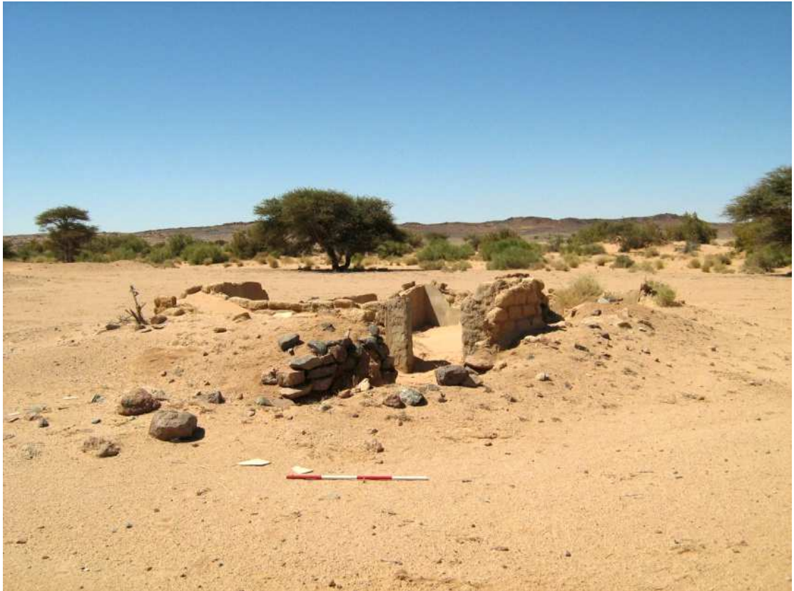
Fig. 6.54: Moroccan Army field structure in the Wadi Tifariti at the TF1 study area. It is built mainly of mud bricks with, in this example, an internal cement render. The structure is surrounded by embanked earth, with an entry passage revetted with stones.
