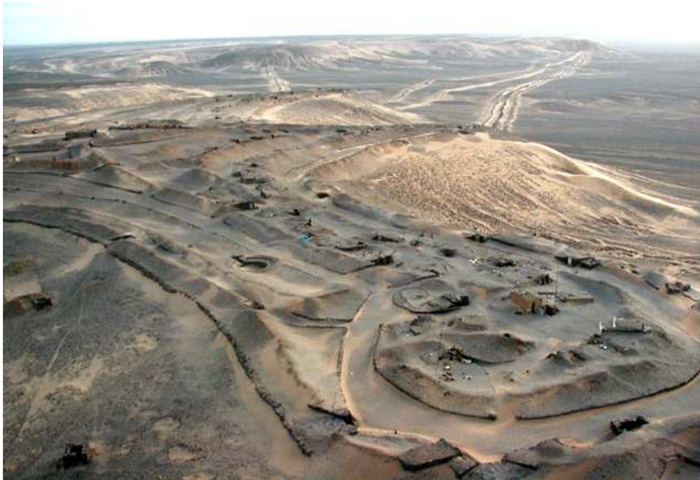
Fig. 4.52: Low level aerial view of fort ft 681 in Fig. 4.51. The view is to the east, so north is to the left. This image clearly illustrates the disposition of this sizable fort on high ground, overlooking Polisario controlled territory to the right (the south). Image source: unattributed image from http://www.lasonet.com/sahara/sh-163.htm accessed 15 January 2014.
