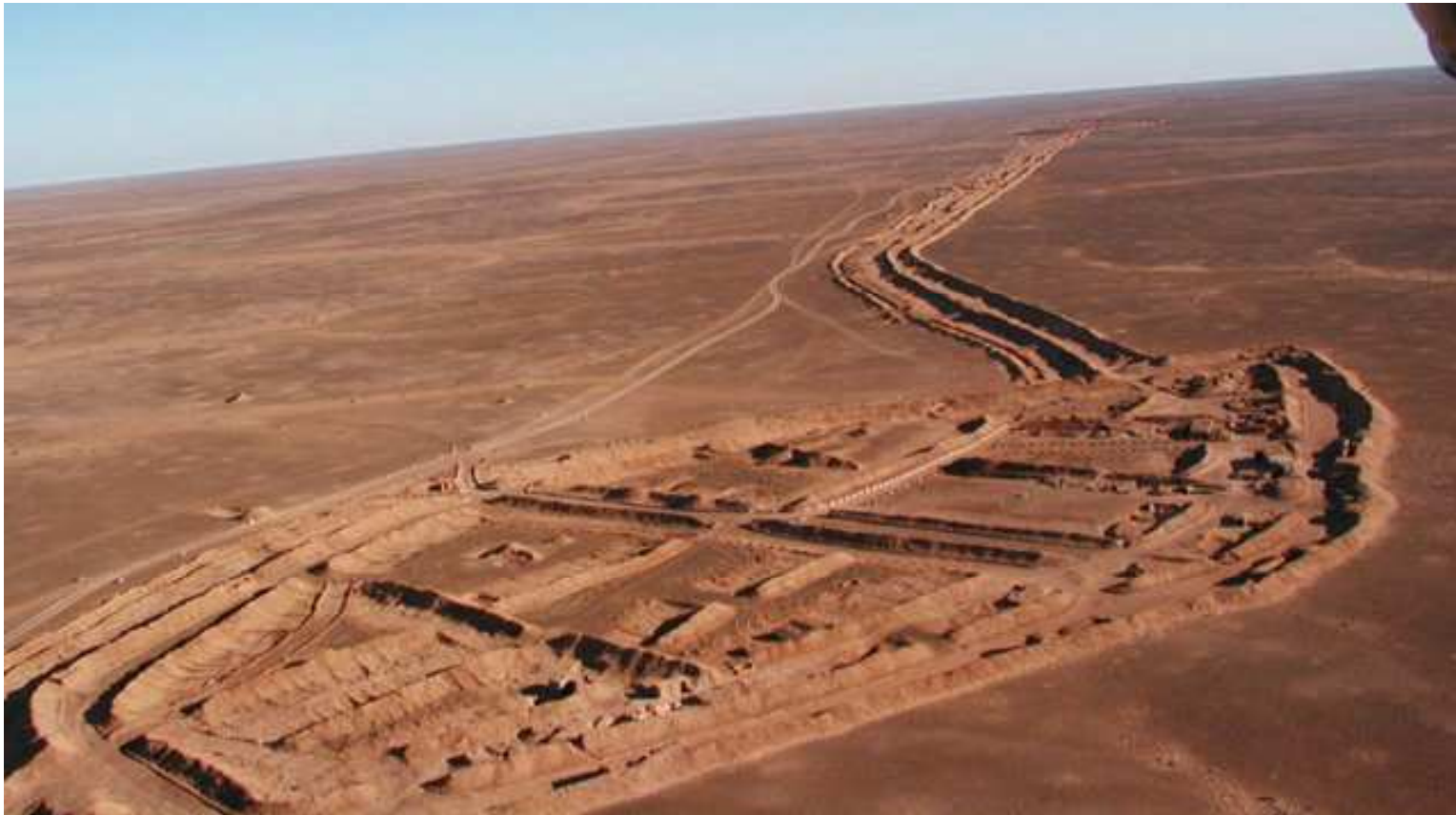
Fig. 4.59: This is a very good example of a concentrically embanked fort on one of the Moroccan berms, illustrating the complexity of internal compartmentalization with sand embanked blast barriers. Image source: unattributed image from http://www.lasonet.com/sahara/sh-163.htm accessed 15 January 2014.
