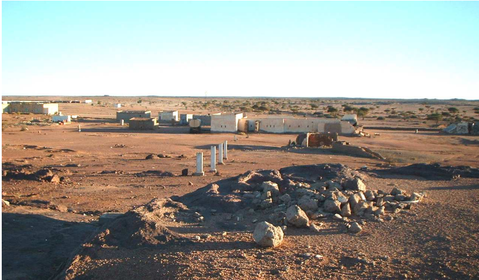
Fig. 6.32: View, to the south, showing the concrete posts that supported the gravity fed pipe that provided water to the Tifariti Fort. The Bake House is also visible in front of the fort. Its northwest, channelled extension (possibly a flue) is visible with ashy ground adjacent.
