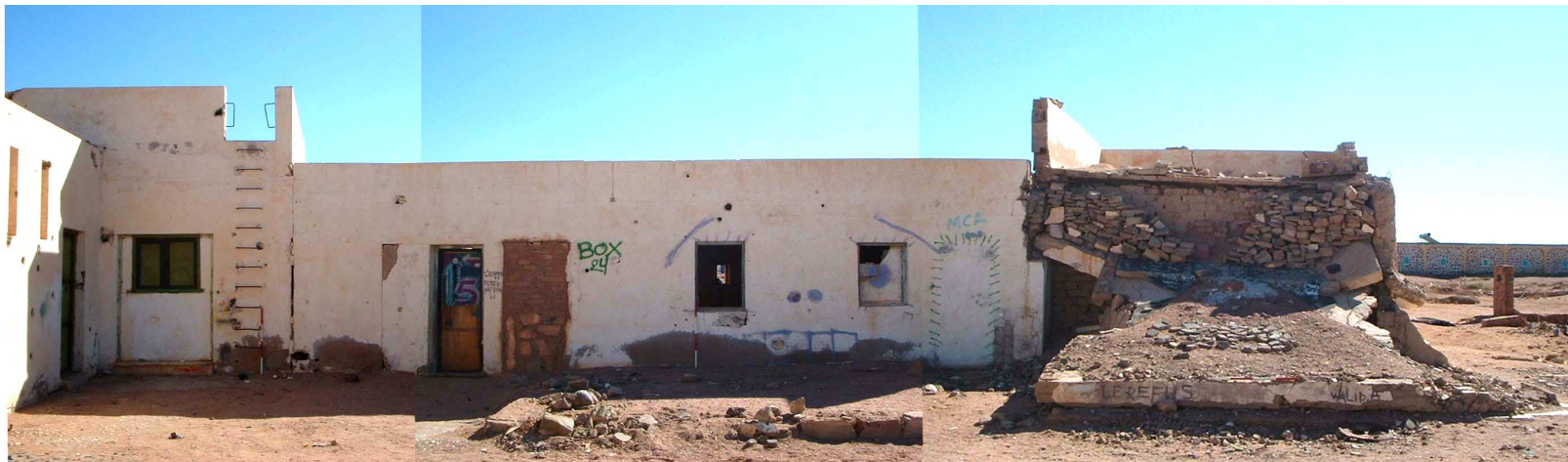
Fig. 6.20: West facing elevation along the east side of the central courtyard of the fort at Tifariti. Composite photograph taken in 2011. The graffiti-like painting on both elevations was applied during one of the ARTifariti festivals held in Tifariti (2007-2010). See Chapter 7.
