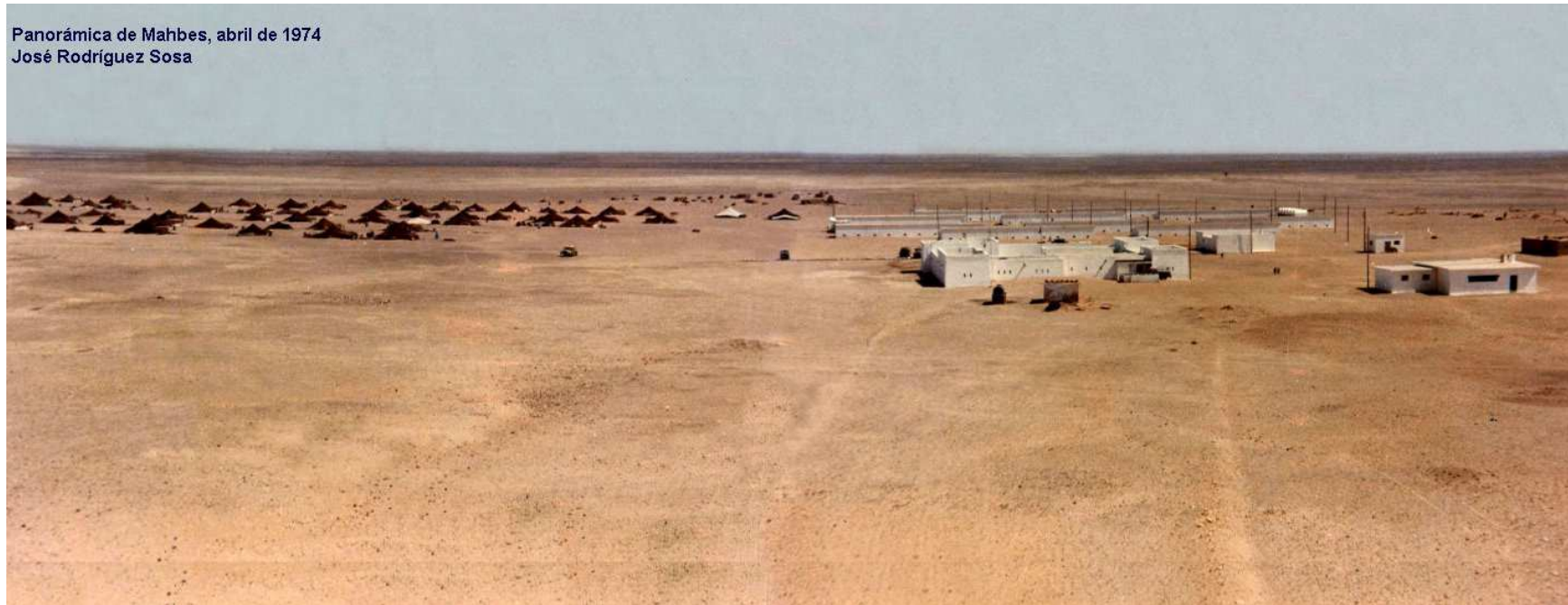
Fig. 6.40: A panorama of Mahbes, showing a large Bedouin encampment in the left half of the photograph; an identical fort to the one at Tifariti off centre to the right; ancillary post buildings beyond the fort; and an infirmary type building at the right hand edge of the photo, similar to the infirmary at Hausa. This image clearly shows the relationship between the different elements, Saharawi and Spanish, making up a Spanish period desert settlement. Image source: photograph taken by José Rodríguez Sosa in 1974, available at http://www.sahara-mili.net/images/jrdgzs/jrs001.jpg accessed 17 March 2013.
