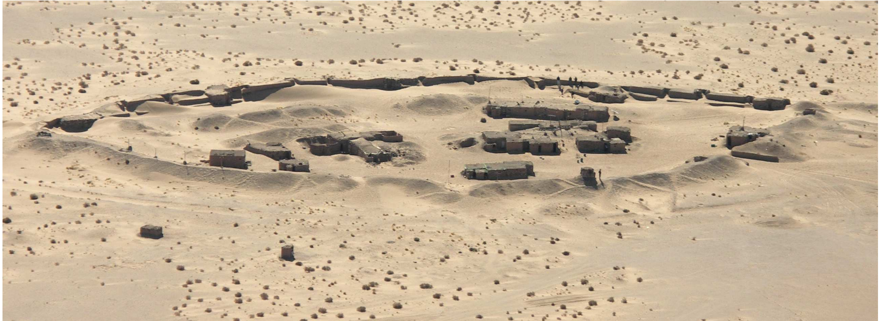
Fig. 4.60: View of a mural fort along one of the Moroccan berms. The image shows the construction of internal buildings quite well, and a parapet walkway with niches: fighting and observation positions. Image source: attributed to ‘MINURSO Database’ and available at http://www.tindoufexpress.org/tep/?page_id=183&lang=en and http://www.tindoufexpress.org/tep/wp-content/uploads/2013/05/Muro_ONU_2007.06.07_-1_028.jpg accessed 17 January 2014.
