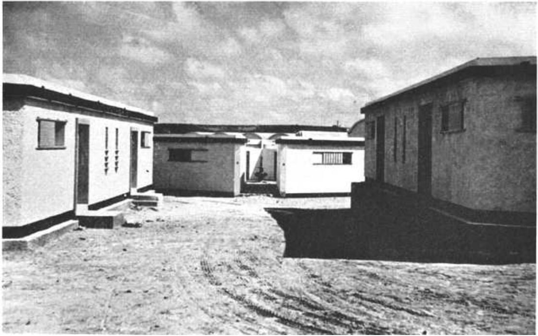
Fig. 6.37: View of low cost housing in El Ayoun in the 1960s. These are examples of what the pre-fabricated housing in the colonia at Tifariti might have looked like. Image source: Norris 1964.
