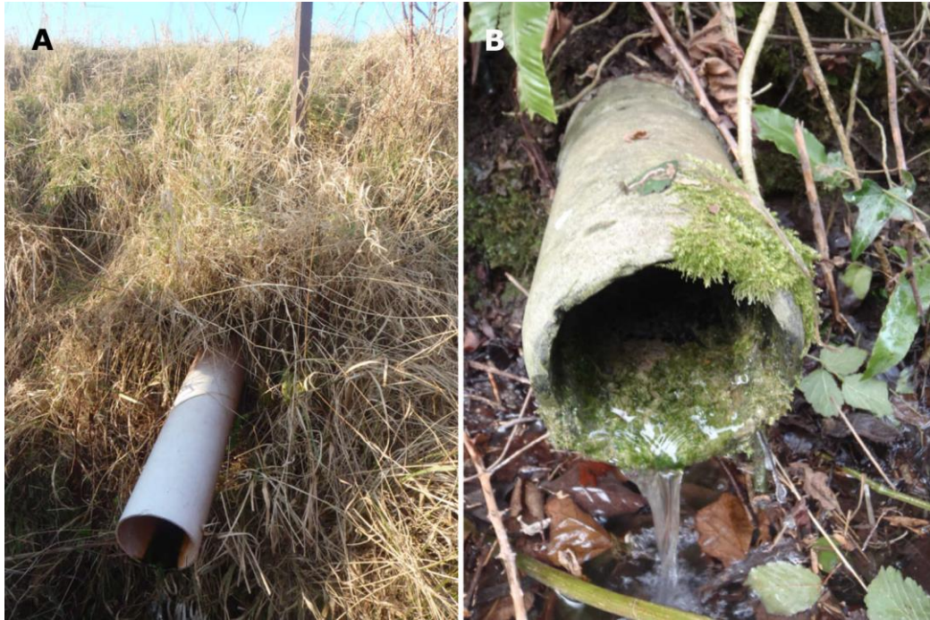
Figure 5.5: Plastic (A), concrete (B) and clay agricultural field drains underlie most of mini-catchments A and B. The majority are situated 1-1.5 m below the surface and discharge directly into the stream. Diameter of both drains shown is ~10 cm.
