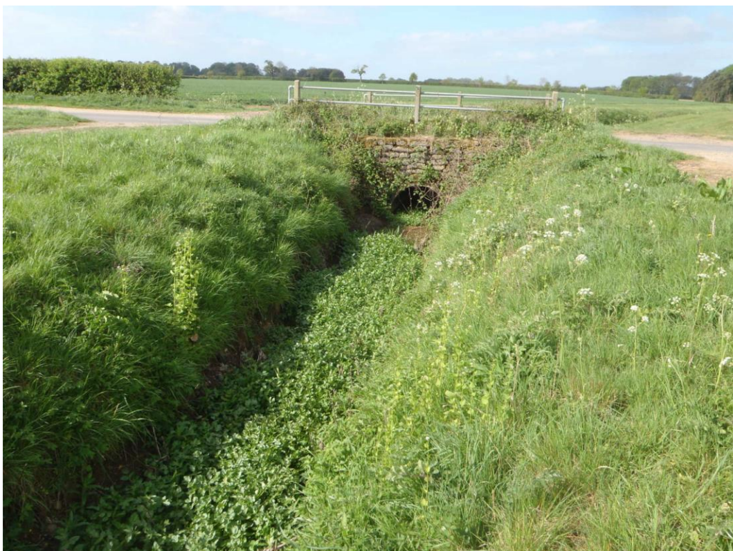
Figure A3: The River Blackwater at the road bridge in mini-catchments A. May 2011. This road crossing is an important location for sediment ingress into the stream channel
