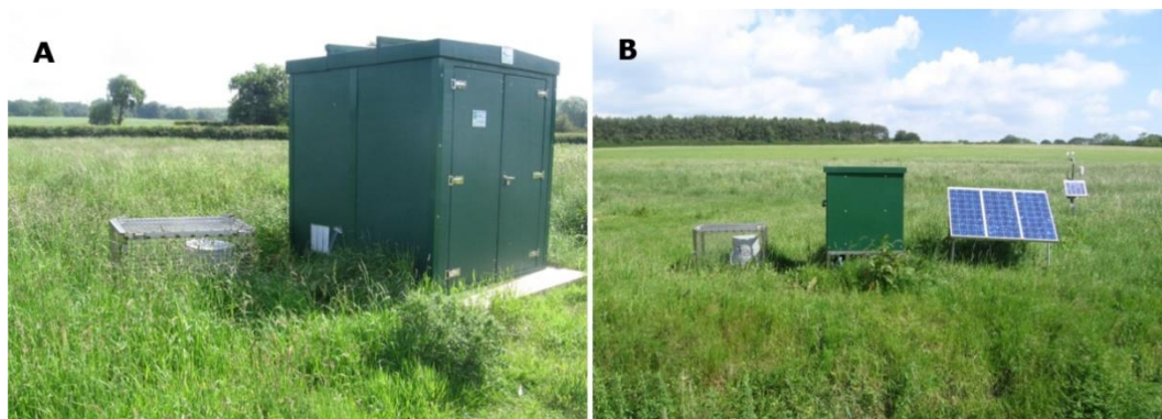
Figure 2.2: Images of the Blackwater sub-catchment showing the main and ‘mini’ bankside monitoring kiosks located at Stinton Hall Farm E (A) and Swanhills A (B), respectively. ISCO automatic samplers are visible in the metal cages to the left hand side of both kiosks. The weather station can be seen in the right hand side of image B. Further images of the Blackwater can be found in Appendix A.
