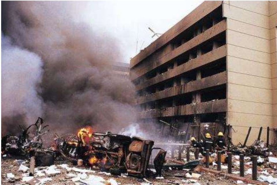
Fig.2.1: The bombed U.S. embassy building, Nairobi, 1998. (Photo: Jacob Otieno).
