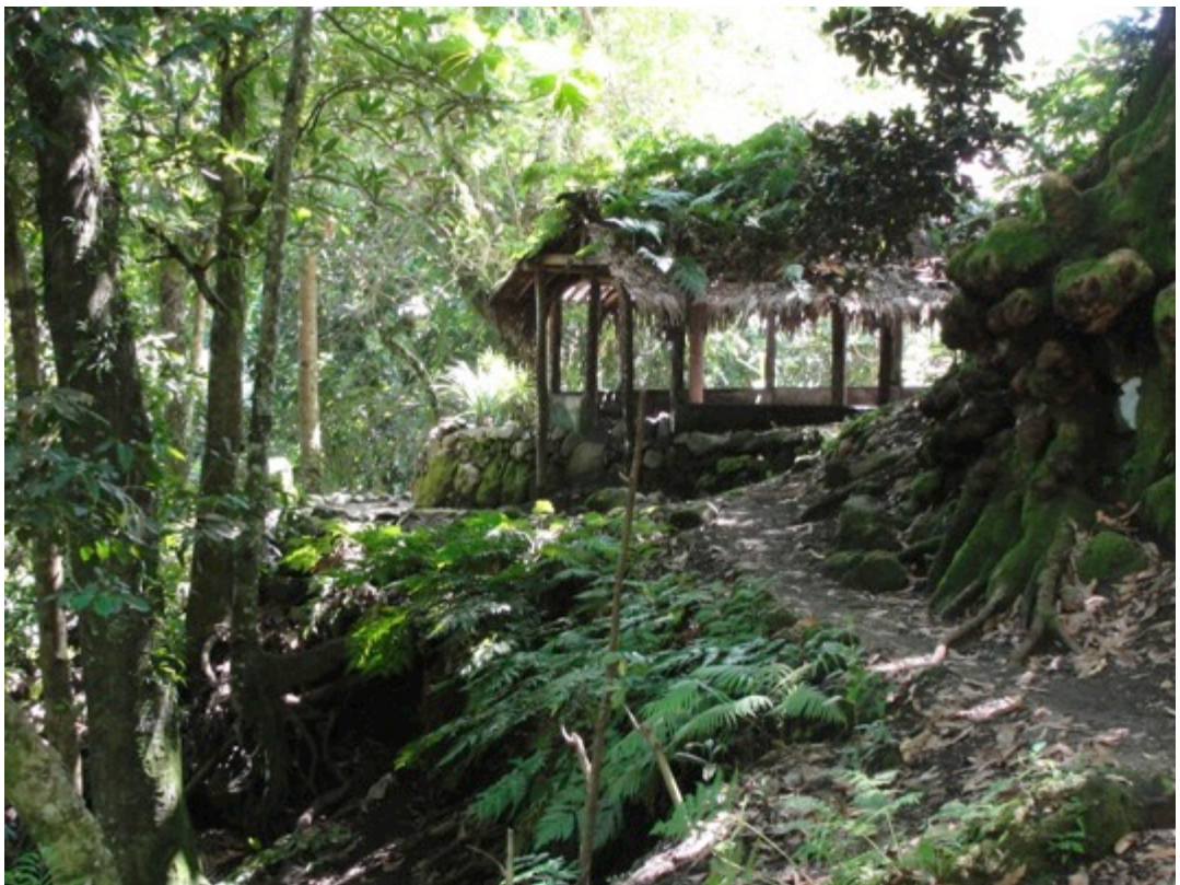
Figure III.01: View of a decayed house situated close to the main path, ne-metsal lap , Beop Hamlet, Tasmat village, 04/05/2011.
