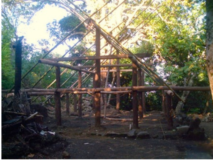
Fig. 5.09: Complete kitchen house structure, with breadfruit leaves attached to it, Lañramo hamlet, Tasmāt village, 25/07/2011.
