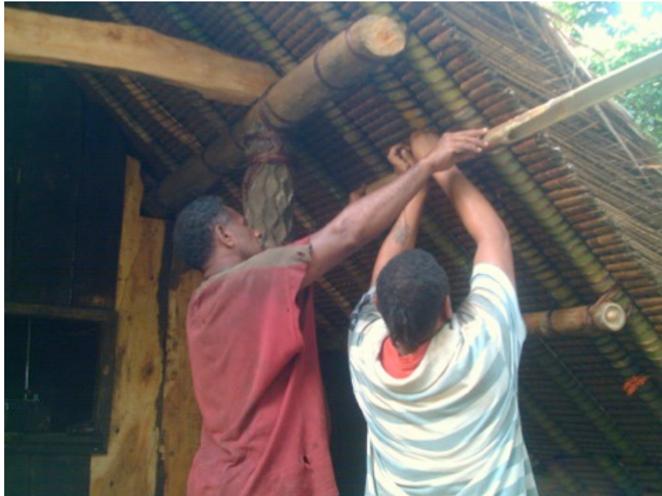
Fig. 4.08: Attaching nu-wutil bamboo to the n-eañ kuk , Luwör hamlet, Leqel village, 27/06/2011.
