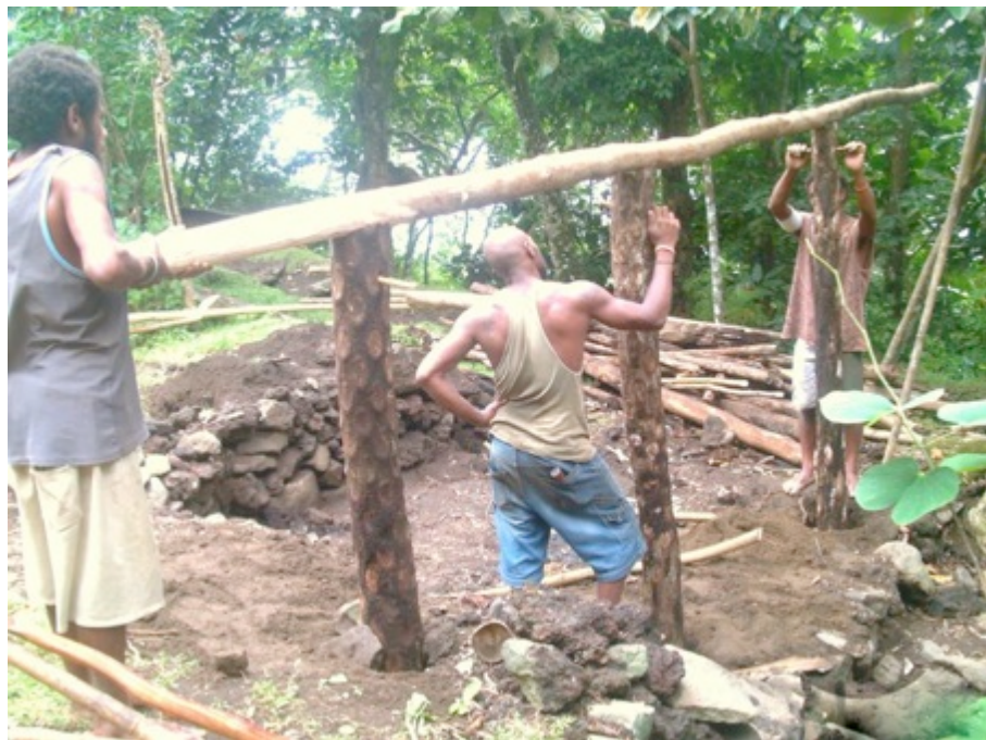
Fig. 5.08: Adjusting one side ne-rēmtiñ posts and ne-selgasēg beam, Leverē hamlet, Leqel village, 01/06/2011.
