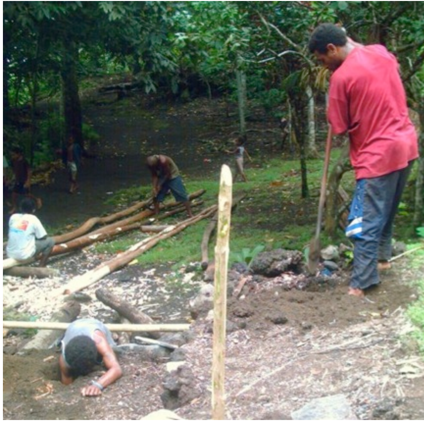
Fig. 5.07: Noel and Matias Rañ digging holes to erect the house's posts, Leverē hamlet, Leqel village, 01/06/2011.
