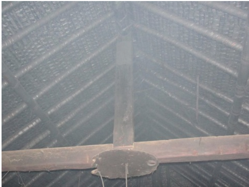
Fig. 3.06: No-wolwol transversal wooden beam, n-eaṅ kuk of Leo Swithun, Palon, Espiritu Santo, 22/04/2011.
