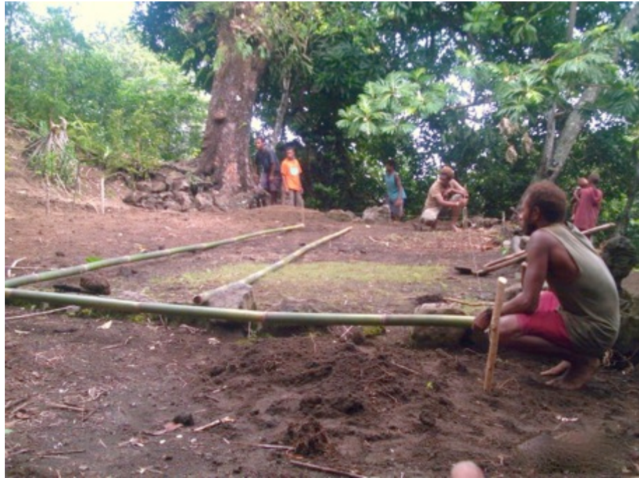
Fig. 5.05: Marking and measuring the house, tow n-eañ , Lañramo hamlet, Tasmat village, 30/06/2011.
