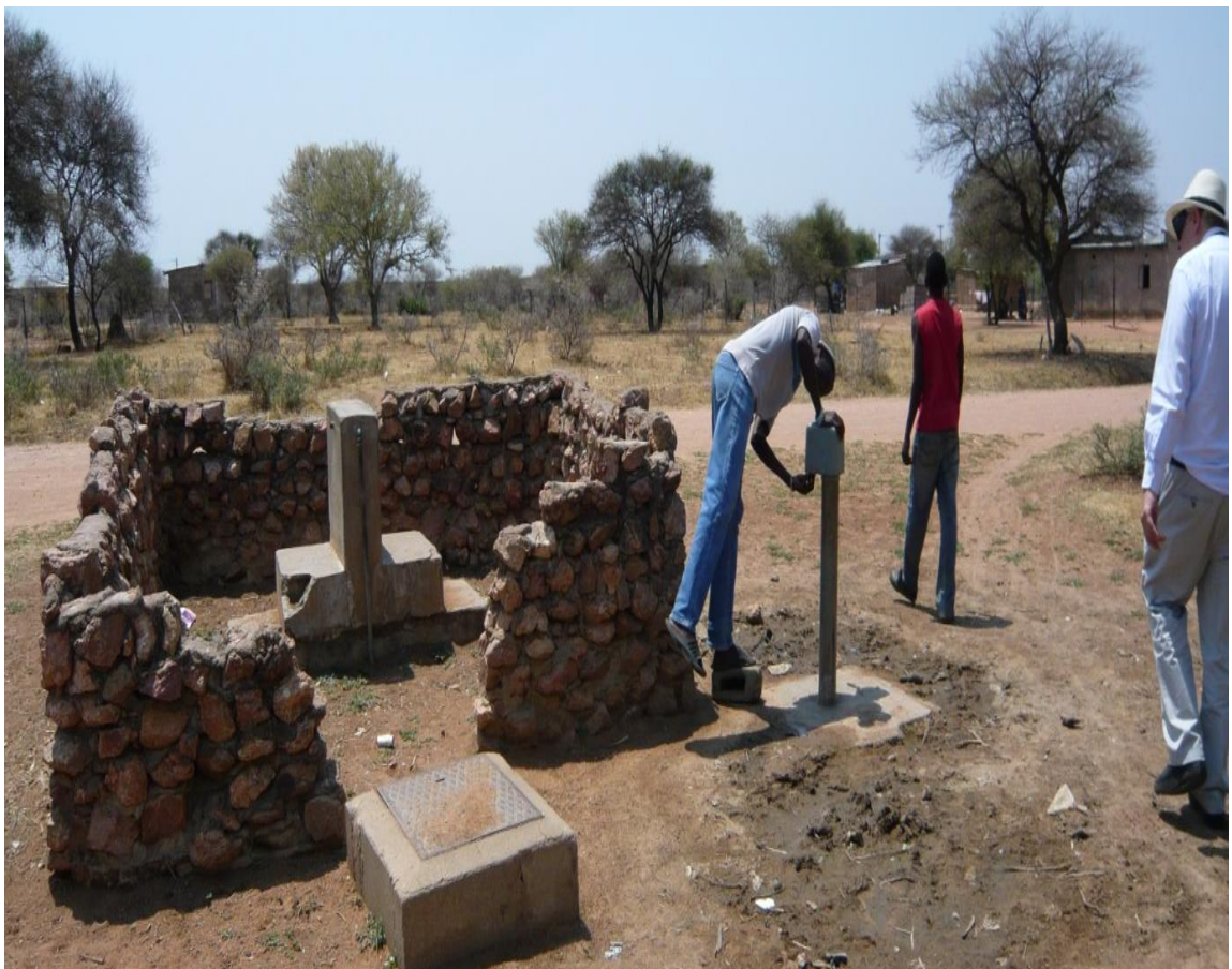
Photograph 9.1 Standpipes old and new (May 2013)
