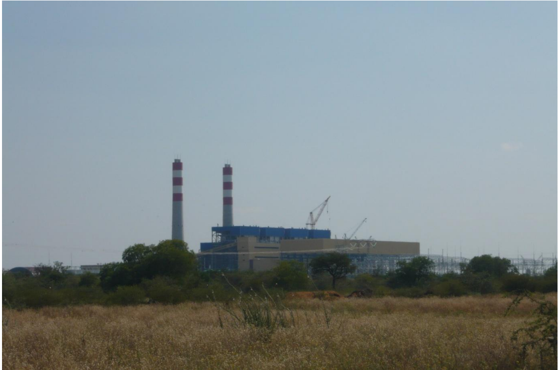
Photograph 5.3 Moropule B Power Station 2013
