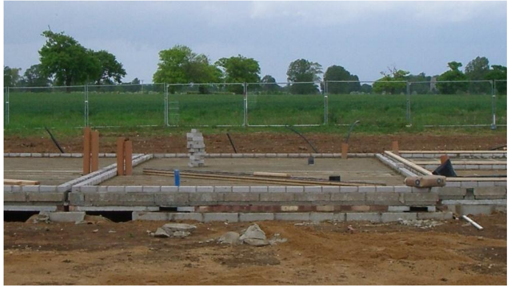
Figure 2-5: Photograph showing oversite foundation slab and brick and block wall below damp proof membrane (image source: J. Monahan)
