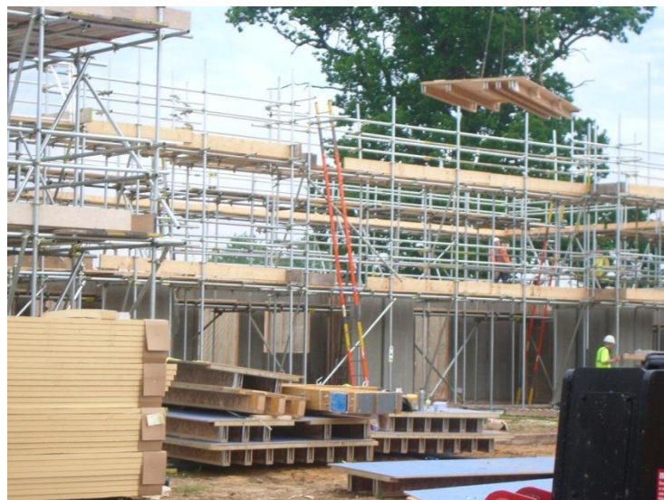
Figure 1-13: Panel system construction (image source: John Youngs Homes Ltd)
