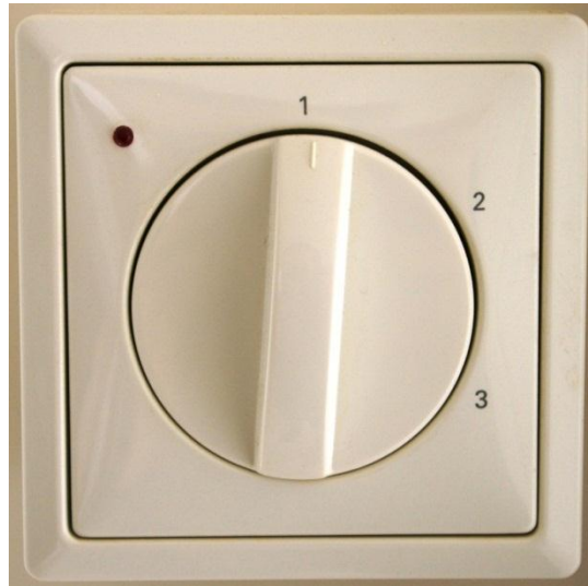
Figure 4-3: Image of air flow controller (source: J.Monahan)
