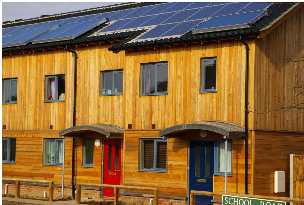
Figure 1-15: SOLAR showing front elevation with PV and solar hot water collectors
