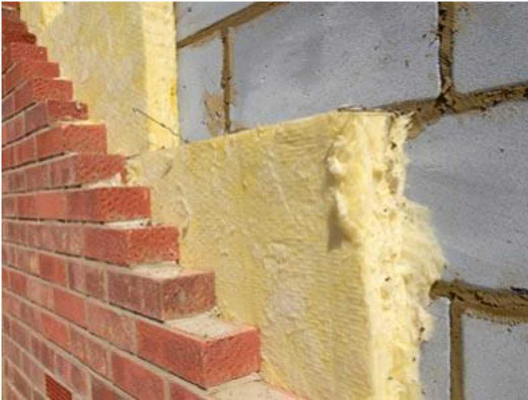
Figure 2-6: Photograph showing a conventional brick and block wall construction with a full fill mineral wool batt insulated cavity (image source: S. Monahan)
