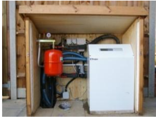
Figure 1-19 Heat pump external housing and contents
