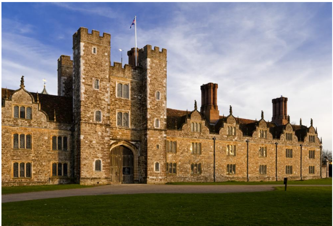
Figure 2.4: The front elevation, and entrance at Knole, Sevenoaks. Copyright: The National Trust.
