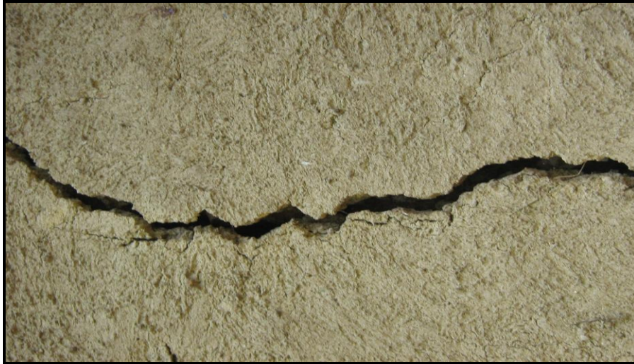
Figure 5.3: A crack in the wall of Wilbert M.'s house
