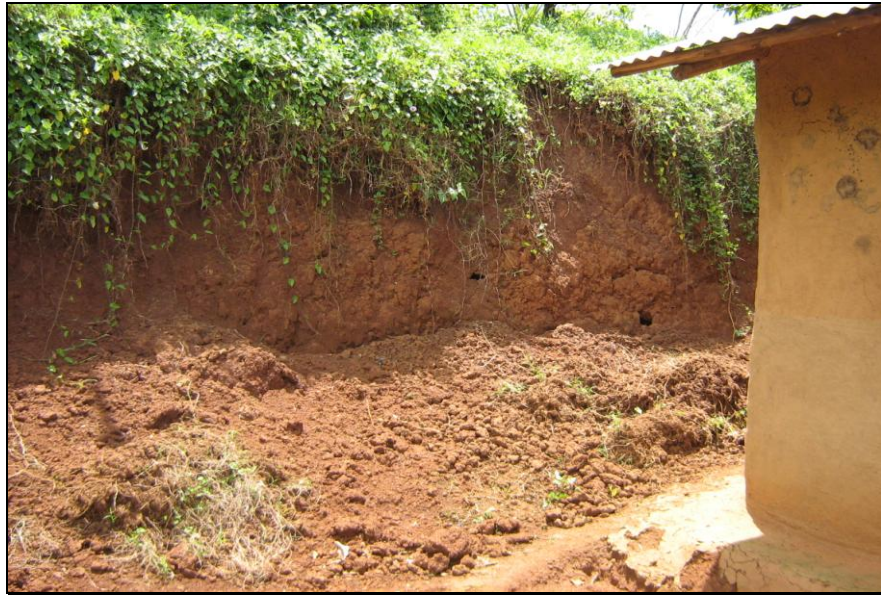
Figure 5.2: A house threatened by a landslide
