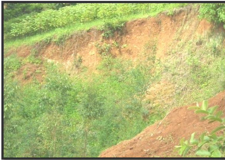
Figure 5.1: Close-up of the 1997 landslide scarp
