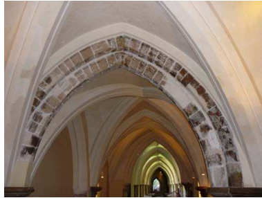
Figure 4.4: Interior of the South Cloister, showing original brickwork.
