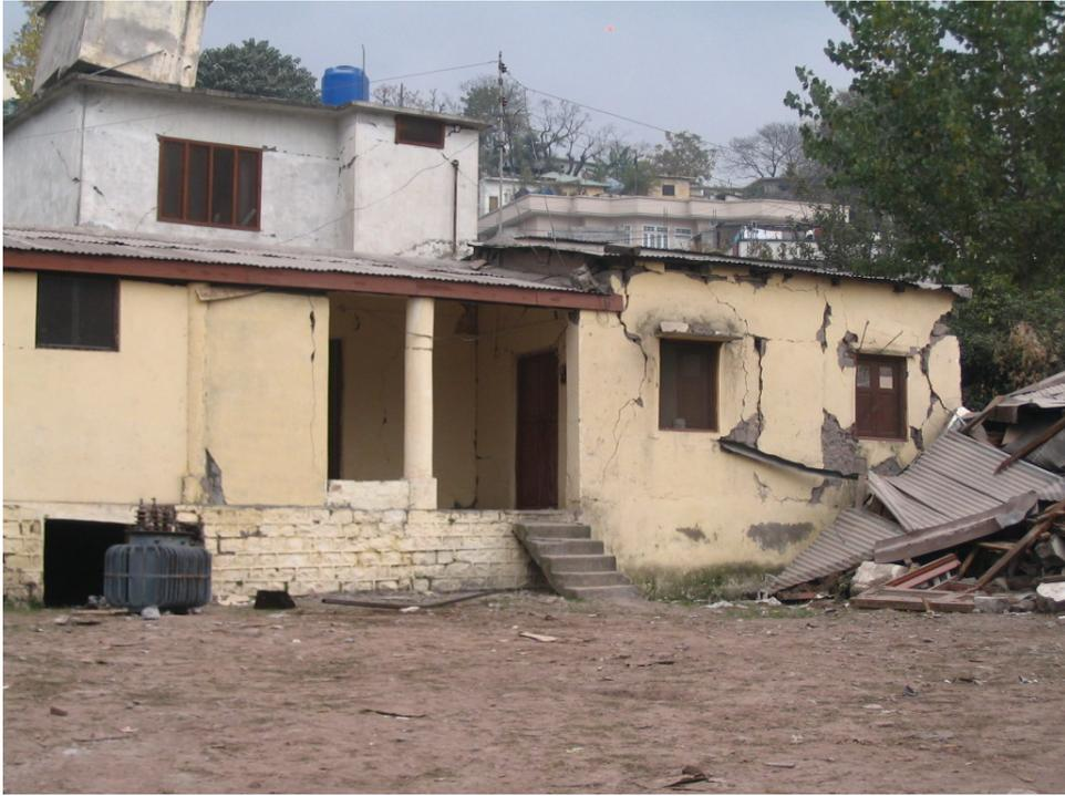
**Figure 3.23: Shear cracks through the concrete block masonry wall of a residential building, moderate damage, Muzaffarabad**
