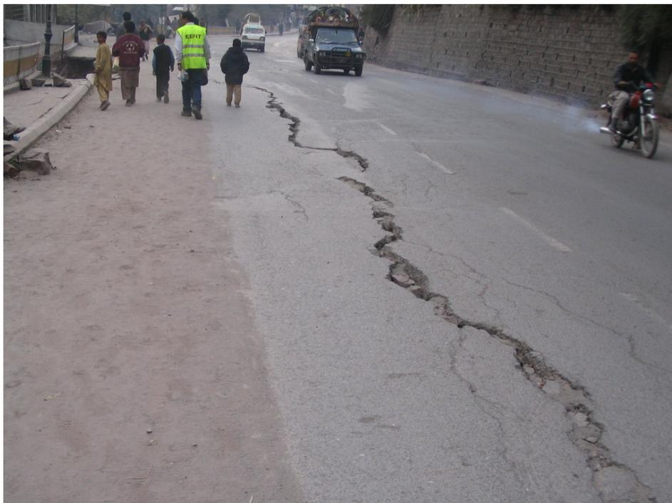
**Figure 4.28: Cracks through a major route through Muzaffarabad due to collapsed retaining wall section**
