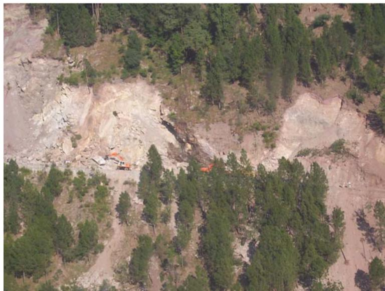
**Figure 4.23: Shallow depth landslide exposing the underlying rock. Mixture of rock fall and soil flow block the northern access road to Balakot City, NWFP (photo by Kathrin Renner (Arup) and US Army)**
