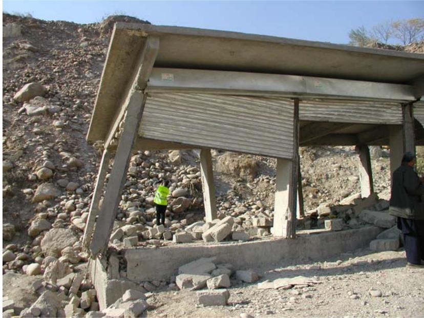
**Figure 4.31: Rock falls and showers. Cobble and boulder material on slopes showered down on road transport during the earthquake. This site in Muzaffarabad City is above and behind the cracked road edge visible in Figure 4.5**
