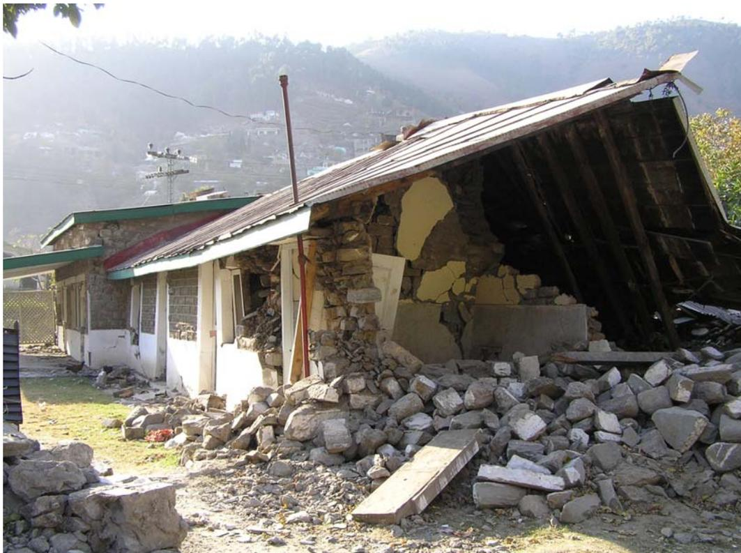
**Figure 3.13: Extensively damaged stone URM building with metal roof in Balakot, used by the local audit officer**
