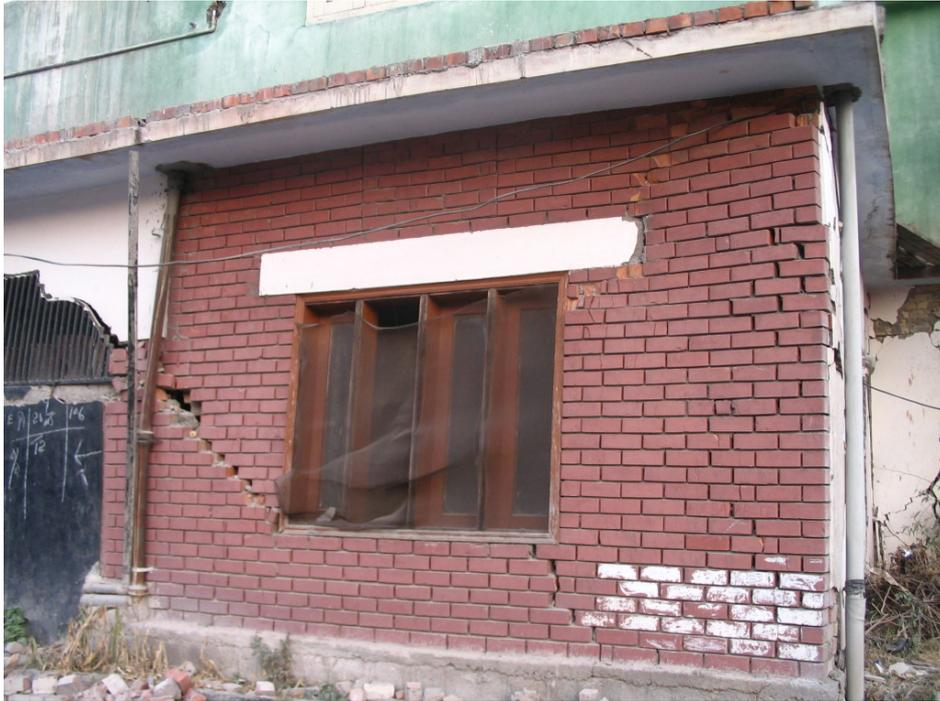
**Figure 3.21: Diagonal shear cracks through window on a brick URM residential building, moderate damage, Muzaffarabad**
