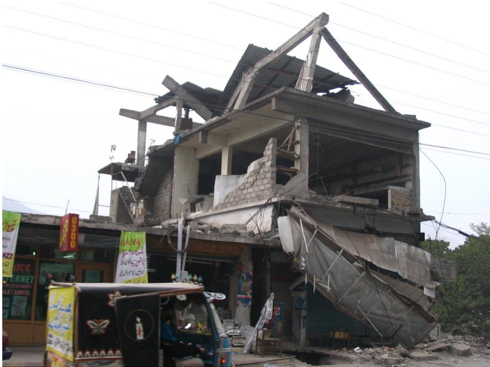
**Figure 3.29: Collapsed RC frame of upper floor of 3-storey commercial building with concrete block masonry infill walls. Failure at beam/column connections of upper floor frame, Muzaffarabad**
