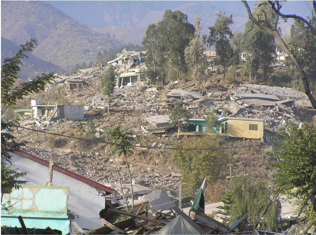
**Figure 3.11: Collapsed and extensively damaged concrete block URM residential units on a hill northwest of Balakot city centre (zone 1)**
