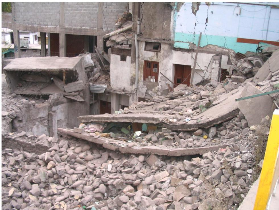
**Figure 3.26: Collapsed 2-storey concrete block URM commercial building. Floor and roof collapse possibly due load bearing wall failure in shear and out-of-plane and high inertia loads from RC slabs, Muzaffarabad**
