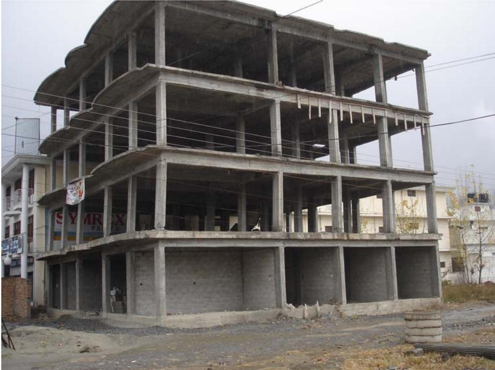
**Figure 3.48: Permanent drift at the first floor of an RC frame and slab 4-storey commercial structure under construction, Abbottabad. Ground floor drift may have been prevented by the infill masonry walls**
