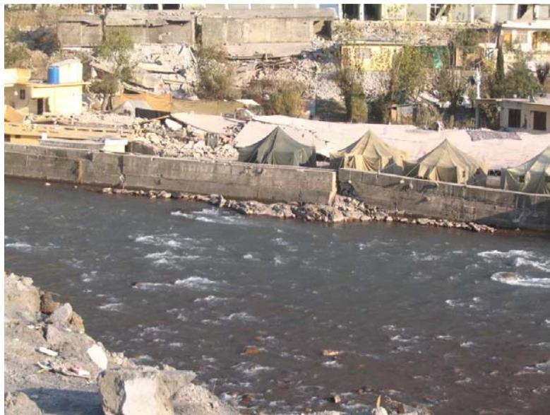
**Figure 4.21: Displaced concrete gravity retaining wall by Kunhar River in Balakot**
