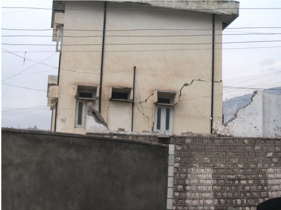
**Figure 3.27: Diagonal shear cracks through concrete block wall of RC frame and slab commercial building with masonry infill walls, moderate damage, Muzaffarabad**
