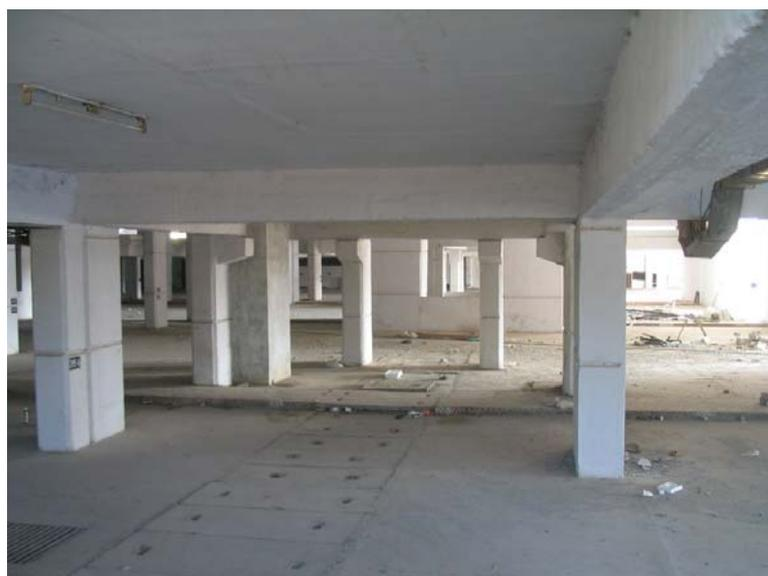
**Figure 3.51: Soft-storey basement in a building adjacent to the collapsed building at Margalla Towers**
