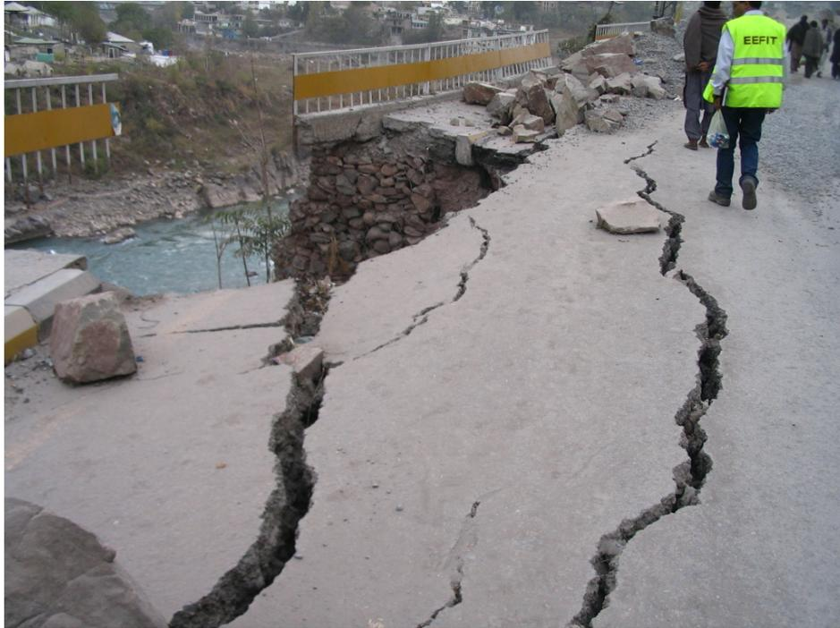
**Figure 4.27: Retaining wall collapse leading to unstable pavement and road sections on a major route through Muzaffarabad**
