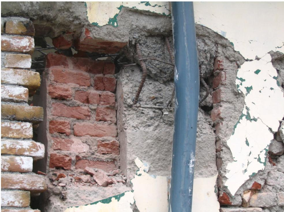
**Figure 3.47: Example of failed beam/column connection due to poor shear and confinement reinforcement detailing**
