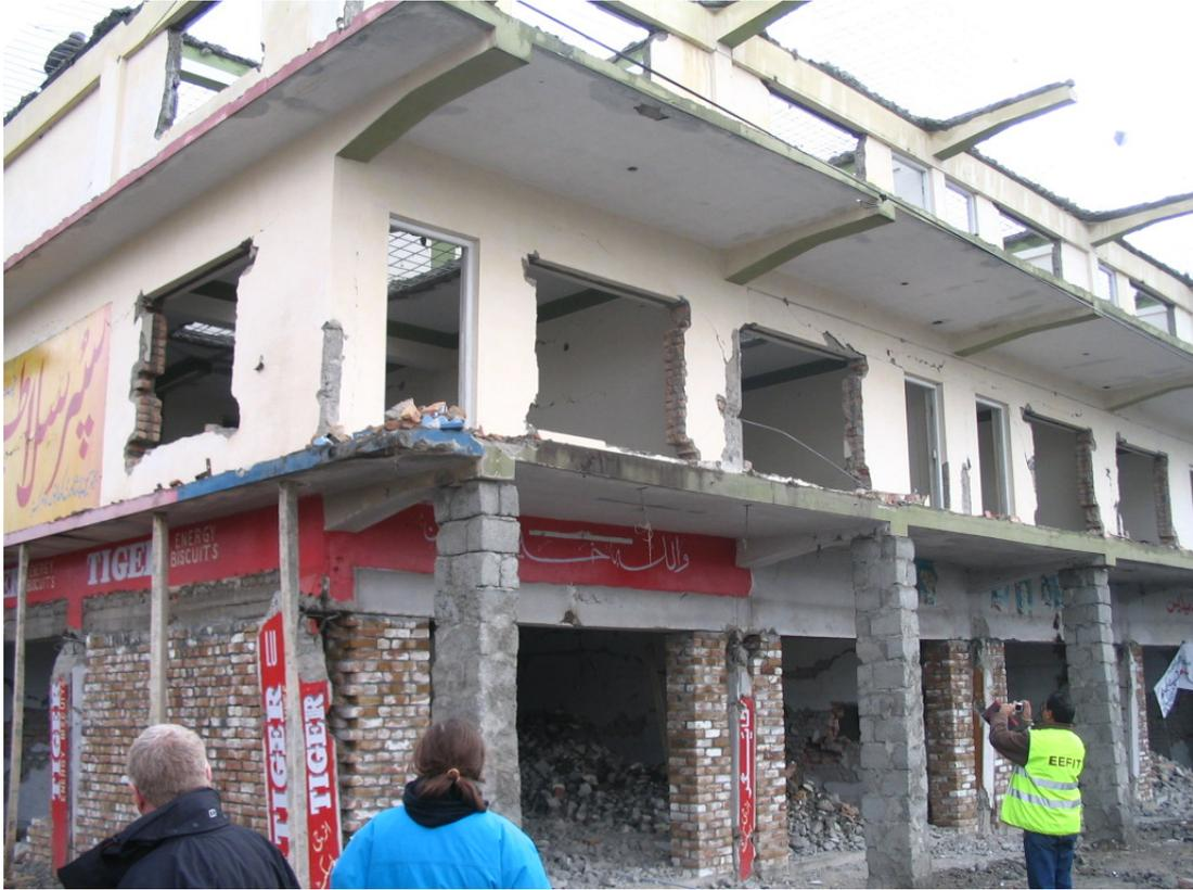
**Figure 3.7: Moderately damaged commercial/retail building of RC frame and slab construction with brick masonry infill in Abbotabad**
