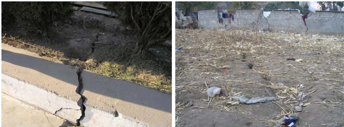
**Figure 2.8: Photos of ground cracks observed by EEFIT and Dr Bijan Kazai (of Columbia University, New York, and member of EERI team) to run through Balakot in a NNW-SSE direction**
