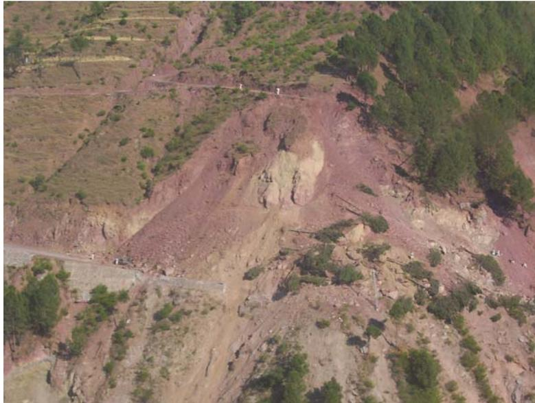
**Figure 4.22: Shallow depth landslide and slumping of soils blocking an access road to Balakot City, NWFP (photo by Kathrin Renner (Arup) and US Army)**
