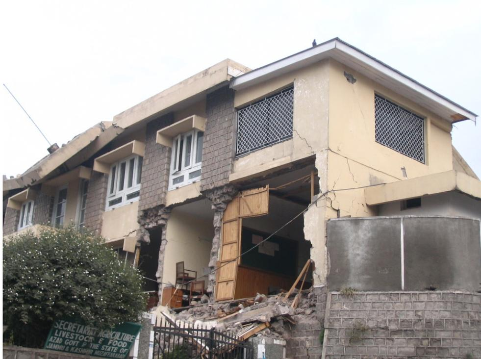
**Figure 3.39: Collapsed wall sections of the concrete block URM, 3-storey building of the AJK Secretariat of Agriculture, Livestock and Food. Collapsed RC slab roof, extensive damage**
