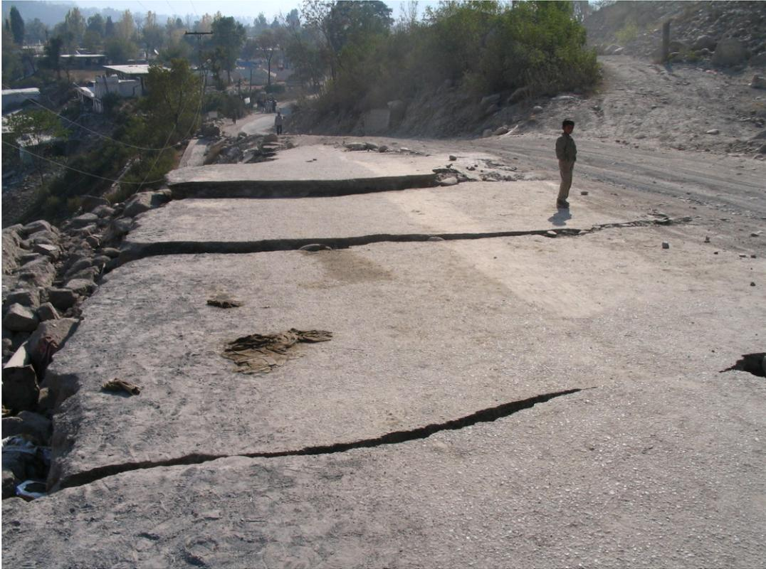
**Figure 5.10: Ground cracks through a road in Muzaffarabad**
