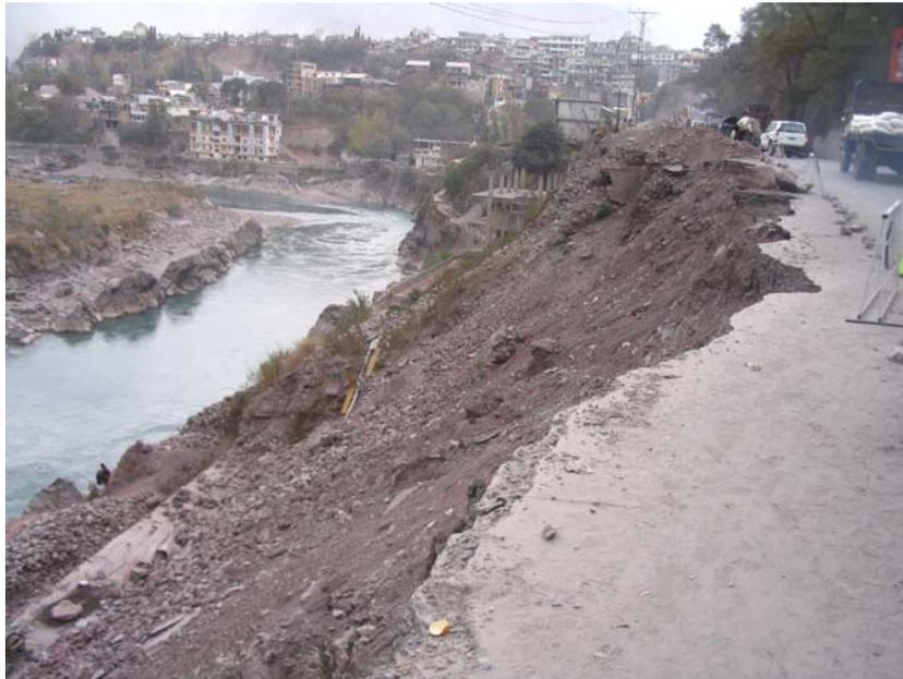
**Figure 4.29: Slope failure adjacent to a major route through Muzaffarabad City, danger of further erosion of the road surface**
