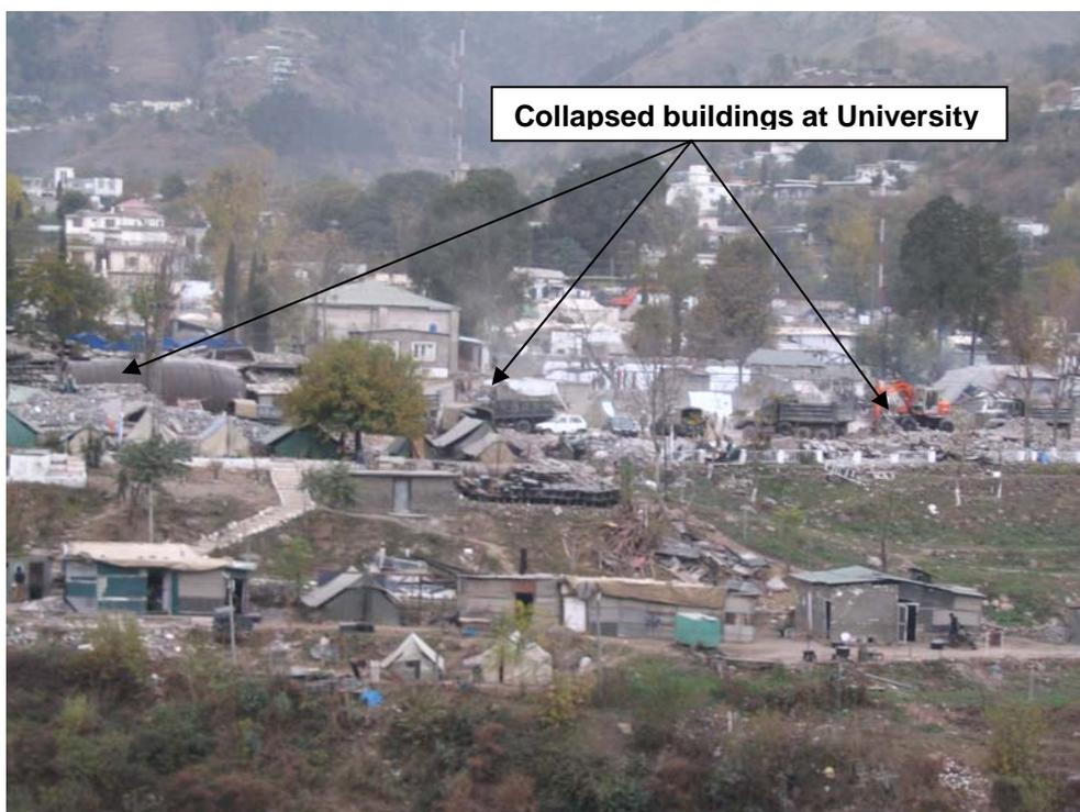
**Figure 3.42: Collapsed concrete block URM buildings of the University of AJK, Muzaffarabad**
