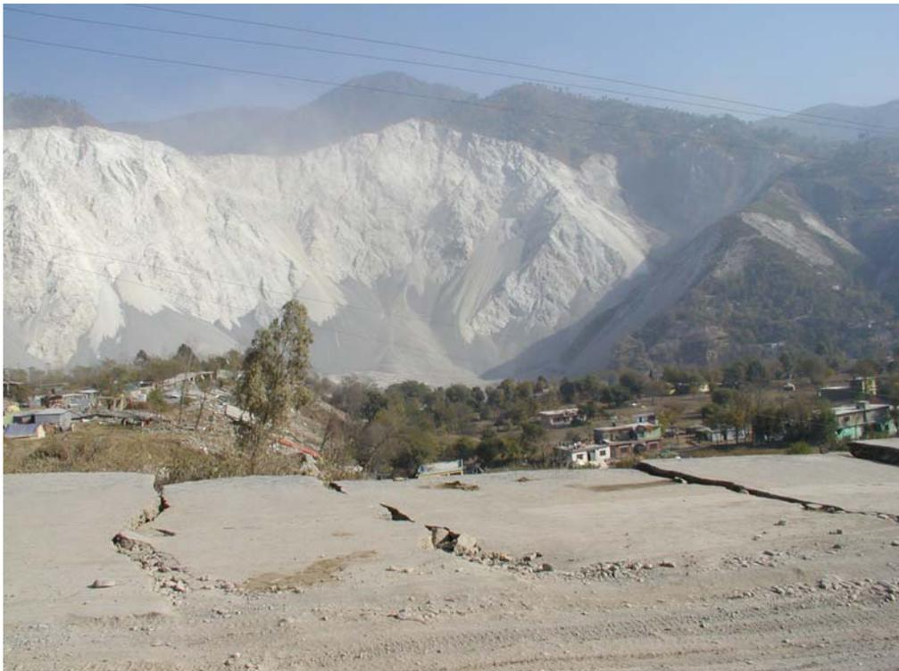
**Figure 4.5: Kashmir earthquake October 8, 2005. Landslide in dolomite mountainside just north of Muzaffarabad at Chela Bandi. Also note cracks through road in foreground and damage to buildings in mid-distance**
