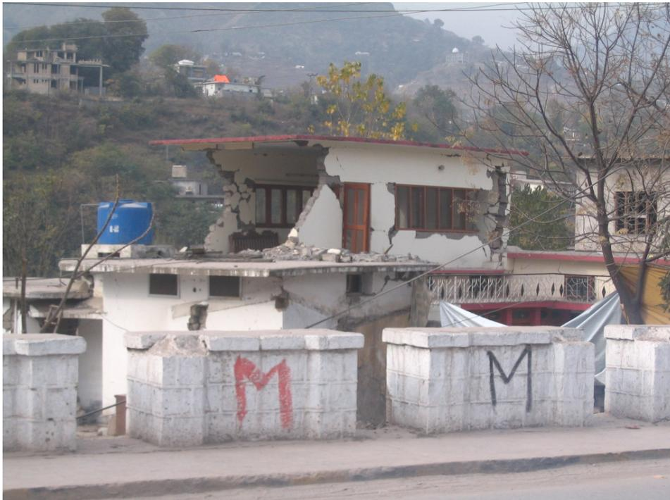
**Figure 3.22: Partially collapsed upper floor walls of a 2-storey concrete block URM residential building with RC slab floors and roof. Shear and out-of-plane failure of concrete block bearing walls, Muzaffarabad**
