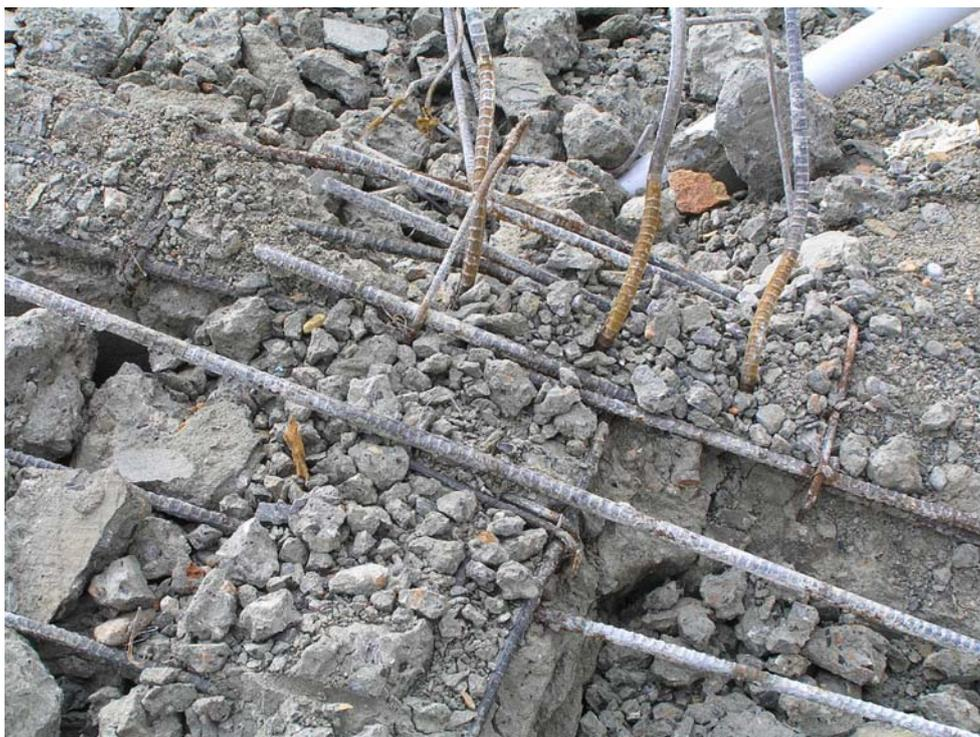
**Figure 3.44: Lack of continuity of reinforcement detailing at the beam/column connection**
