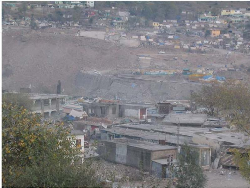
**Figure 4.20: Collapsed retaining wall and concrete facing structures in Balakot**
