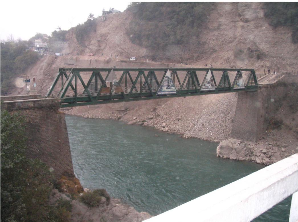
**Figure 5.8: Slightly damaged pedestrian bridge across Nelum River, Muzaffarabad. Steel truss single span simply supported on brick masonry abutments**
