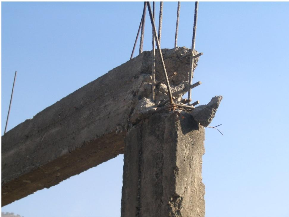
**Figure 3.30: Example of poor beam/column reinforcement detailing. No proper connection of column and beam reinforcement for moment resisting action**
