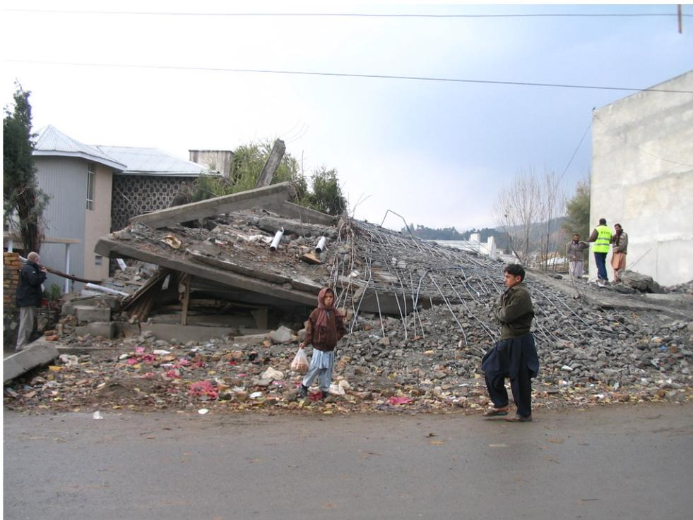
**Figure 3.43: Collapsed RC 3-storey commercial and residential building. Collapse appears to be due to failure of beam/column connections, Abbottabad**
