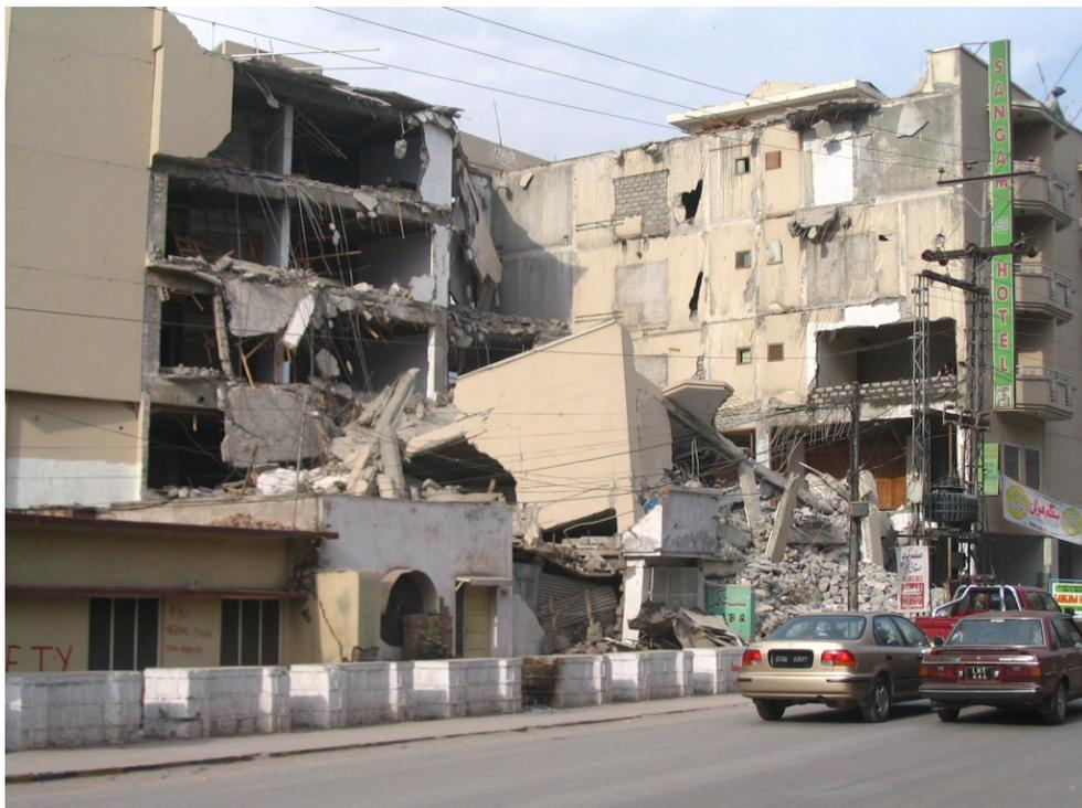
**Figure 3.32: Collapsed section of Samgam Hotel, RC frame and slab construction, 5-storey. Collapse due to failure at beam/column connections, Muzaffarabad**
