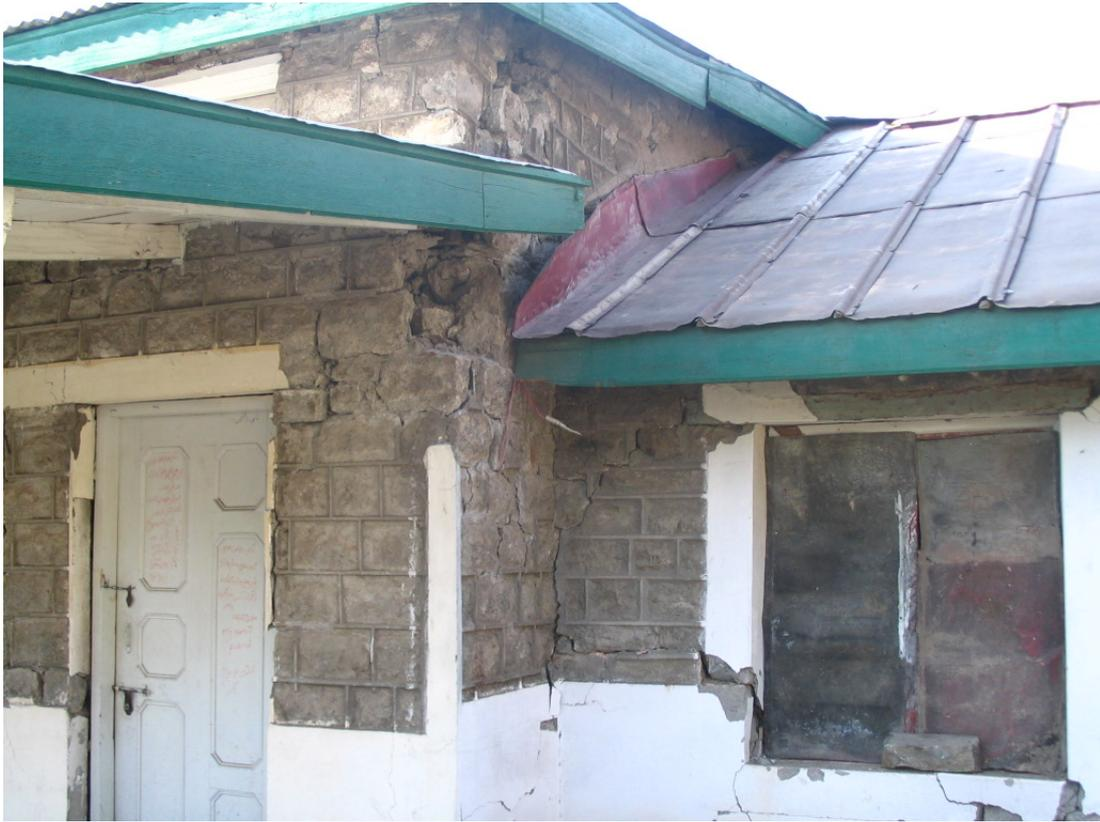
**Figure 3.14: Cracks through stone and mortar in a stone URM building adjacent to the extensively damaged stone building in Figure 3.5**
