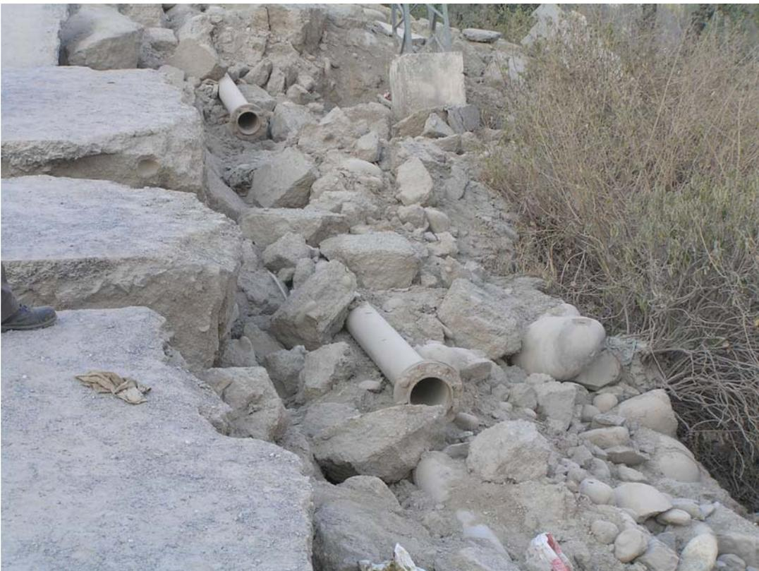
**Figure 5.11: Separated segments of a water supply system due to ground cracks, Muzaffarabad**
