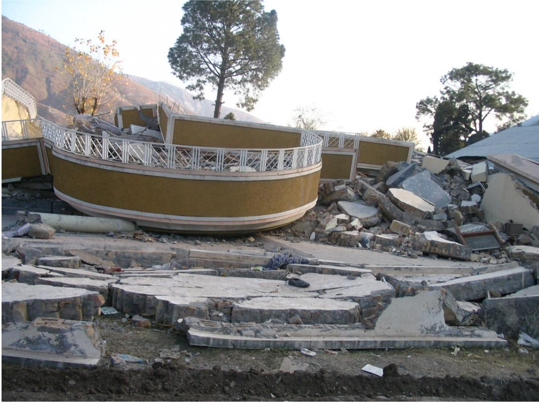
**Figure 3.5: Collapsed unreinforced brick masonry house in Balakot**
