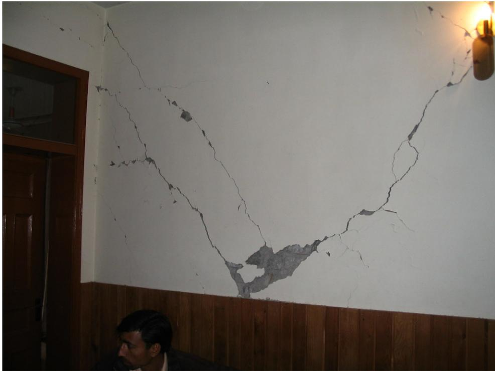
**Figure 3.37: Diagonal shear cracks through the brick URM walls of the Muzaffarabad Tourist Information Office, moderate damage**
