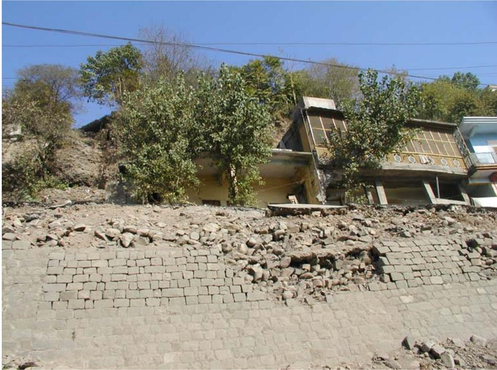
**Figure 4.25: Stone block masonry retaining wall in Muzaffarabad: slippage and collapse of this wall undermined buildings**
