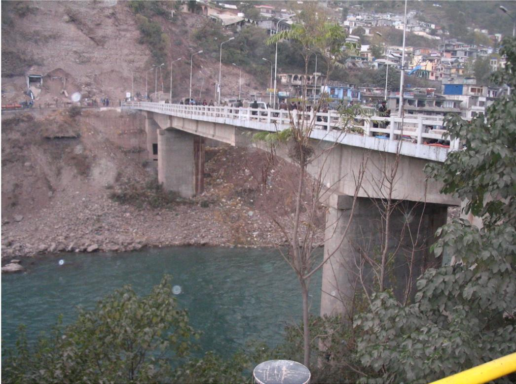
**Figure 5.7: Undamaged vehicle bridge across Nelum River, Muzaffarabad. RC spans simply supported on RC piers and abutment**
