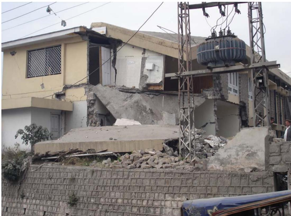
**Figure 3.4: Damaged 2-storey concrete block masonry building in Muzaffarabad**
