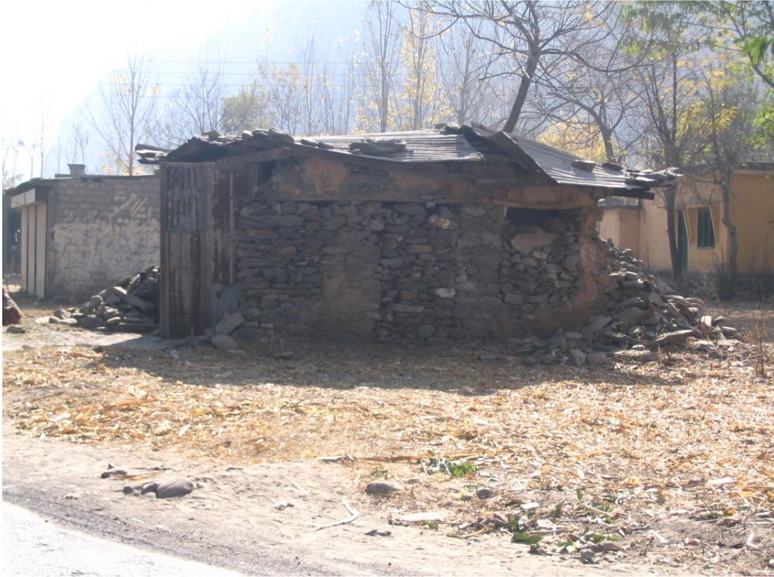
**Figure 3.1: Typical unreinforced stone masonry wall house (Katcha house)**
