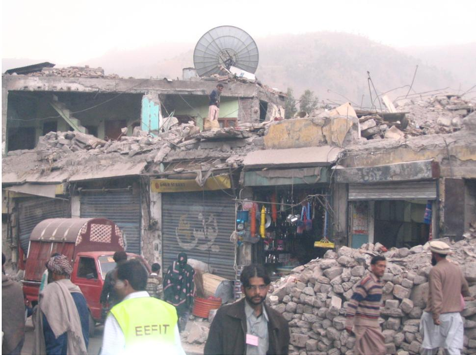
**Figure 3.25: Collapsed roof of 2-storey RC frame and slab commercial buildings with concrete block masonry infill walls. Failure of beam/column connections at upper floor. Intact ground floor walls and first floor slab, Muzaffarabad**
