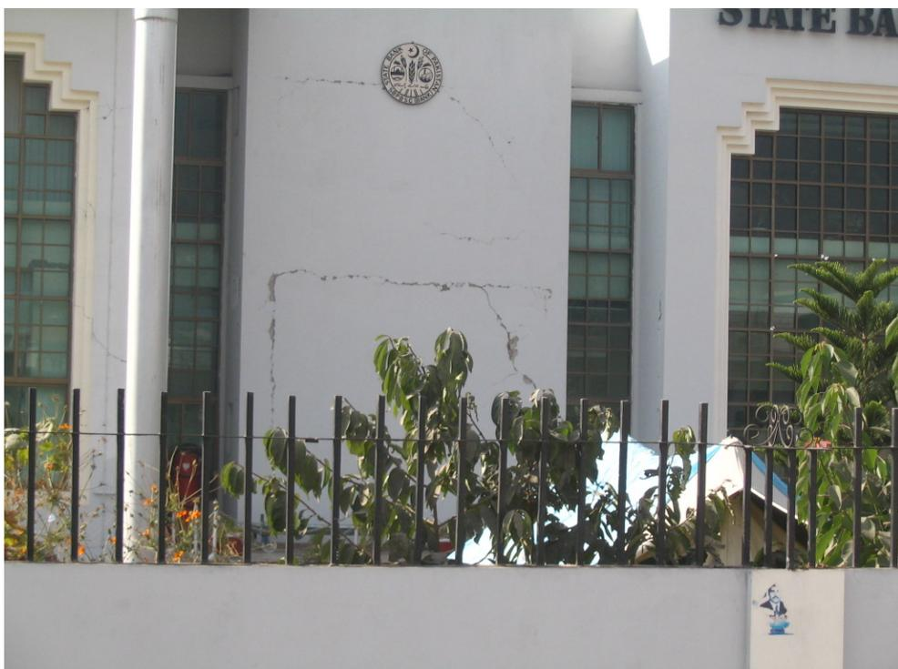
**Figure 3.38: Shear cracks through the brick URM walls of the State Bank of Pakistan building, moderate damage**
