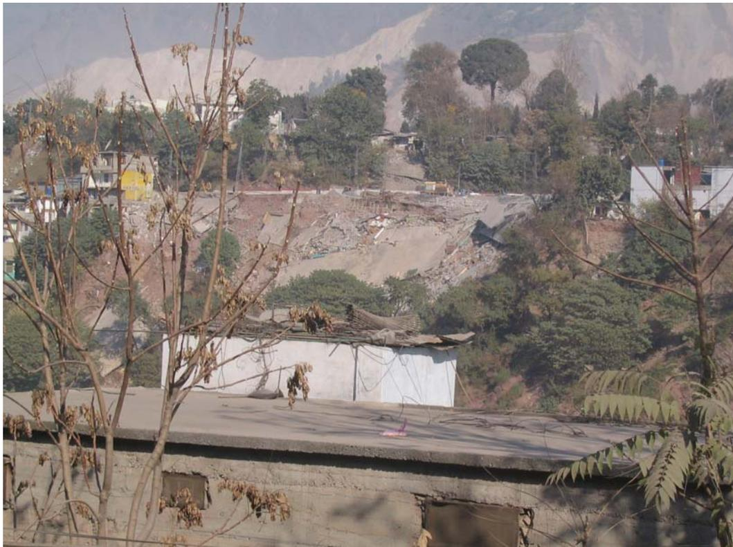
**Figure 4.24: Collapsed concrete retaining wall section in Muzaffarabad leaving the road above vulnerable to further collapse**
