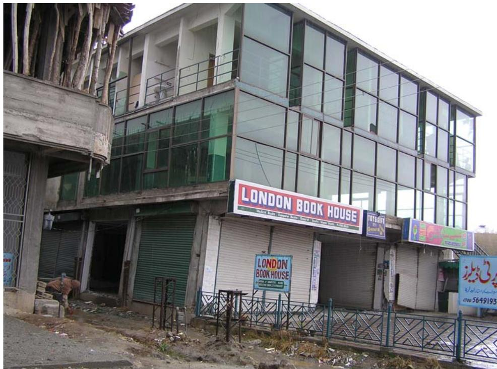
**Figure 3.49: Permanent drift at ground floor due to soft-storey in RC frame and slab 3-storey commercial structure, Abbottabad. The ground floor drift prevented large deformation at upper floors, hence glass frontage was intact**
