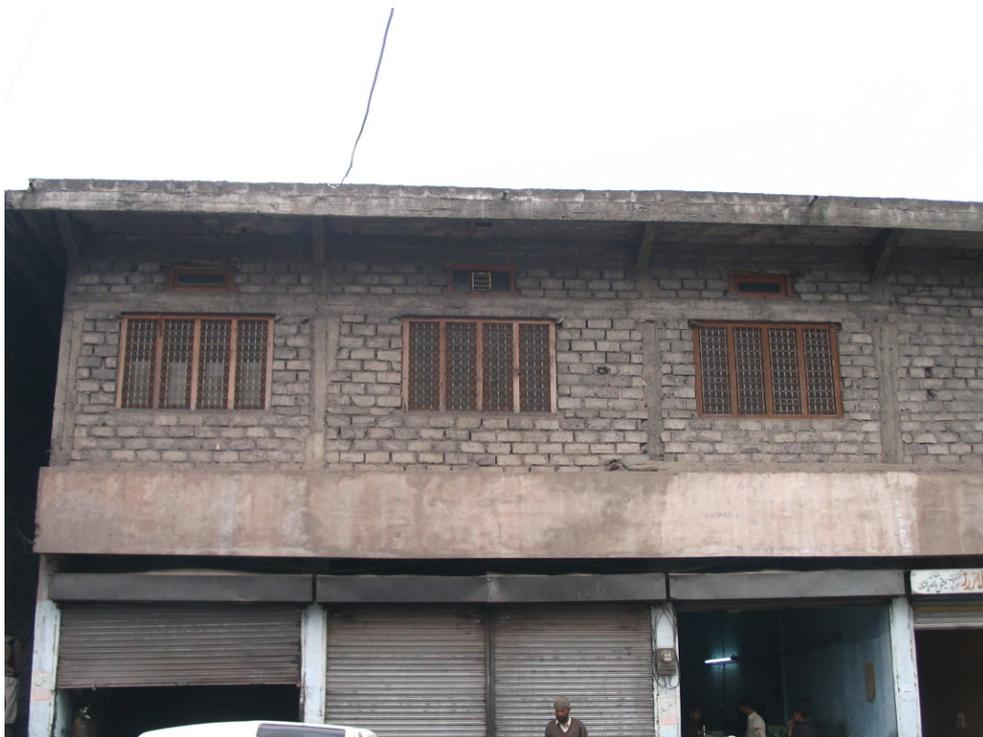
**Figure 3.28: Undamaged RC frame and slab commercial building with concrete block masonry infill walls. RC lintel beam continuous over the structure perimeter, Muzaffarabad**
