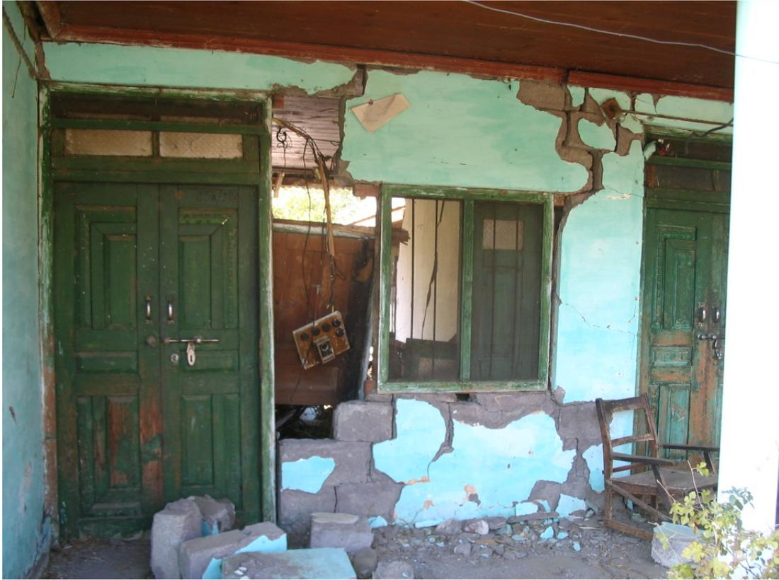
**Figure 3.3: Damaged unreinforced concrete block masonry office building south of Balakot**
