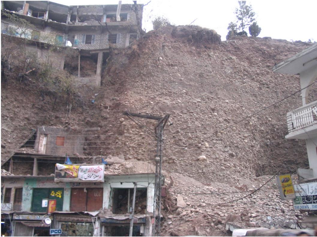
**Figure 4.18: Slope failure burying and extensively damaging the commercial building below and destabilising the residential structure above, Muzaffarabad**
