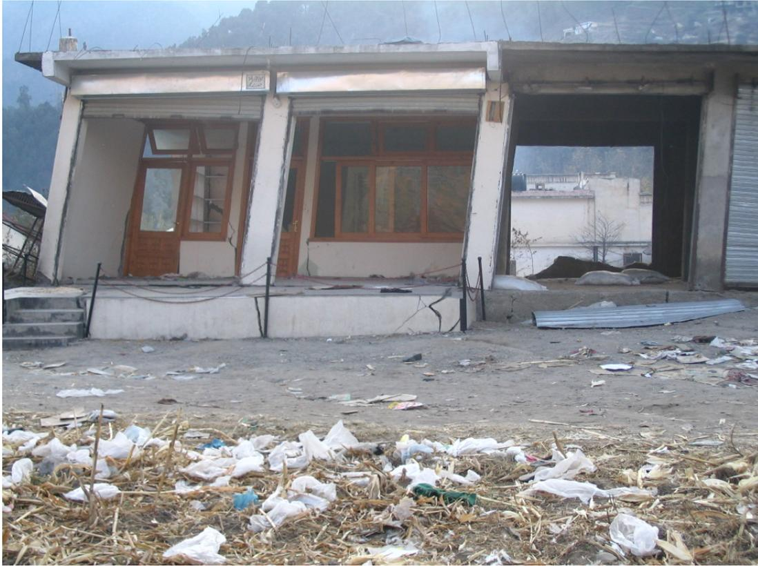
**Figure 3.18: Deformed RC frame structure with rotation at the column/slab connection**
