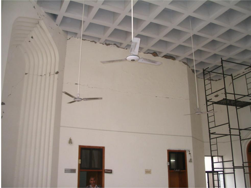
**Figure 3.35: Shear cracks through the brick masonry walls of the Muzaffarabad Supreme Court building. Cracking visible at the roof/wall intersection, moderate damage**
