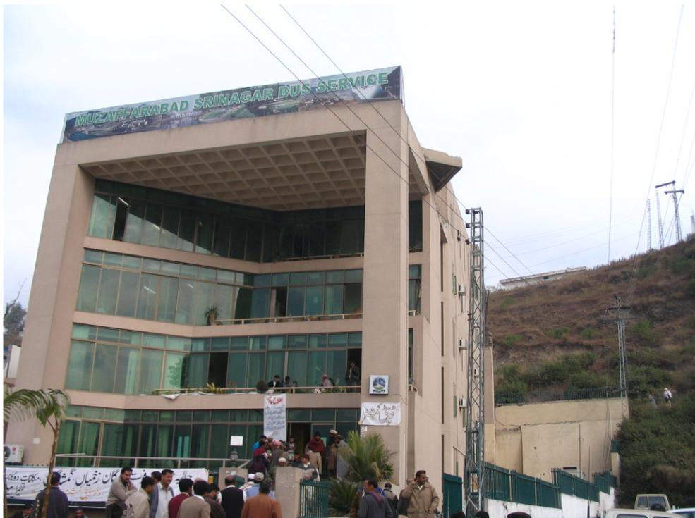
**Figure 3.34: Undamaged RC frame and slab commercial building, Muzaffarabad**
