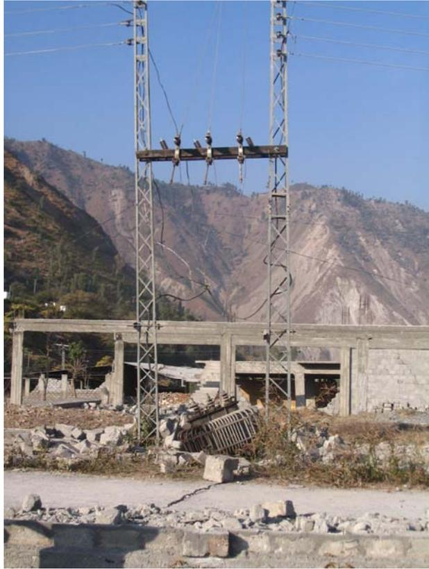
**Figure 5.12: Transformer unit detached from the supporting structure, Muzaffarabad**
