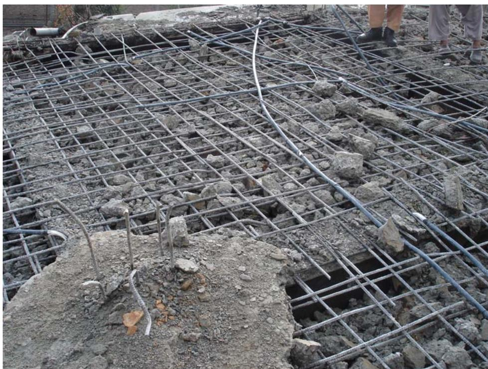
**Figure 3.45: Reinforcement layout of a collapsed slab revealed after removing the concrete**
