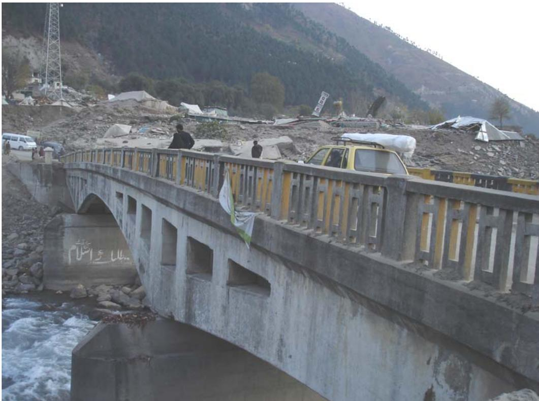
**Figure 5.1: Laterally displaced RC deck of the vehicle bridge in Balakot**
