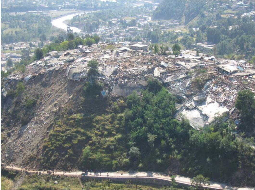
**Figure 3.12: Collapsed and extensively damaged concrete block URM residential units in zone 1 overlooking Balakot city centre (photo by Kathrin Renner (Arup) and US Army)**
