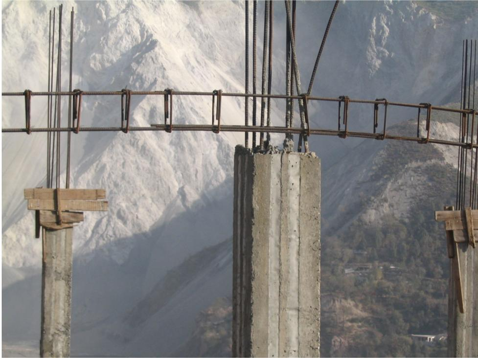
**Figure 3.31: Incorrect splicing of reinforcing bar at beam/column connection of a moment frame under construction. Shear links configuration inadequate for seismic shear forces**
