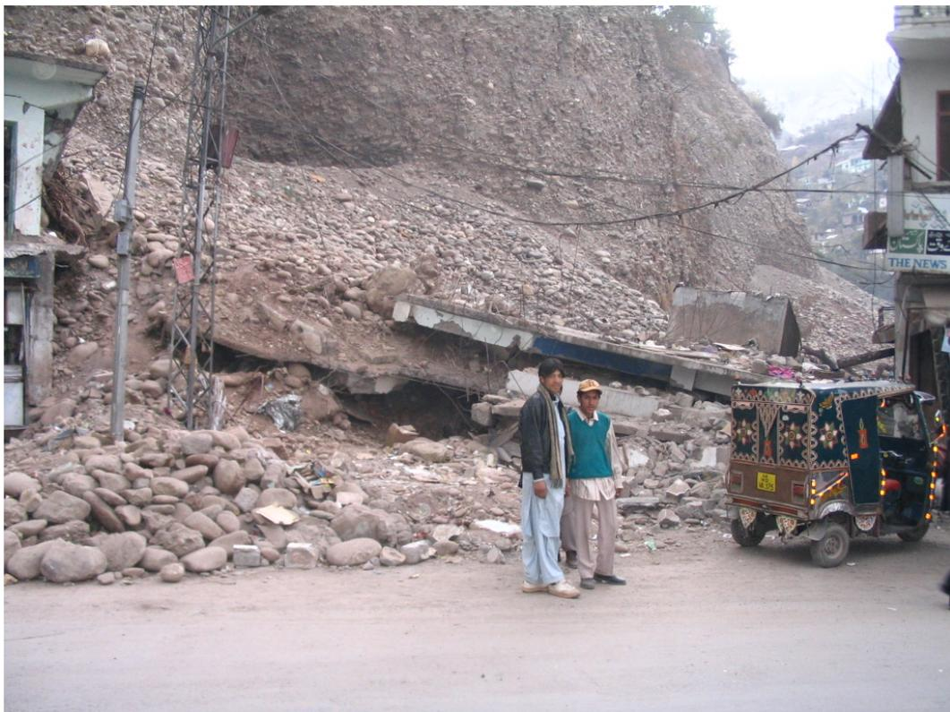
**Figure 4.19: Collapsed and buried commercial building from the soil and rock due to the slope failure shown in Figure 4.18, Muzaffarabad**
