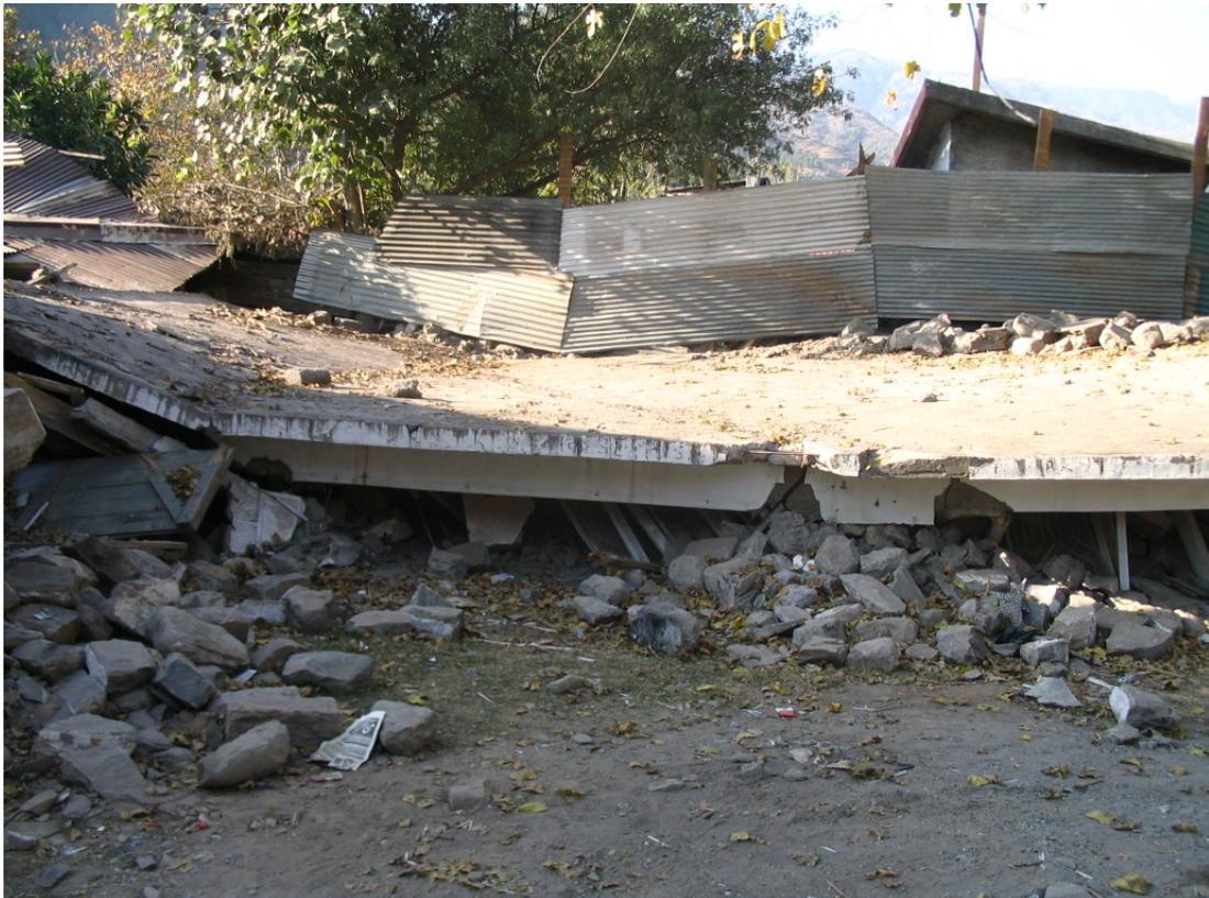
**Figure 3.15: Collapsed concrete block URM residential building in Balakot**
