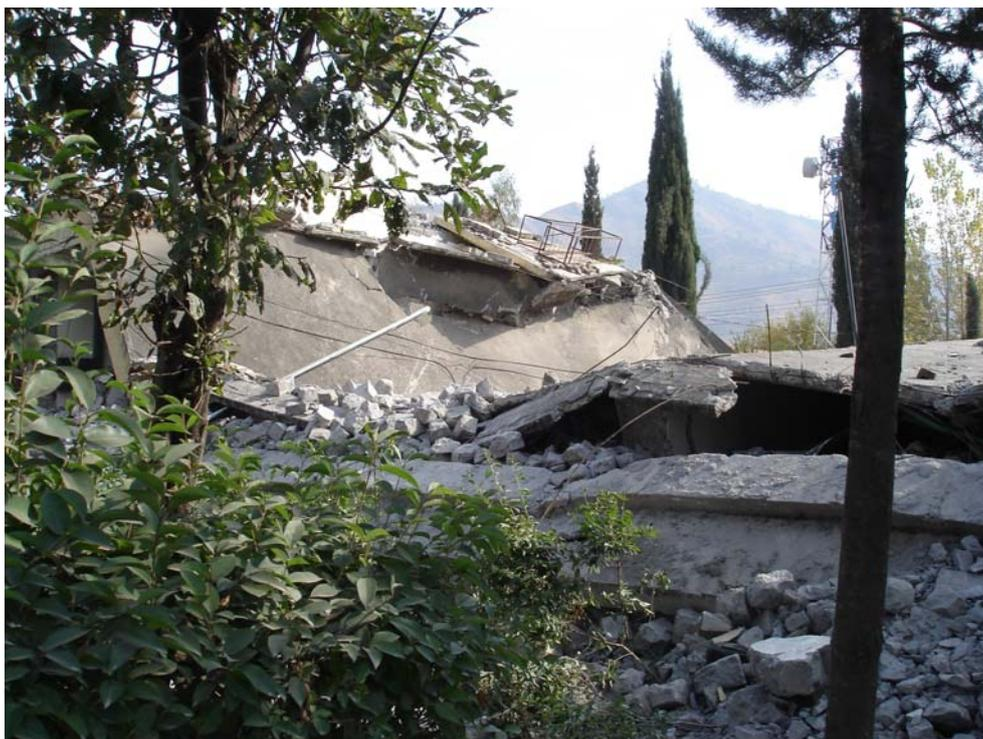
**Figure 3.41: Collapsed concrete block URM school building, Muzaffarabad**
