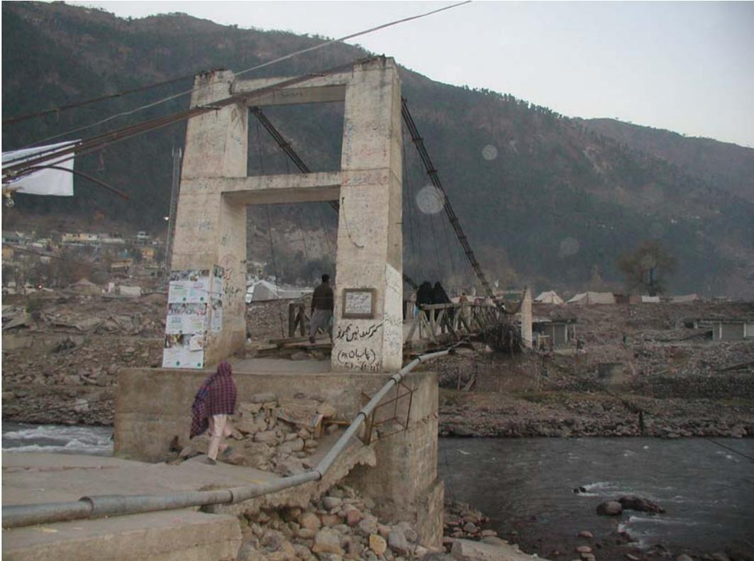
**Figure 5.2: Pedestrian bridge with damaged approaches in Balakot**
