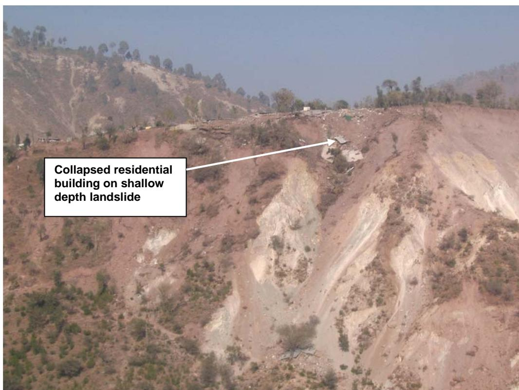
**Figure 4.17: Collapsed residential building due to a shallow depth landslide north of Muzaffarabad City**
