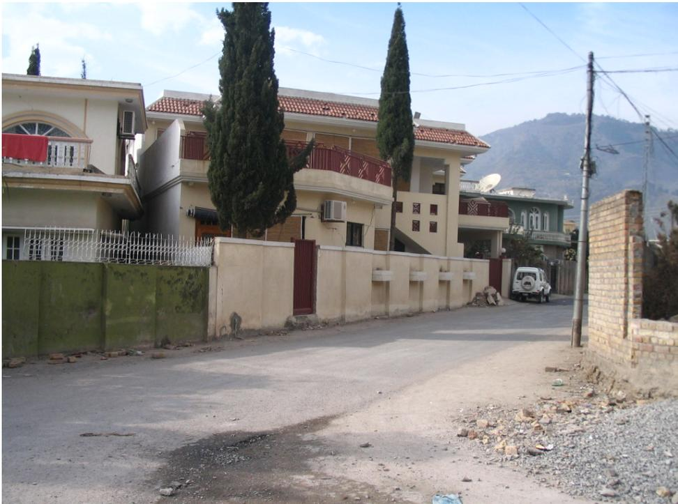
**Figure 3.24: Undamaged RC frame and slab residential building with concrete block masonry infill walls, Muzaffarabad**
