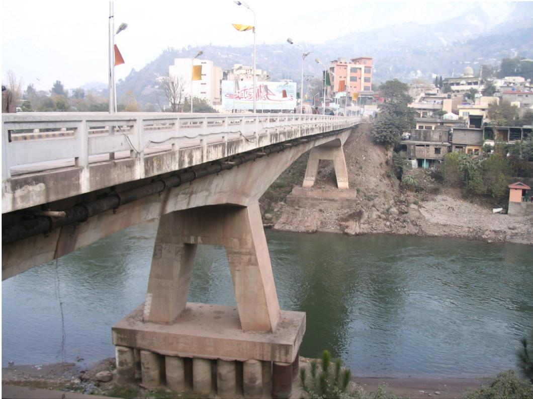
**Figure 5.5: Undamaged vehicle bridge across Jhelum River in Muzaffarabad. RC bridge deck, multi-span with integral abutments supported on RC piles with steel casing**
