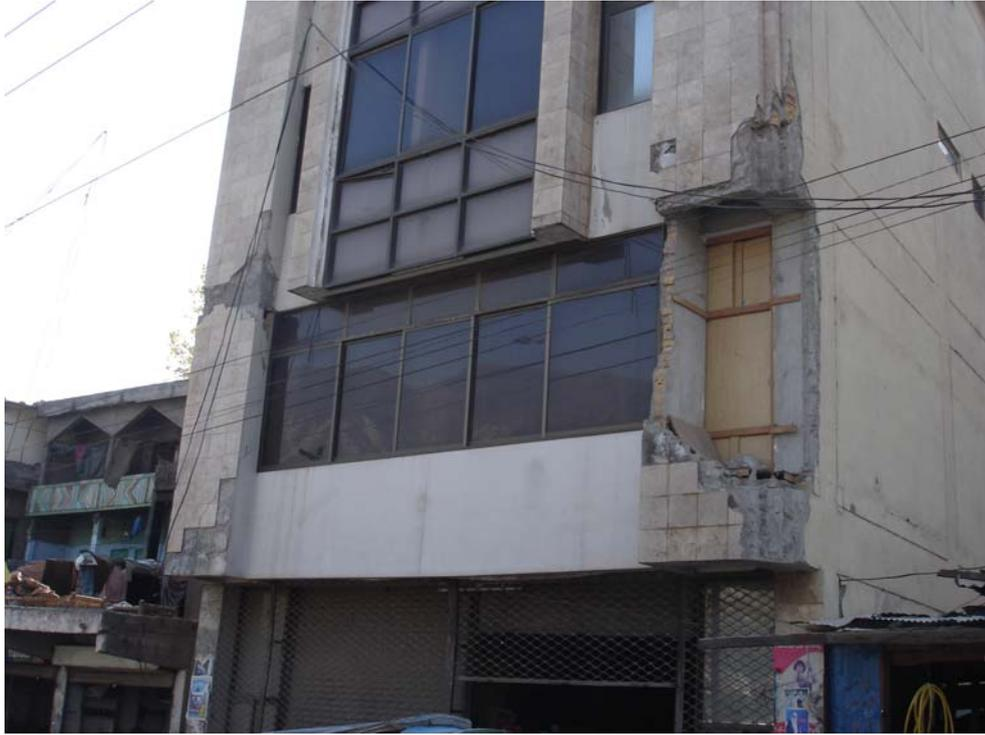
**Figure 3.33: Slightly damaged 4-storey RC frame and slab commercial building with concrete block masonry infill, Muzaffarabad**
