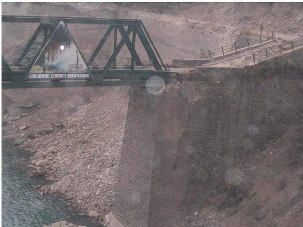
**Figure 5.9: Crack at one of the masonry abutments of the pedestrian bridge shown in Figure 5.8**
