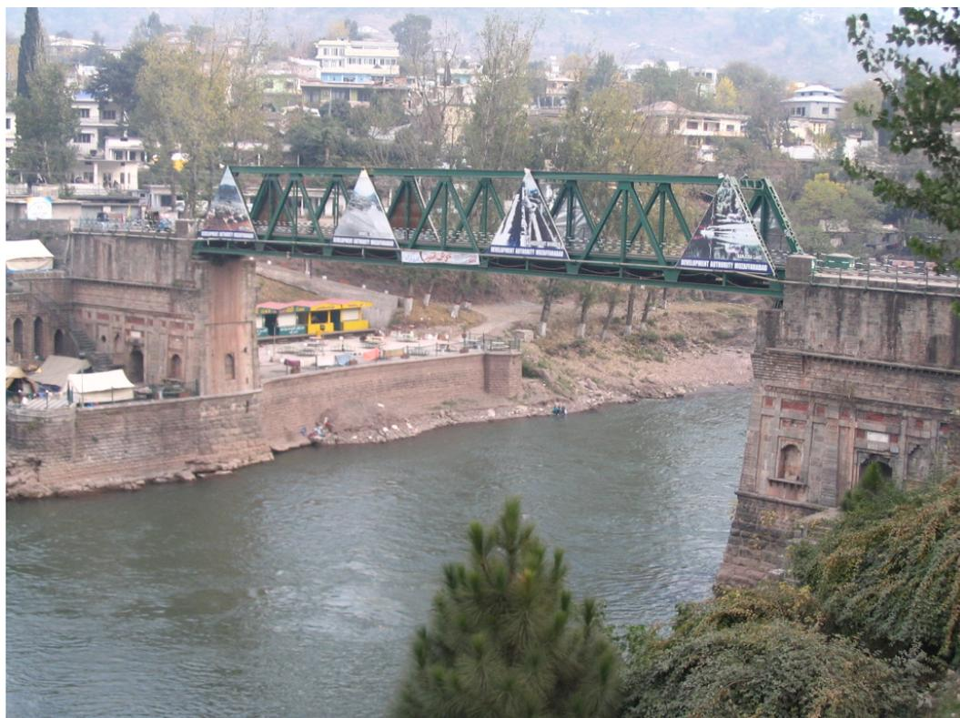
**Figure 5.6: Undamaged pedestrian bridge across Jhelum River, Muzaffarabad. Bridge consists of steel truss single span simply supported on brick masonry gravity abutments**
