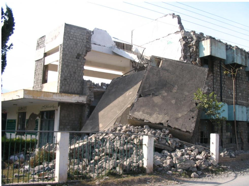
**Figure 3.40: Collapsed sections of the concrete block URM, 2-storey school building. Roof and floor slab collapse due to failure of masonry bearing walls, Muzaffarabad**
