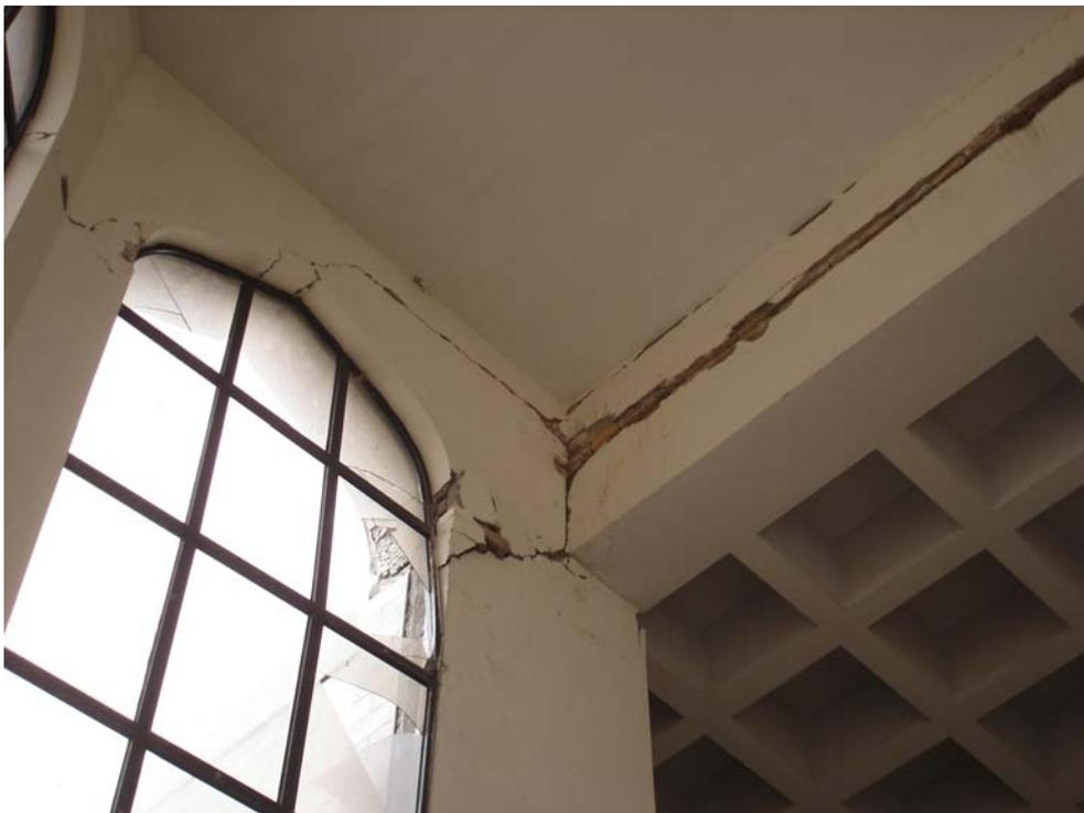
**Figure 3.36: Shear cracks through the brick masonry column and roof beam connection at the Muzaffarabad Supreme Court building. Damaged glass due to shearing through the window**
