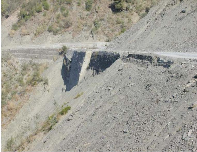
**Figure 4.33: Road network and topography: reactivated landslide blocked this road for about 24 hours and has started to undercut the abutment. View from the same position as Figure 4.32**
