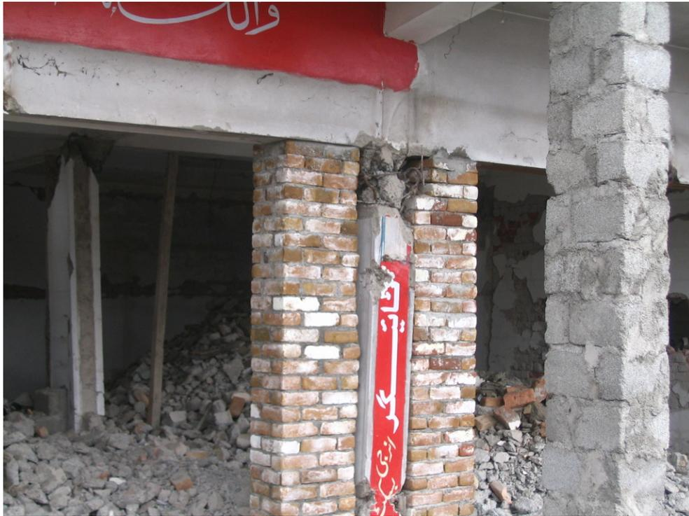
**Figure 3.46: Extensively damaged 3-storey RC commercial building. Failed beam/column connections due to lack of shear or confinement reinforcement and inadequate layout, collapsed and cracked brick masonry infill walls inside the building, Abbottabad**
