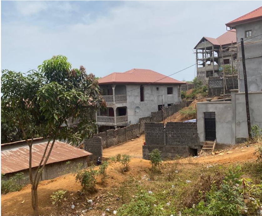
Figure 5: A house under construction in the neighbourhood
