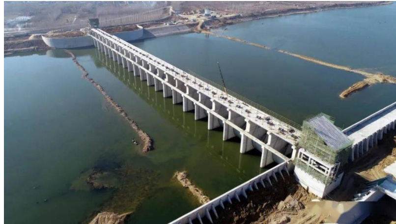
Figure 6.2. The storage dam of Matou irrigation district.
