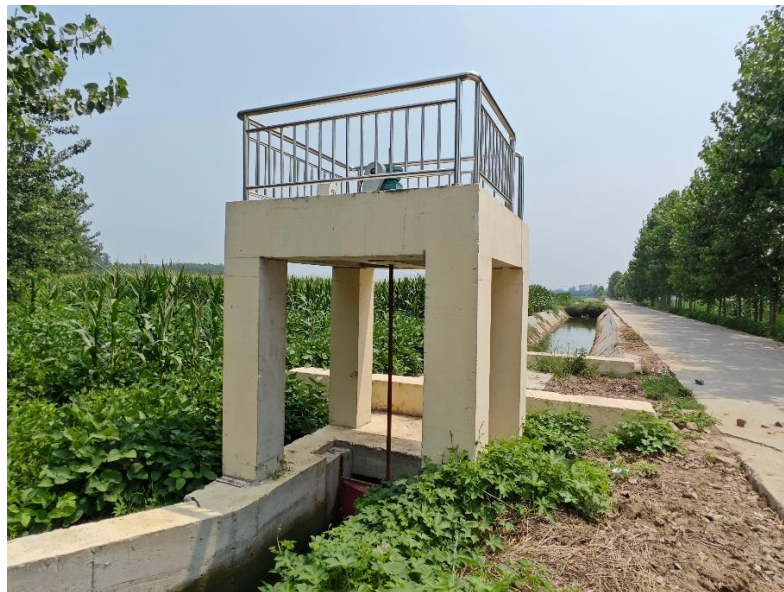
(b) The distribution gate in the branch canal.
