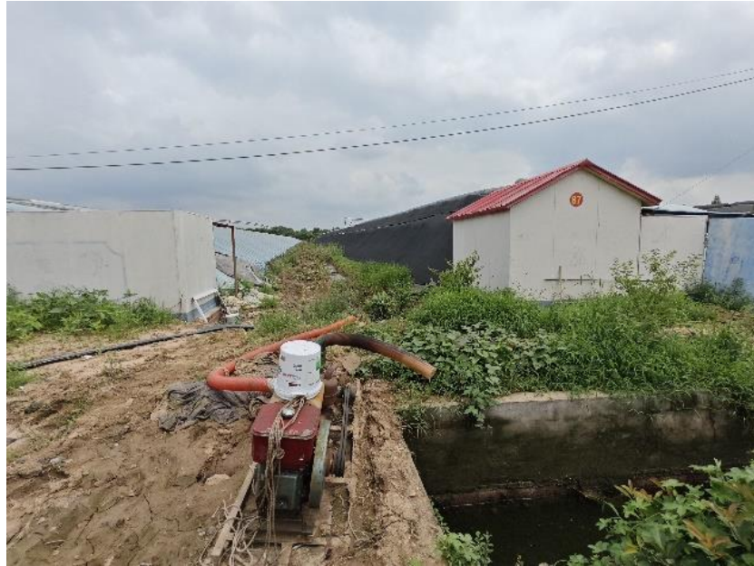
Figure 7.10. The diesel engine used to pump water off the greenhouse.
