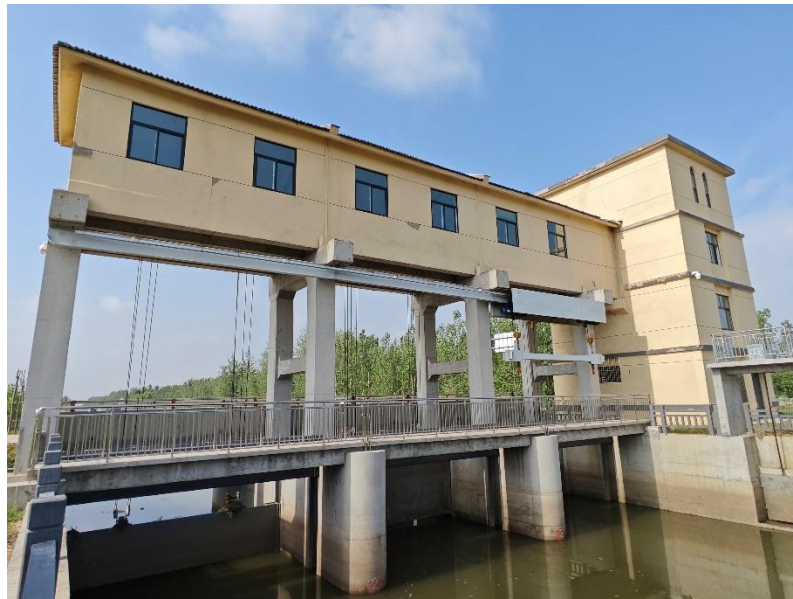
(a) The regulation gate in the main canal.
