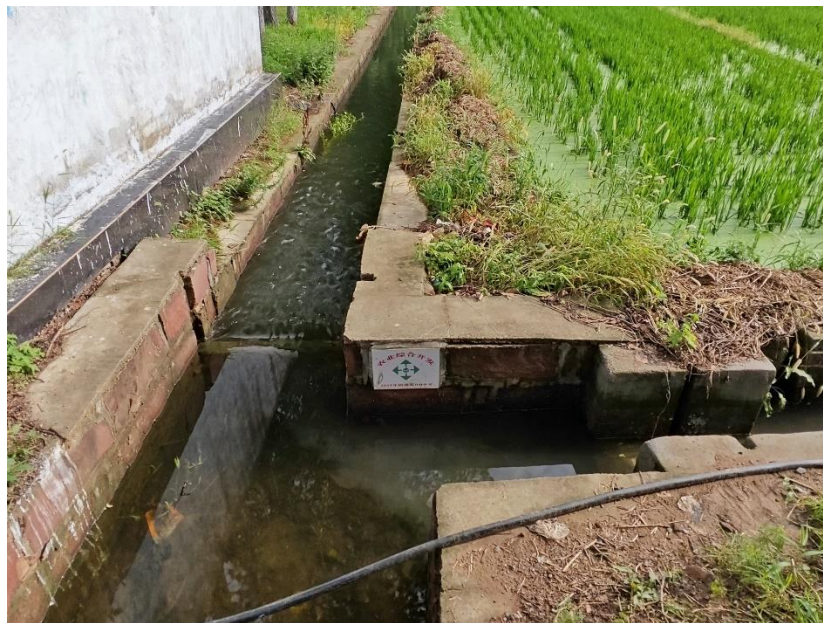
(b) The lined canal branch.
