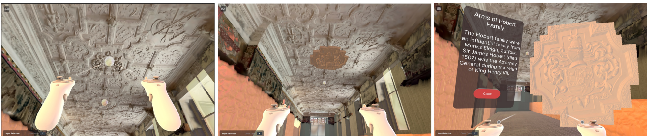
Figure 1: Our Level-of-Detail (LOD) framework enables efficient digitization of high heritage ceilings, demonstrated through the 4.8-meter-high historical ceiling (37.5m length) at the National Trust’s Blickling Hall, United Kingdom. Our approach combines 3D Gaussian Splatting (3DGS) [KKLD23] reconstruction with high-resolution 3D scanings of intricate emblematic patterns, creating a hybrid visualization system in Virtual Reality (VR). The VR environment enables seamless transitions between architectural-scale visualization and immersive inspection of fine details, enhanced by integrated narrative storytelling.
