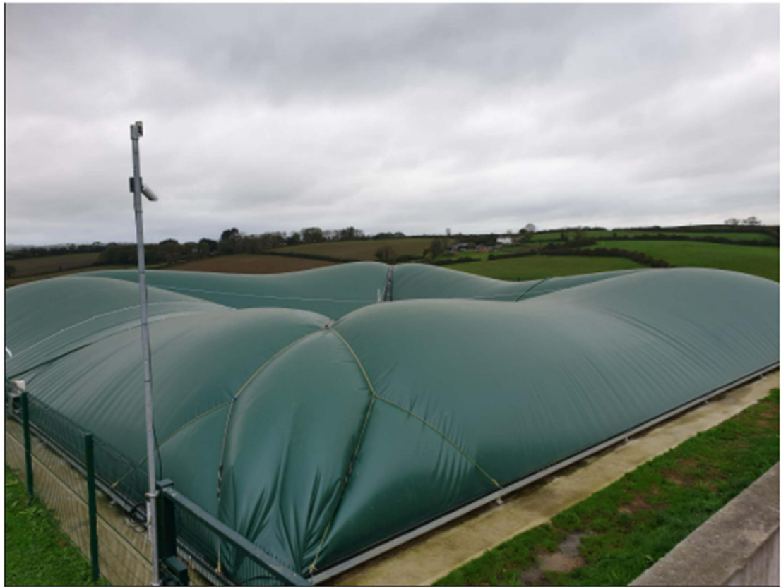
Figure 3. A Slurry Storage Facility with an Air-Tight Cover to Capture Methane Emissions.
