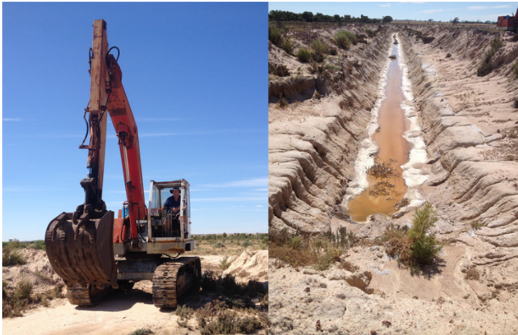
Figure 2.7.7: Salt drainage trench excavation in action.
