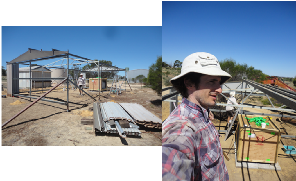
Figure 2.7.5: The first task was to build suitable shelter for the IRES.
