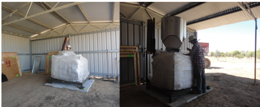
Figure 2.7.6: Commissioning the IRES in its new home.
