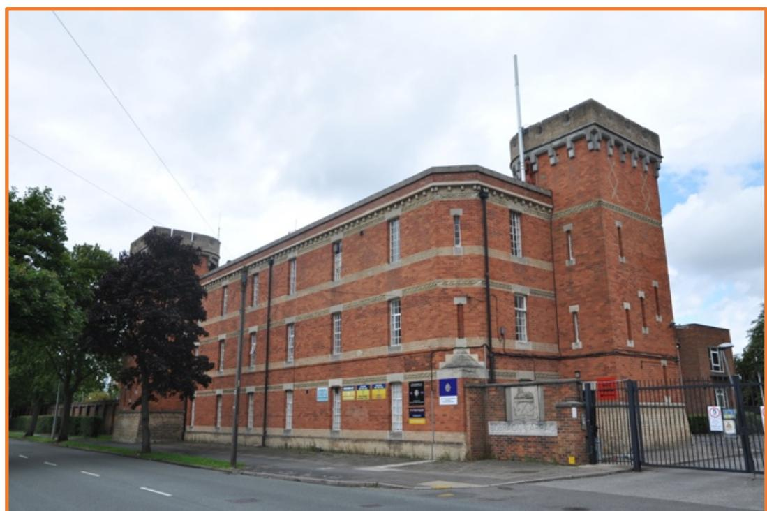
These three of the newly built Cardwell barracks in the East from the 1870s provide very clear examples of the dominant keep as integral to the designs produced by Major Seddon. They usually had concrete floors supported on iron columns, with a powder
