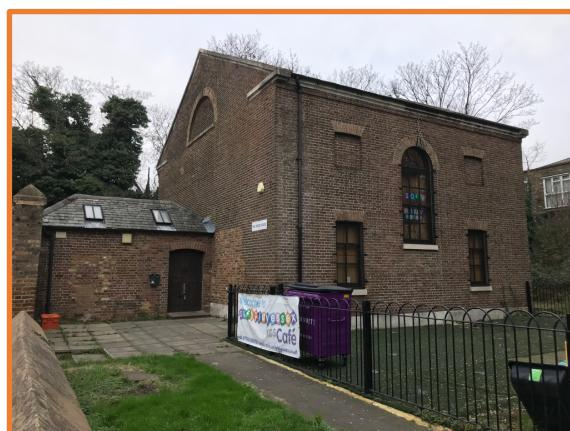
The five magazine buildings had a capacity of 52,000 barrels, each magazine could hold 10,400 barrels (460 tons) of gunpowder. The most significant monument to its past military use is the No. 5 Powder Magazine building which remains largely as originally built. It is divided as a pair of long brick barrel-vaulted aisles, each 19ft wide and 17ft from floor to head of vault. At the east and west ends groined cross vaults
