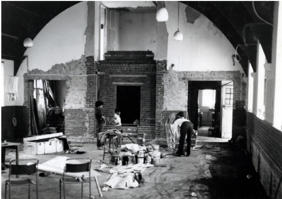
Figure 17: Shree Ghanapathy Temple in construction, image from their website. Online: https://ghanapathy.co.uk/history/ . [accessed: 22/04/2023].
