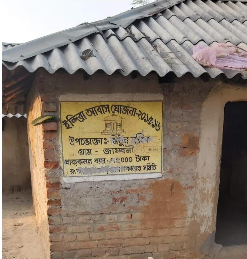
A Lodha house built under state welfare scheme, without doors or windows.
