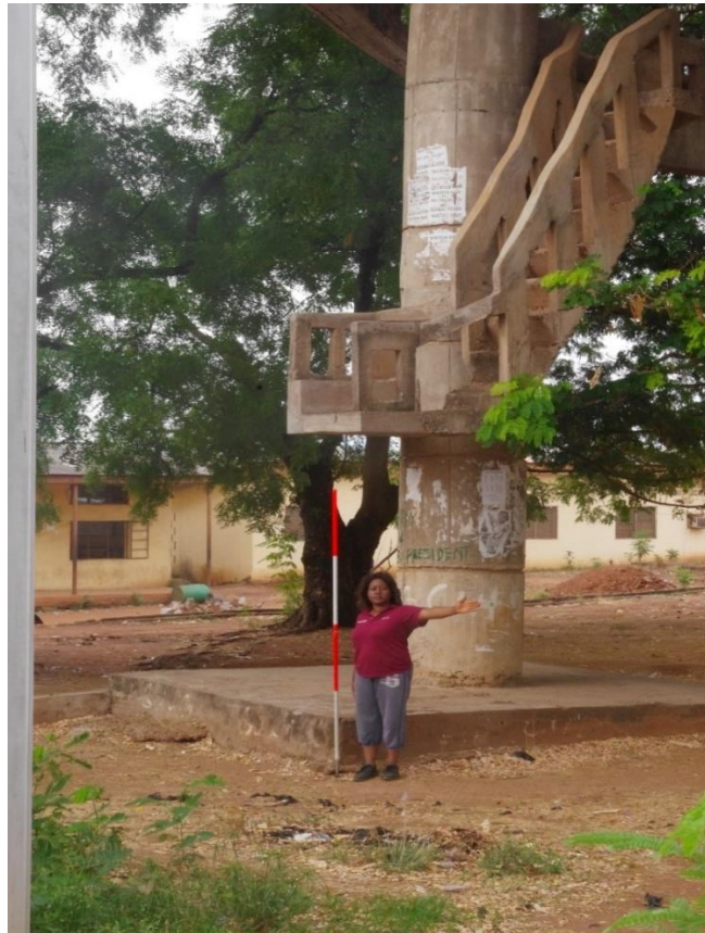
Figure 3.19. The researcher during the surveys of a concrete water reservoir at Kwara State College of Education grounds Ilorin (see Figures 3.3 & 3.4 and Table 3.3 for concrete water reservoir location and coordinates) (Photo: Emmanuel Adeara 2020).
