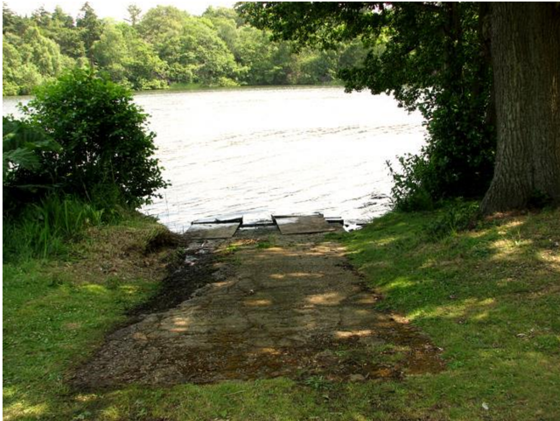
Fig.57 Slipway at Fritton Lake; rare remaining surface structure 112
