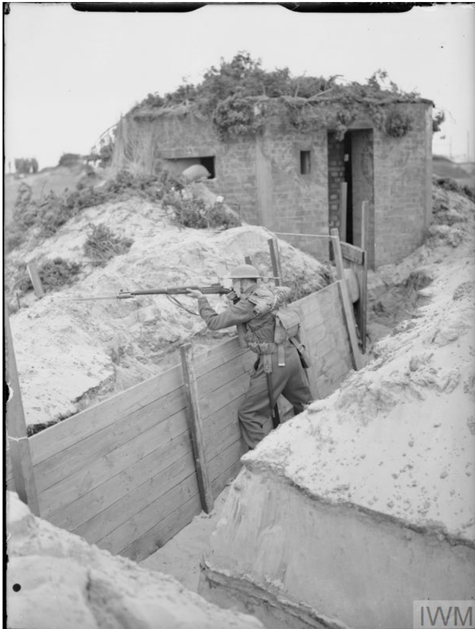
Fig.13 The trench systems connecting pillboxes in the front line of defence. ‘A soldier of the 4 th Battalion, The Royal Norfolk Regiment, mans a trench near a pillbox at Great Yarmouth 31 July–2 August 1940’ 86
