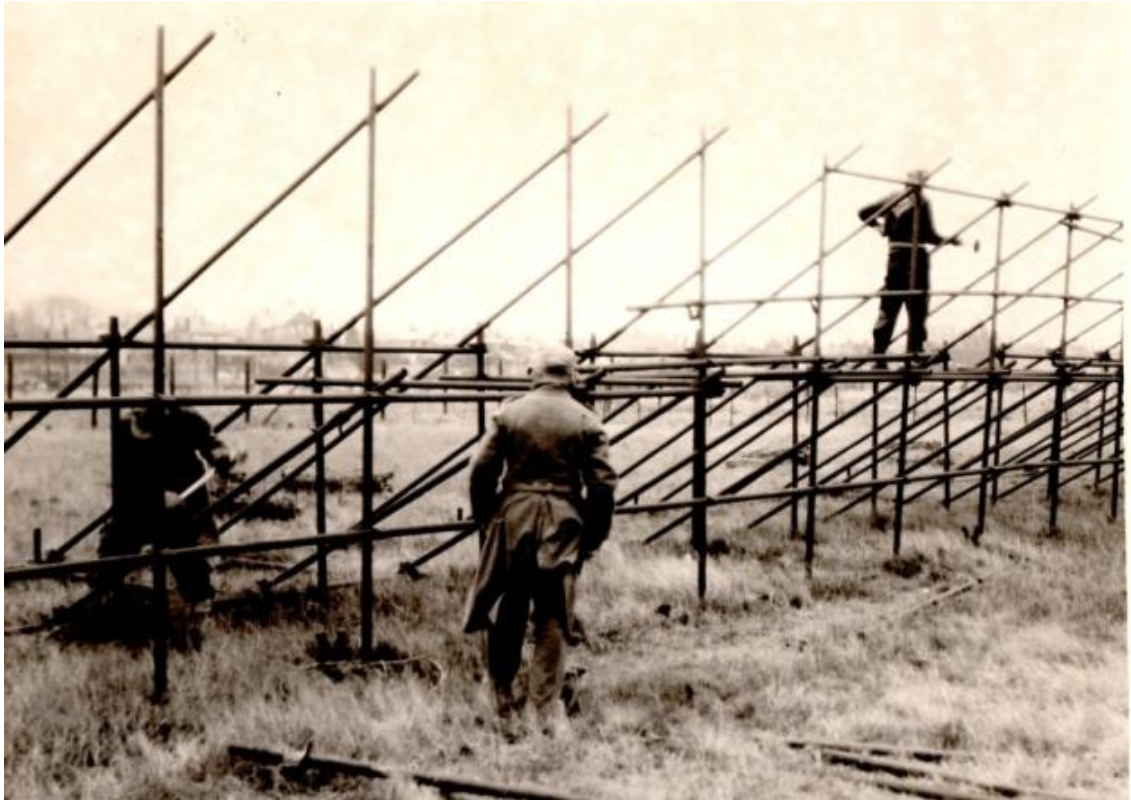
Fig.27 German Prisoners of PoWs removing beach scaffolding on the North Denes, Great Yarmouth, 1946. 161
