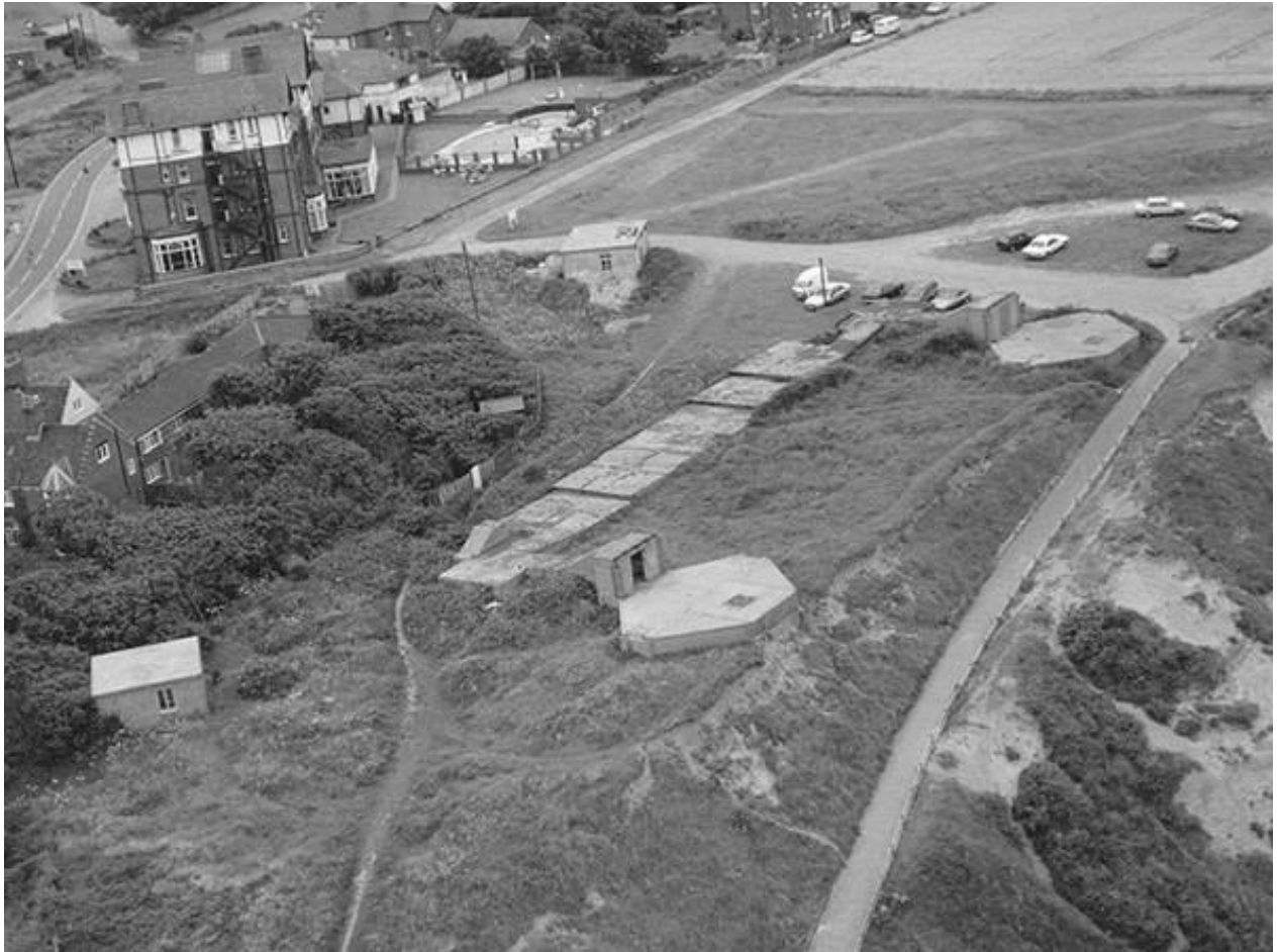
Fig.9 Oblique aerial perspective of Mundesley Emergency Coastal Defence Battery. 66
