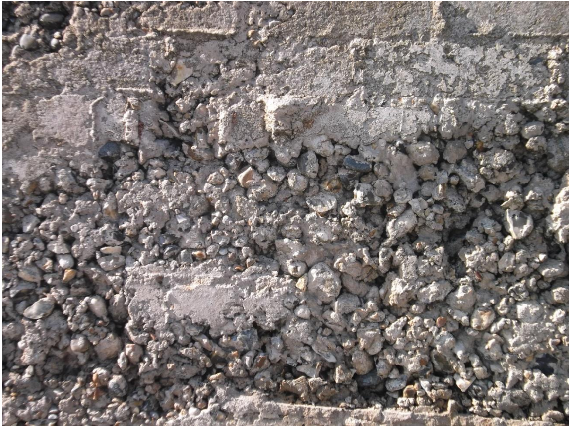
Fig.17 Close view of exposed wall section of pillbox on Weybourne beach, showing quantity of local beach stone used as aggregate. (Author's photo)
