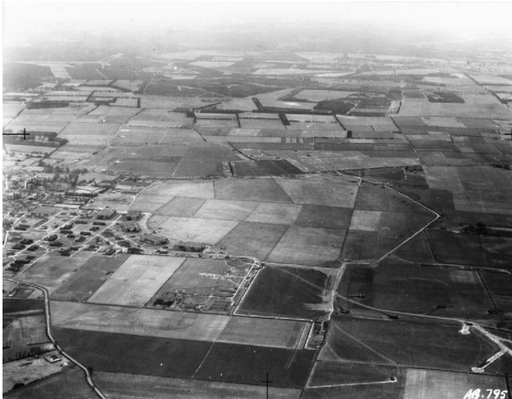
Fig. 33 Oblique aerial view of Feltwell, Norfolk, from the west. The flying field extends south from the clustered buildings. The airfield has been skilfully camouflaged with a field pattern. 35
