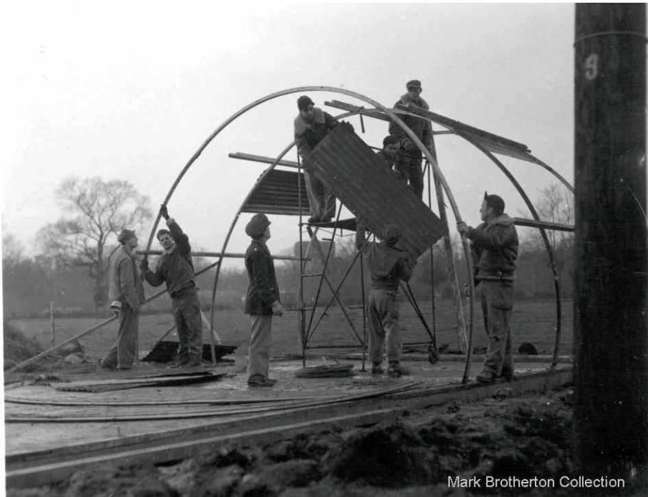
Fig.48 Buildings construction in progress at Thorpe Abbots 124
