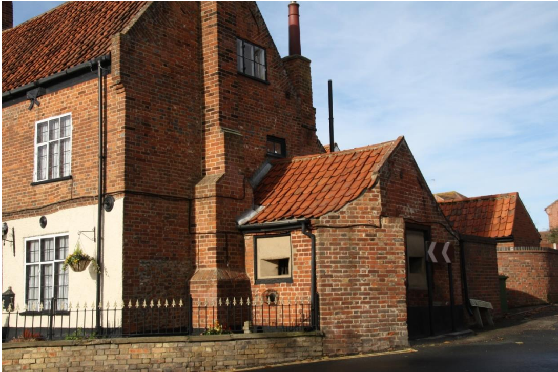
Fig.14 Acle, mid-way between Norwich and Gt Yarmouth, was a Category 'A' Nodal point. Concealed pillbox incorporated into flank wall of The Manor House, covering central road junction (author's photo).
