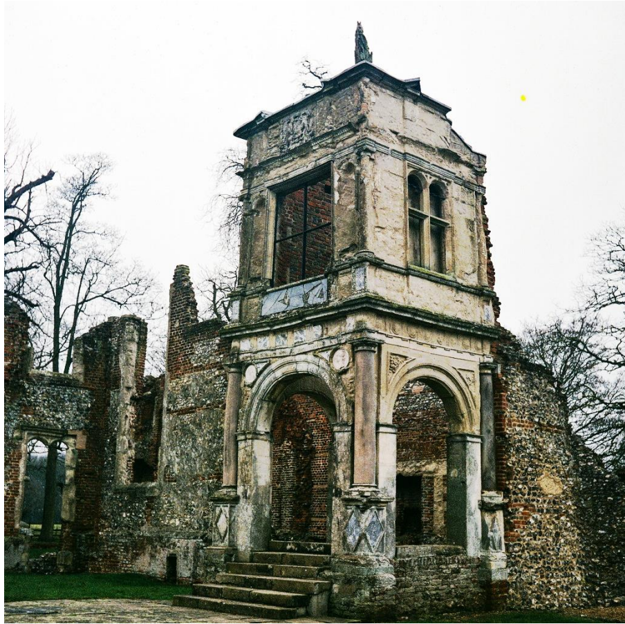
Fig. 4.11 - Entrance porch, Old Gorhambury House
