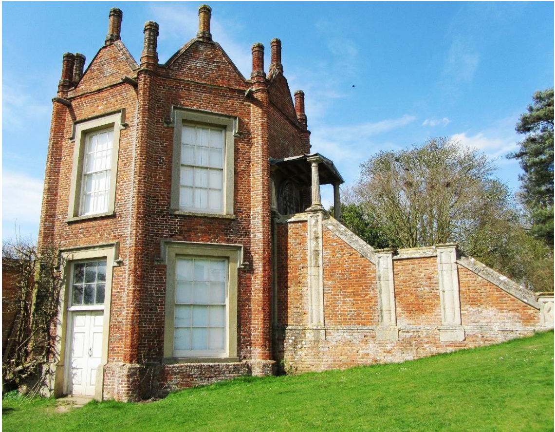
Fig. 6.44 - Banqueting House, Melford Hall
