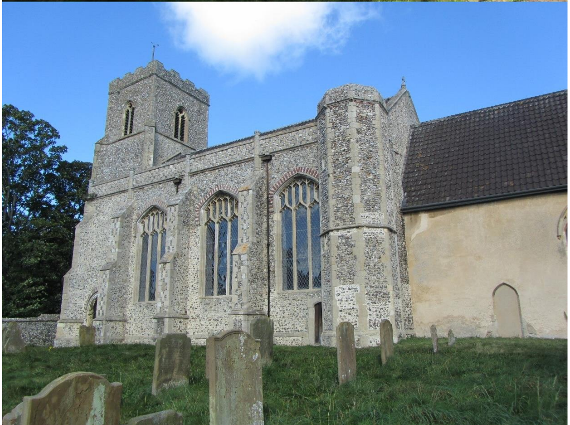
Fig. 3.19 - Photographic observations of landscape context at Stiffkey Old Hall (top) and parish church (bottom)
