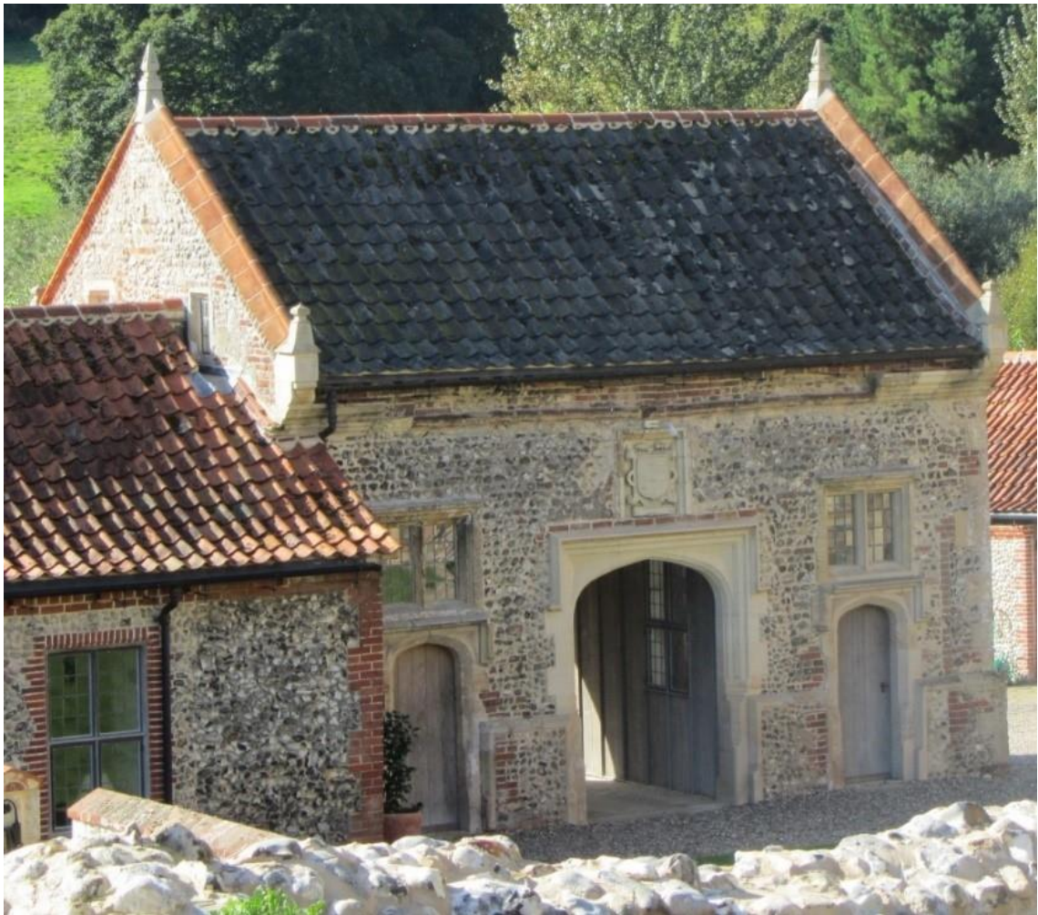
Fig. 3.27 - Photographic observation of Gatehouse, Stiffkey Old Hall
