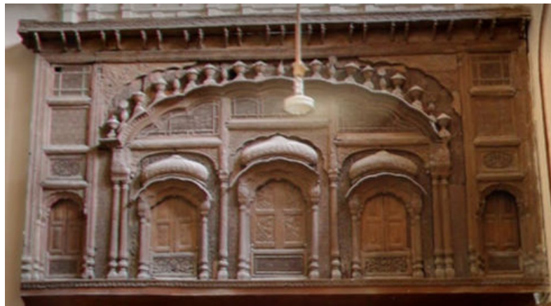
FIGURE 6.2: Facade of the Lal Nath temple in the General Gallery, Lahore Museum. Author's photograph, 2016.
