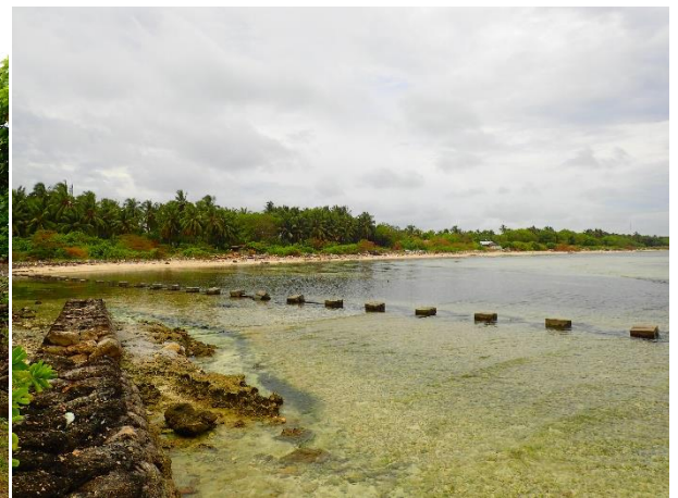
Fig 7: Concrete sandbag structure to reduce wave erosion (Photo by Annalisa Christie, February 2017)
