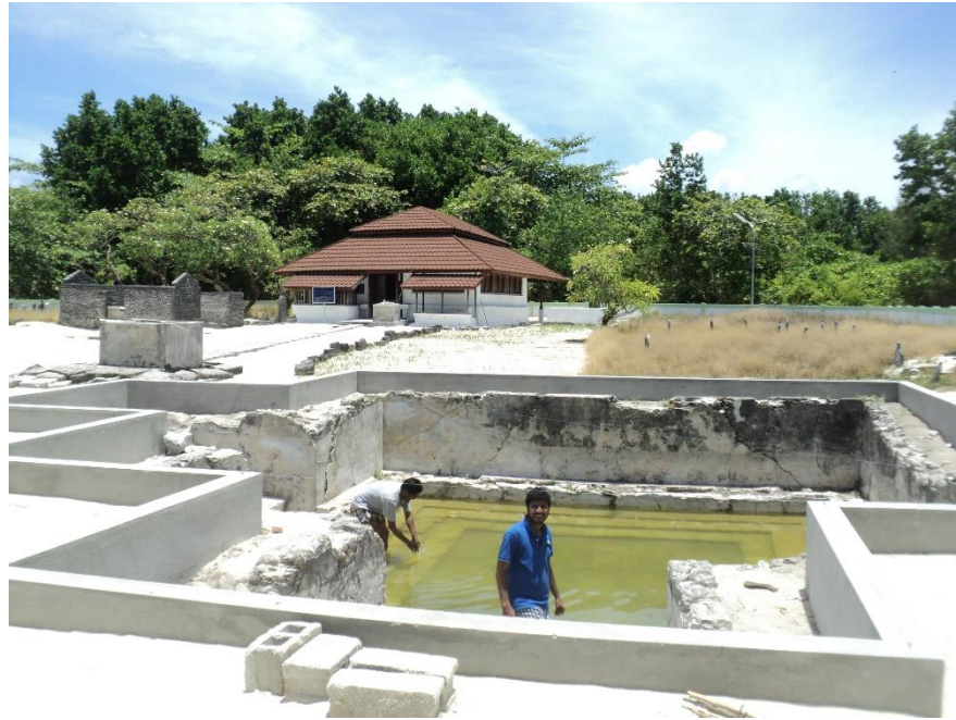
Fig 28: Excavation of bathing tank in Ha. Utheemu with the ancient Kan'dhuvalu mosque and the cemetery behind the tank (Source: Shiura Jaufar 2012)
