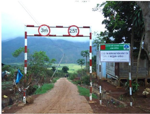
Figure 8. The concrete road sponsored by the FLITCH project in Kala Tongu
