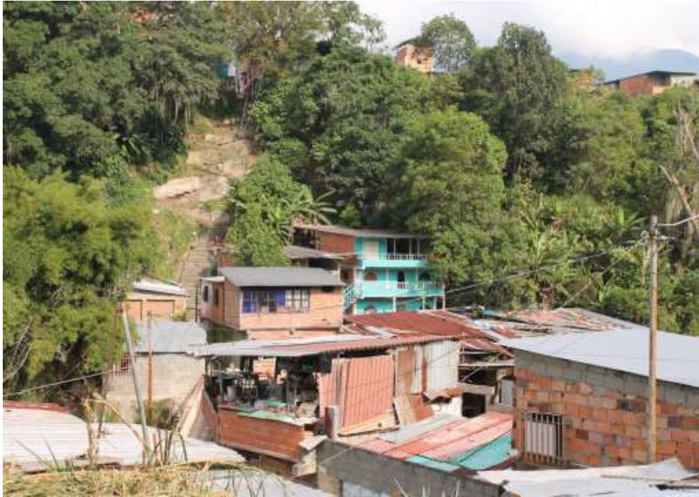
Photo 1. In Pueblo Nuevo and Simon Bolivar, homes have different building standards. June 2014
