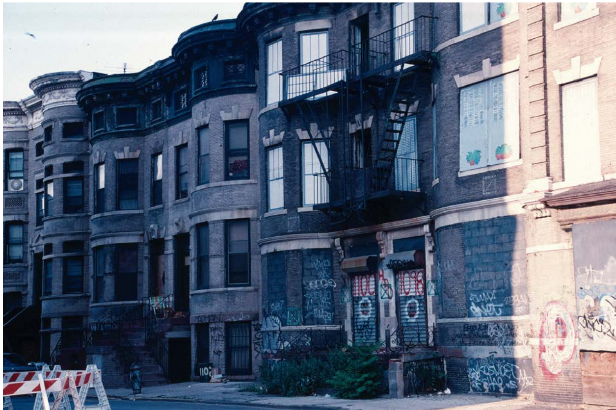
Figure 7. Building in the South Bronx with vinyl decals. Source: Photo taken by the author in 1997.
