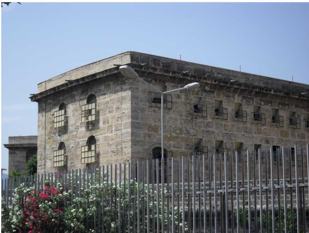
Picture 2: The panels covering the windows were originally built to prevent inmates from having any view of the outside. Panels for the same purpose can be seen at San Vittore (see picture 3).
