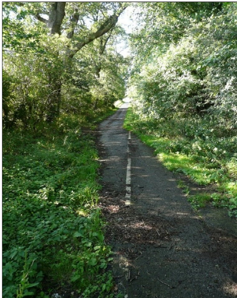
Figure 2. A section of the former A140 at Marsham in Norfolk which has been replaced by a new carriageway to its west. Its tarmac surface is rapidly becoming overgrown where it is not still being used as a footpath.
