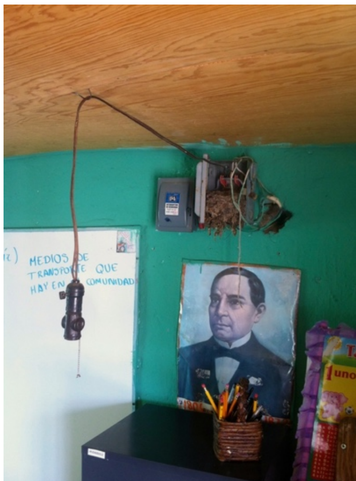
Image 11: Lack of electricity in a classroom. Pueblo Nuevo, Durango. 28 May 2013
