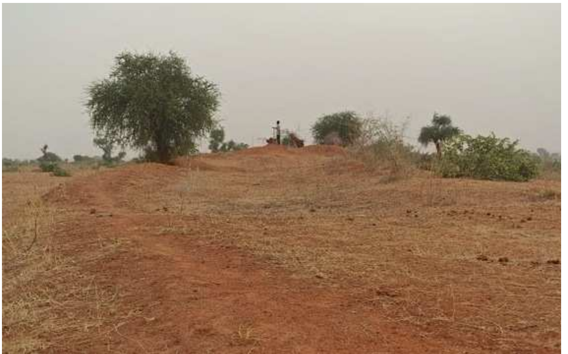
Figure 4.24: The Gandu Shira defensive wall.
