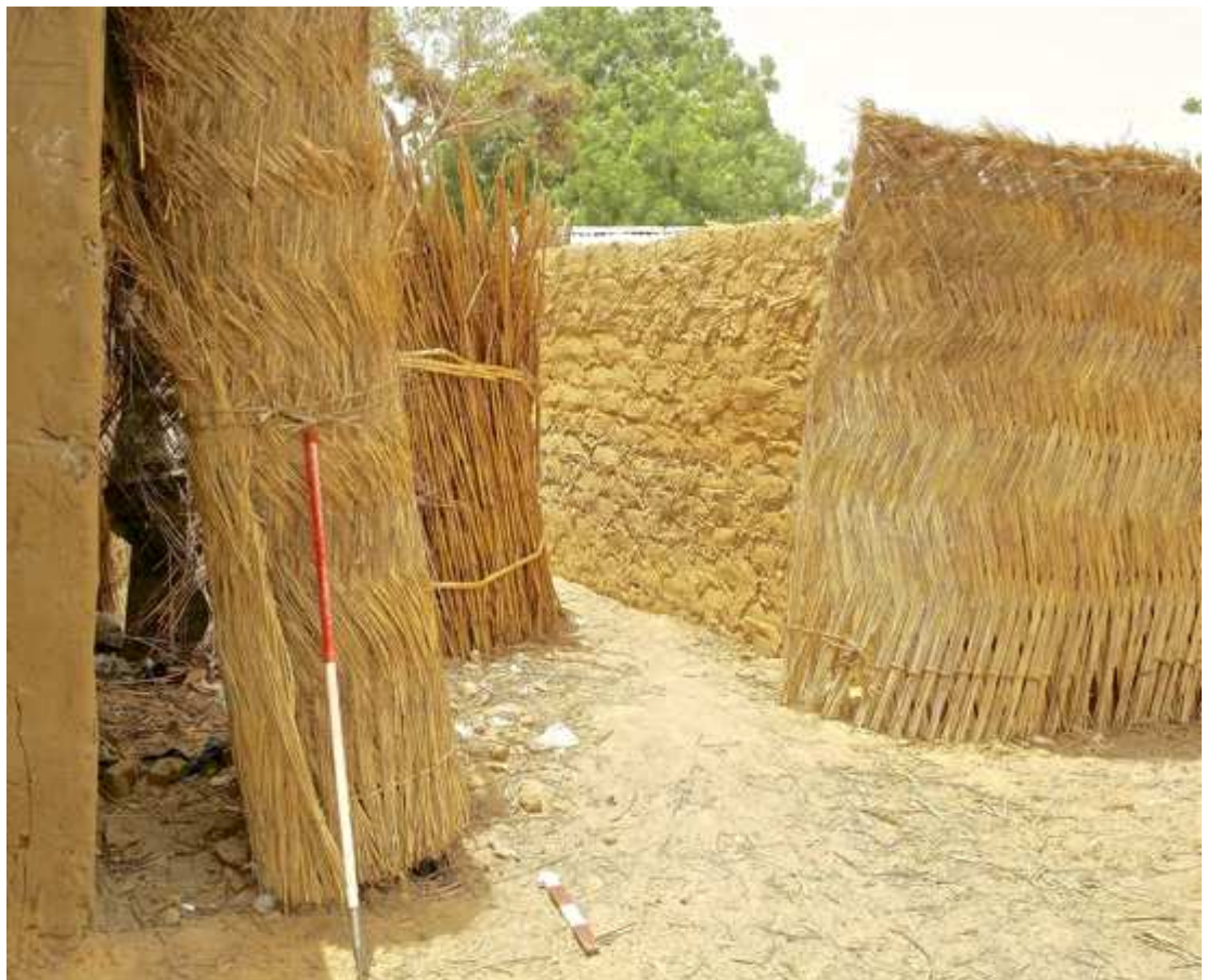
Figure 3.8: Weaving of grasses into a wall - danga (top) and the finished wall in Malori.
