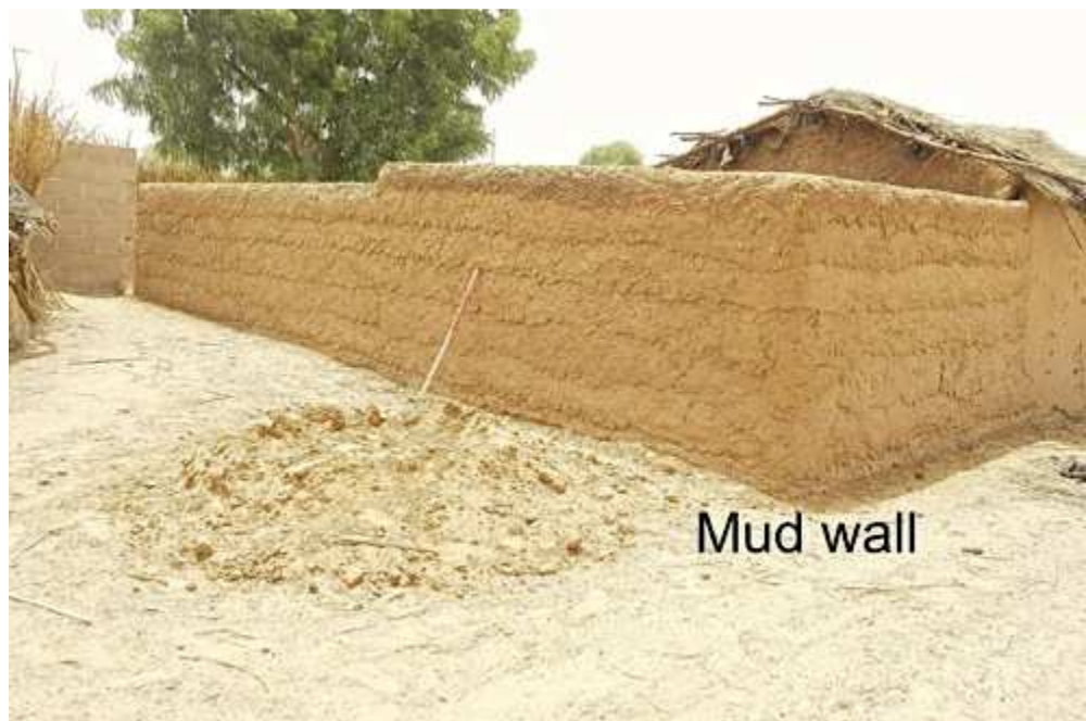
Figure 3.7: The different types of fencing houses and materials (grass and mud) used in Shira.
