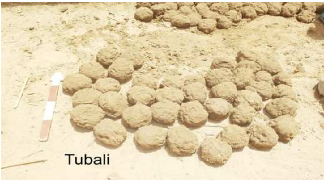
Figure 3.9: Mixing mud for tubali building in Faggo and Malori, Shira.
