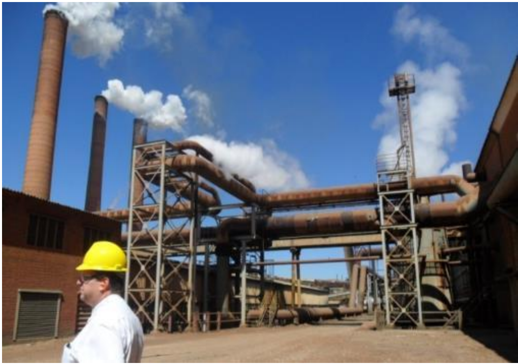
Figure 6: USJ's sugarcane processing plant (Source: author).
