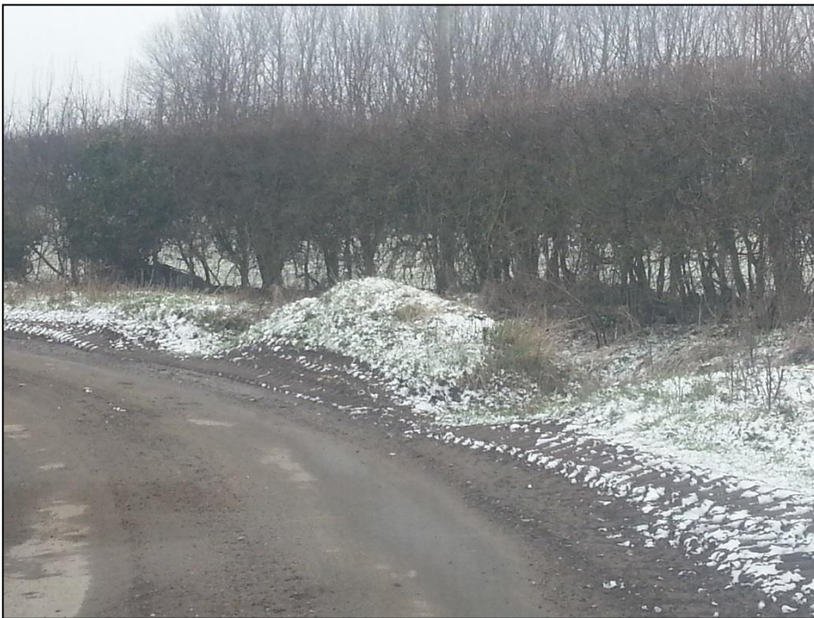
Fig. 5.11 Erosion of verge grips due to heavy machinery, only the fact that the ground was frozen prevented additional silt being washed into the ditch on the other side of the hedge
