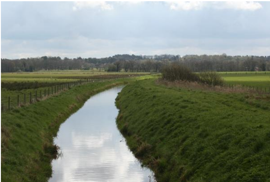
Fig. 3.8 A canalised section of the Gaywood chalk river showing the raised banks and disconnection from the floodplain. Here the water is deep with little natural plant life and a layer of silt covers the gravel bottom; precipitation results in quickly raised river levels increasing flood risk downstream.
