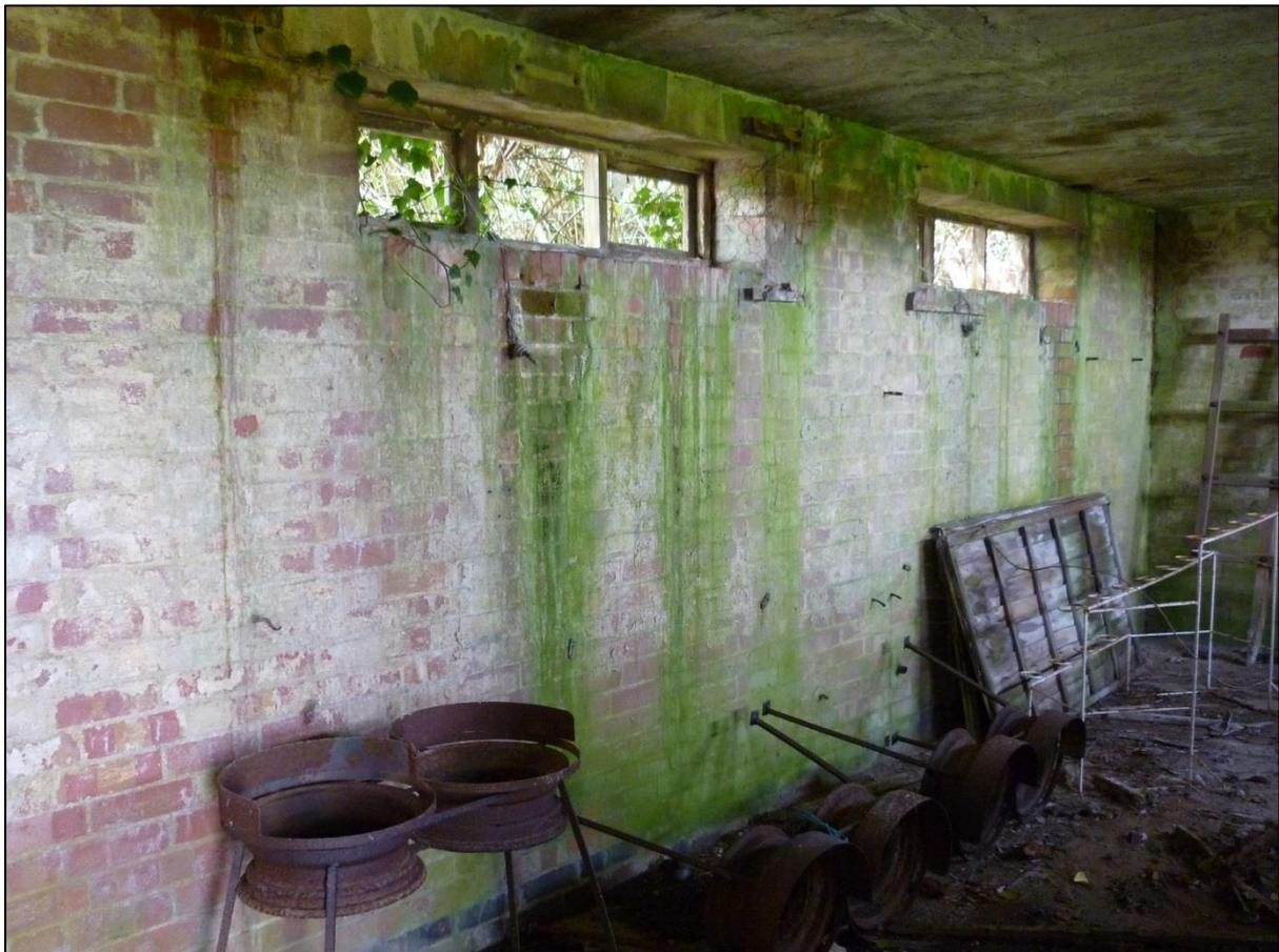
*Figure 10: Photograph taken looking south-west towards the southern elevation of Room 5 within the Generator Building. The in situ wooden window frames are clearly visible (Gregory 2013).*
