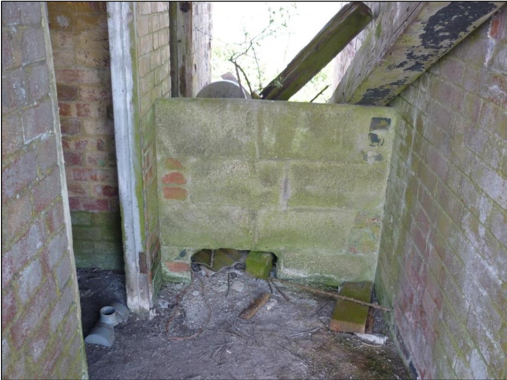
*Figure 28: Photograph of the breeze block half-wall in Room 1 of the Generator Building (Gregory 2013).*
