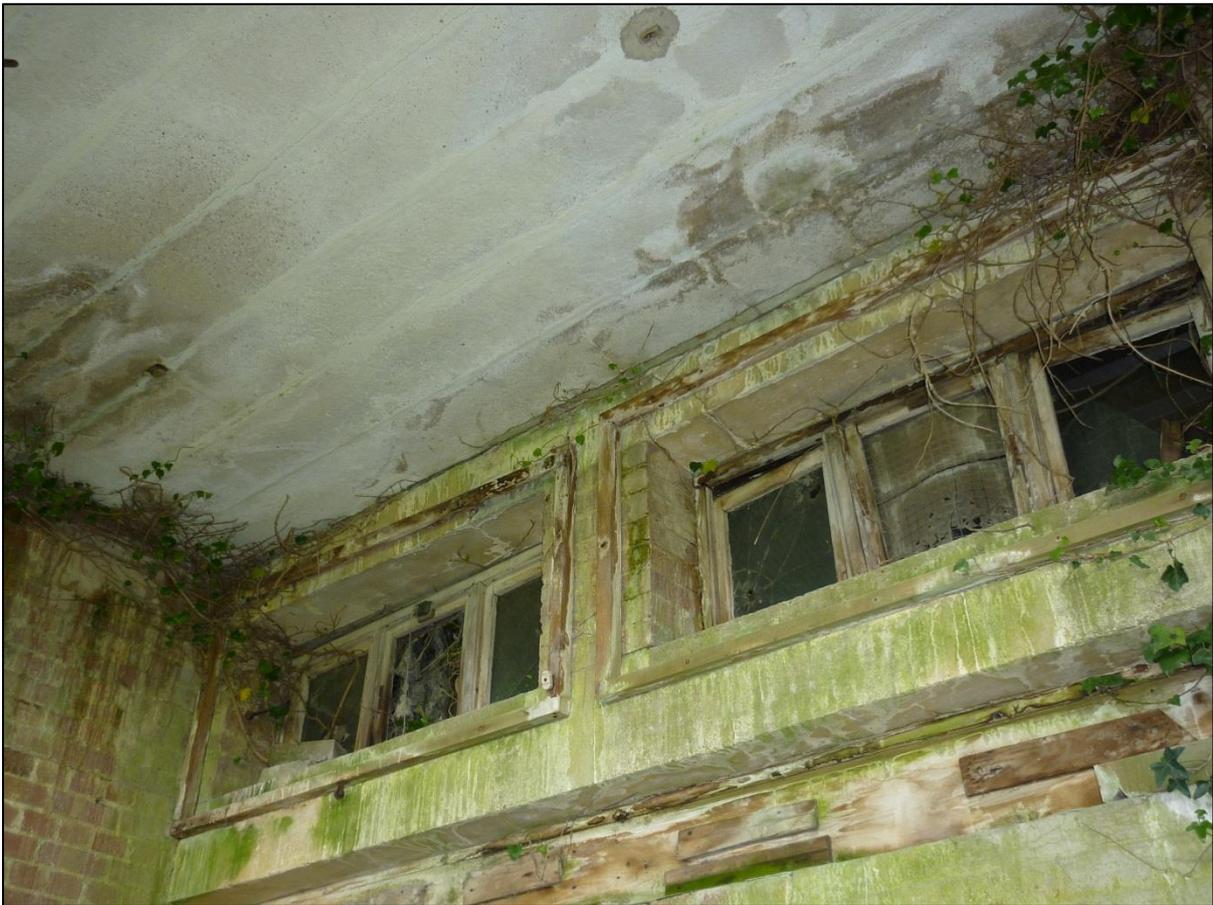
*Figure 23: Photograph of in situ window frames in Room 4 of the Transmitter Building. Wire-meshed glass panes are visible within the windows. The method of opening the windows via a series of pulleys can be observed in this photograph (Gregory 2013).*
