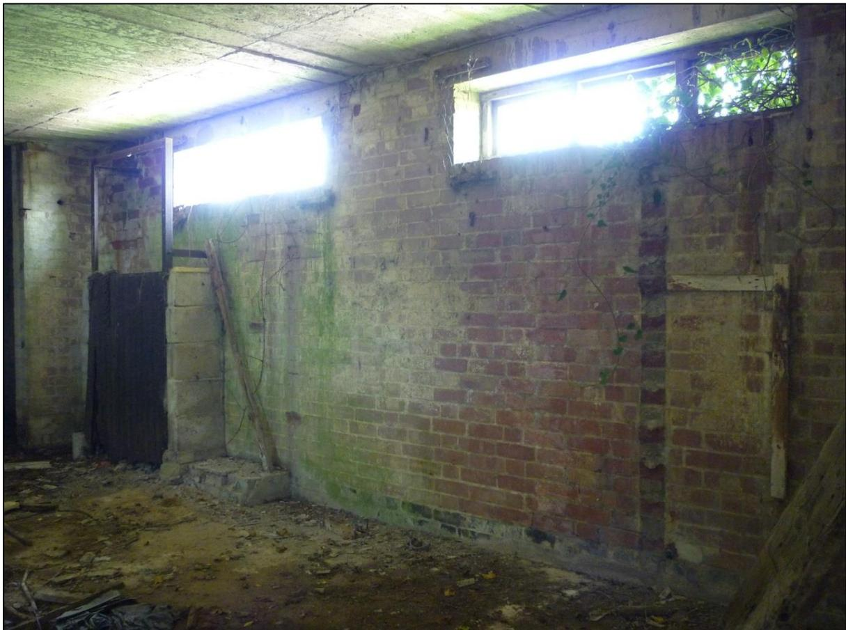
*Figure 11: Photograph taken looking north-west of the northern elevation of Room 5 of the Generator Building. The brick footing for a piece of equipment is clearly visible to the left of the photograph (Gregory 2013).*
