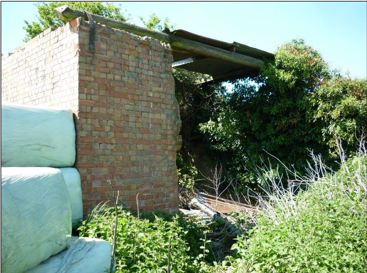
*Figure 14: Photograph taken looking north-west towards the entrance to Room 7 of the Generator Building. The 'English' bond brickwork is clearly visible. At a later date, the southern section of the eastern elevation was partially demolished. There is no evidence that the room was originally roofed (Gregory 2013).*
