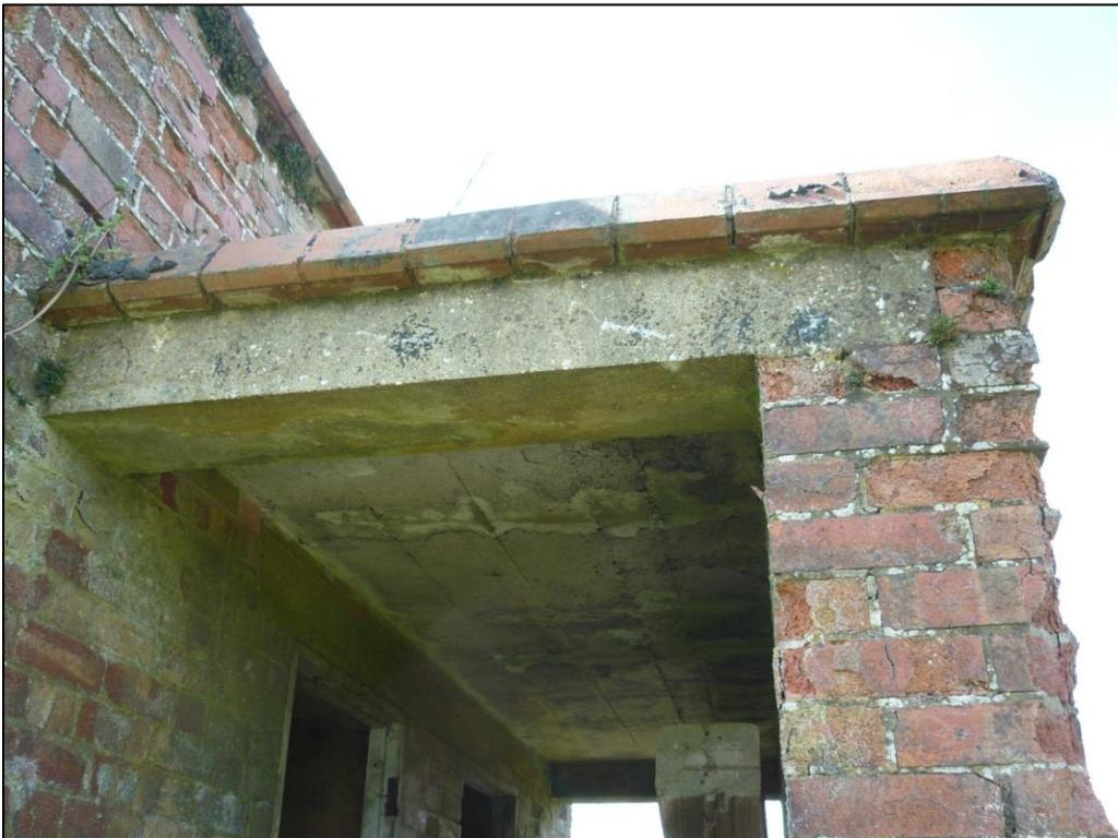
*Figure 27: Supporting beam across the northern entrance to Room 1 of the Generator Building (Gregory 2013).*
