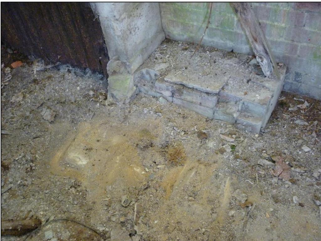
*Figure 31: Brick footing attached to the western section of the northern elevation in Room 4 of the Generator Building (Gregory 2013).*
