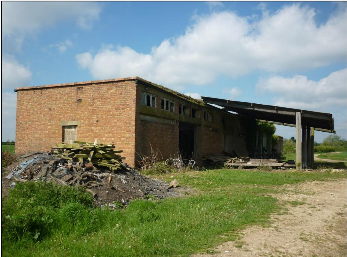
*Figure 16: The Transmitter Building from the north-east. To the right of the picture, the later addition of a lean-to is clearly visible. It is believed that the wooden posts once formed the antennae of SOE's Station 53B transmitter complex. The blocked up doorway into Room5 is visible on the eastern elevation of the building (Gregory 2013).*
